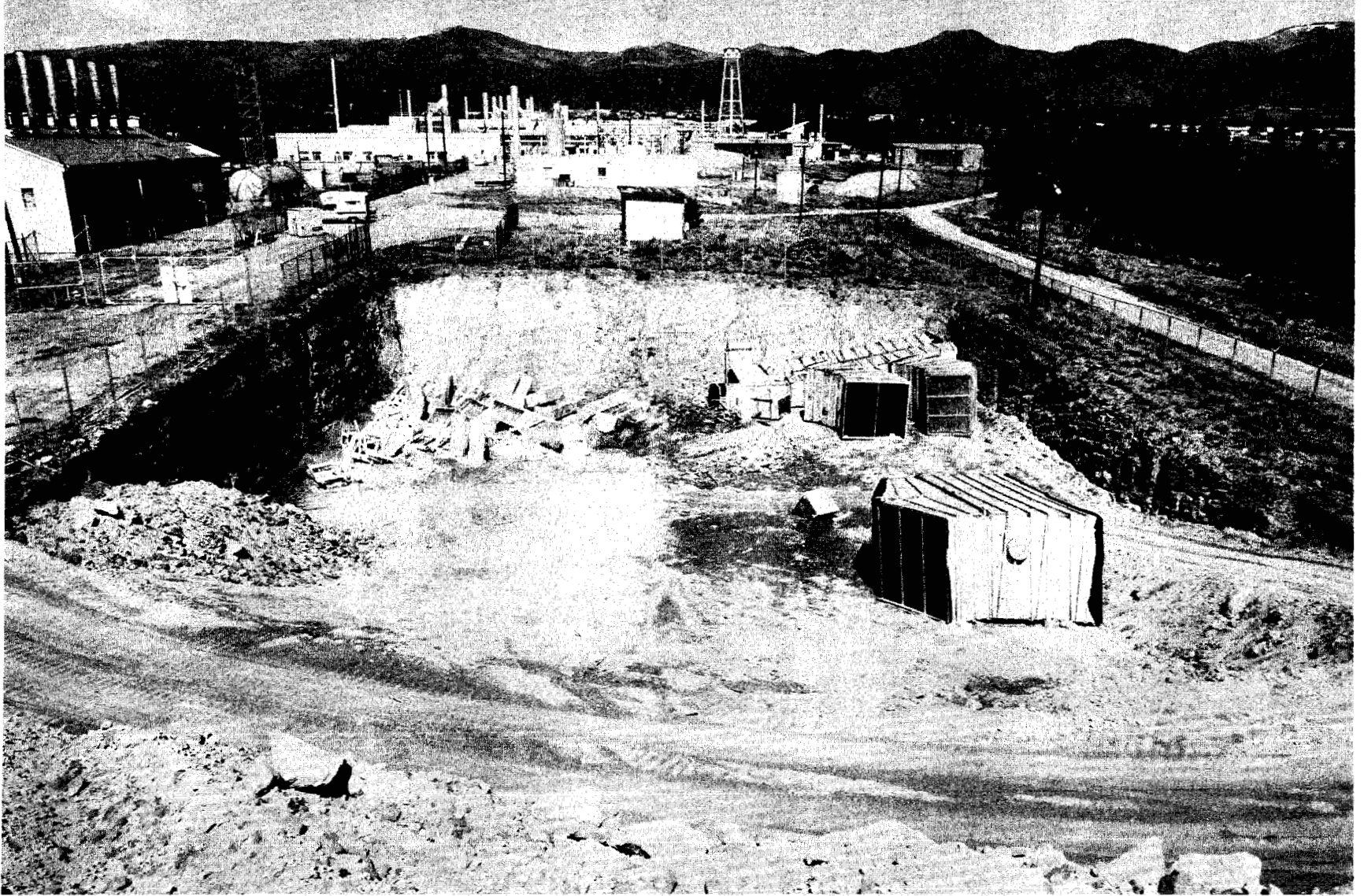
Fig. 12. Photograph (1973) showing burial of building demolition materials in the disposal pit.
