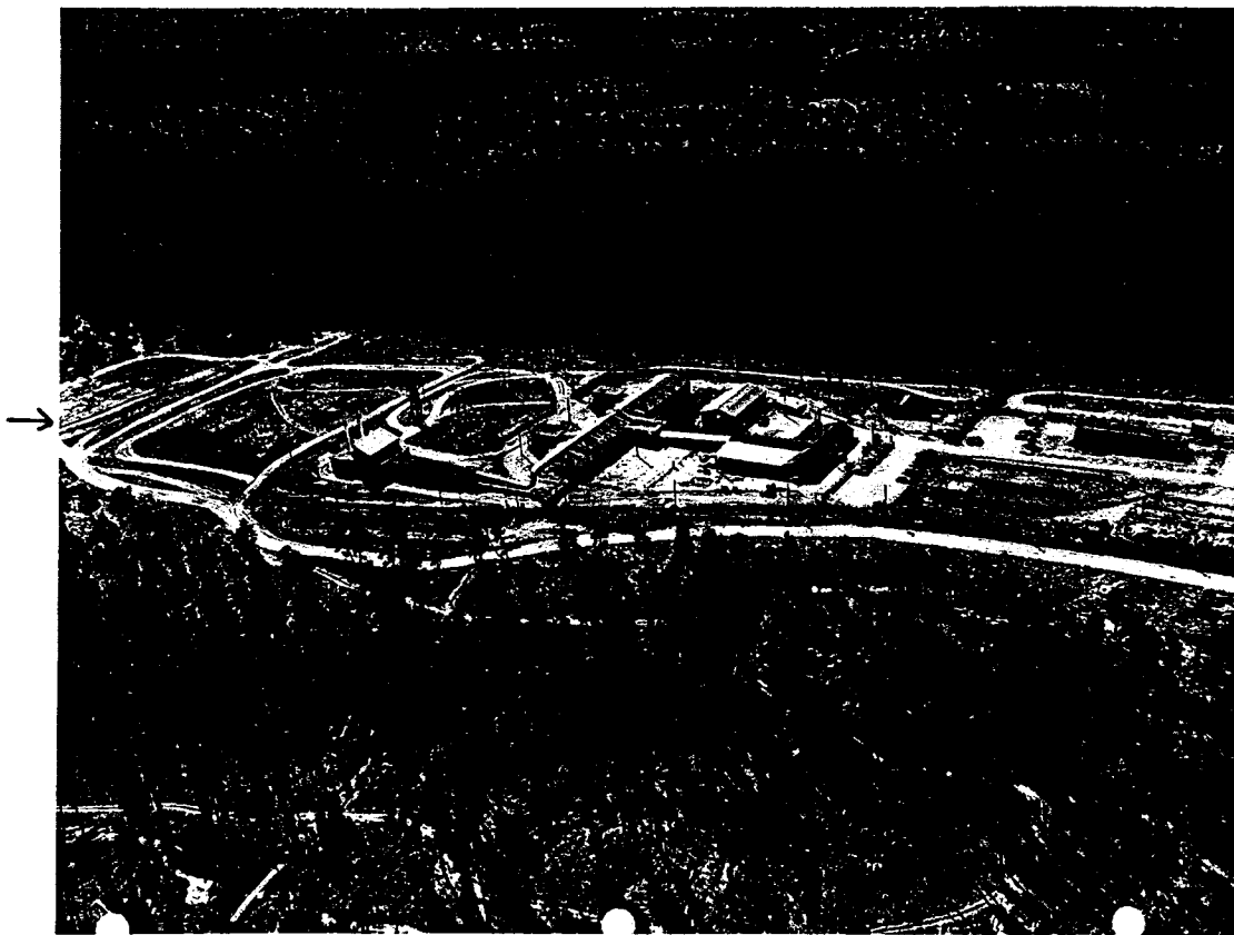
Photograph 5 View Looking South at the East End of TA-21, (ERID0019082)
