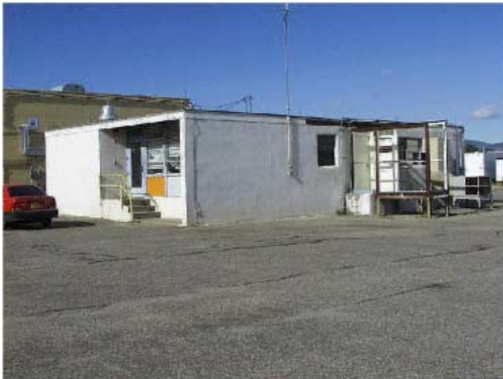
TA-21-1 South and East Elevations
