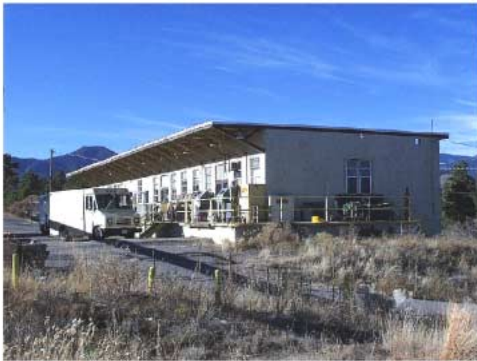
TA-21-31 South and East Elevations
