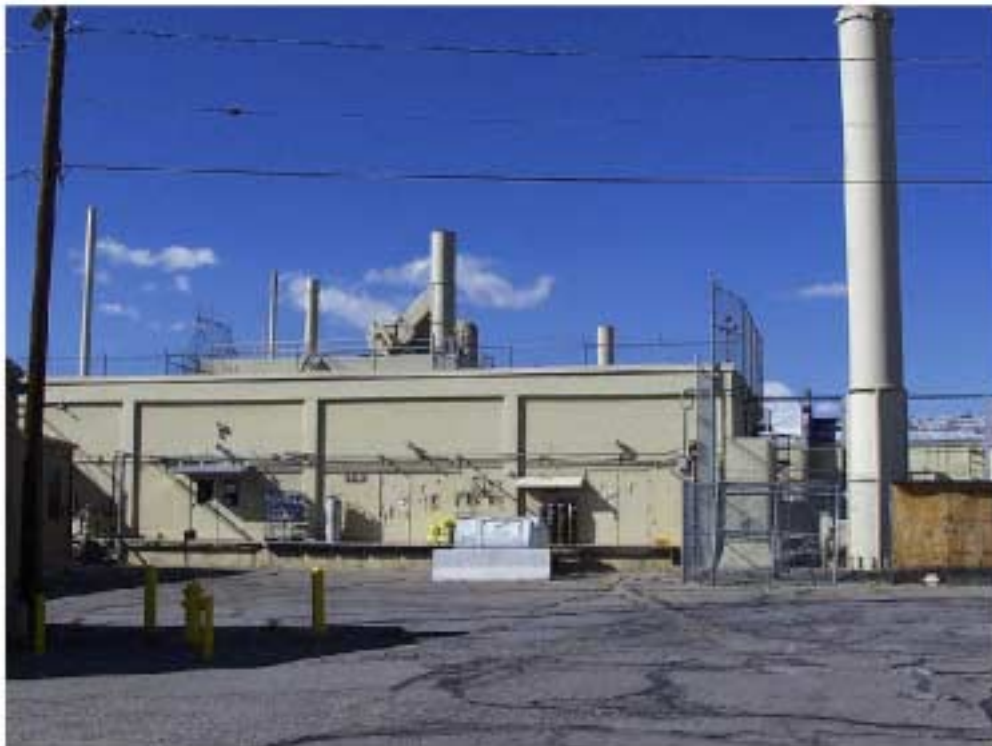
TA-21-150 East Elevation of North Wing
