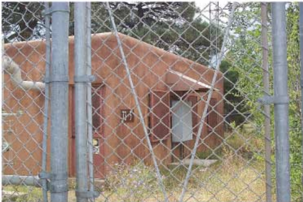
TA-73-5 East and North Elevations
