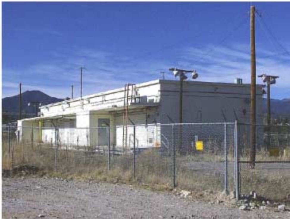
TA-21-21 South and East Elevations
