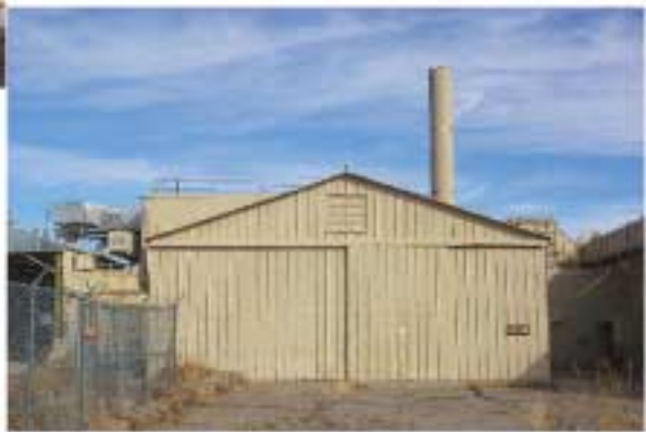
TA-21-116 South Elevation of 1957/1958 Portion
