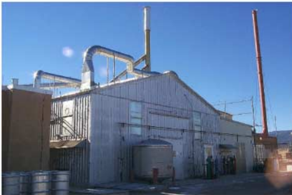
TA-21-152 East and North Elevations
