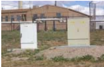
Telephone Pedestals/Cabinets
