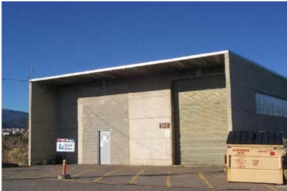
TA-73-2 South and East Elevations
