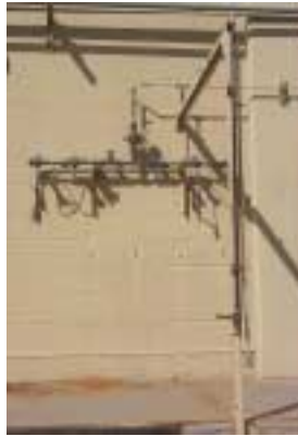
Example of small gas manifold
