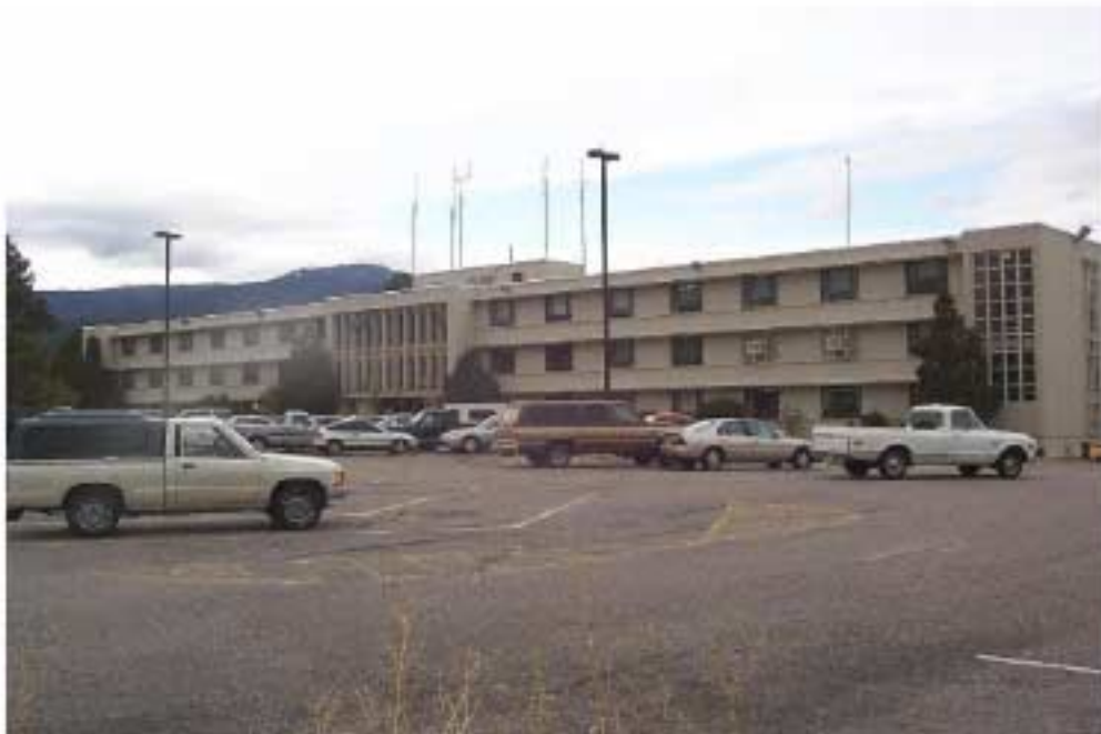
TA-43-39 South and East Elevations
