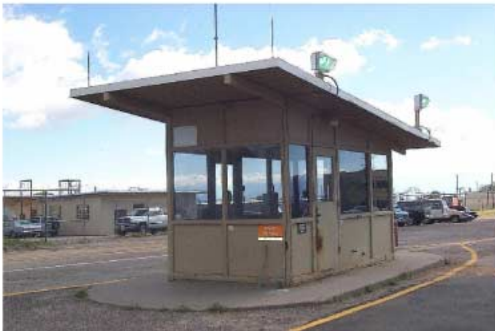
TA-21-254 West and South Elevations
