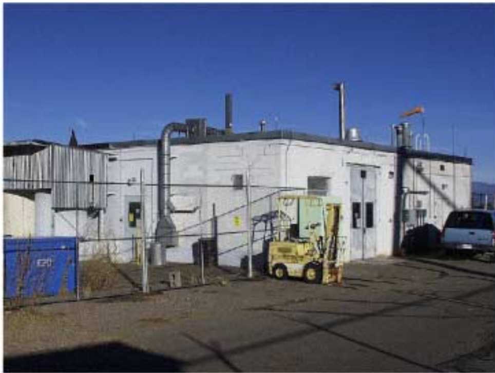
TA-21-257 West and South Elevations
