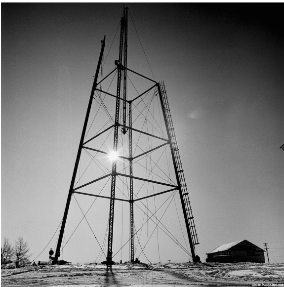
Figure 62. Dismantling the tower.
