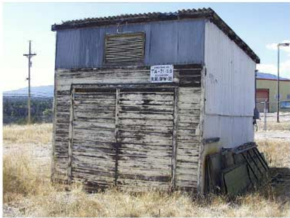
TA-21-59 East and North Elevations
