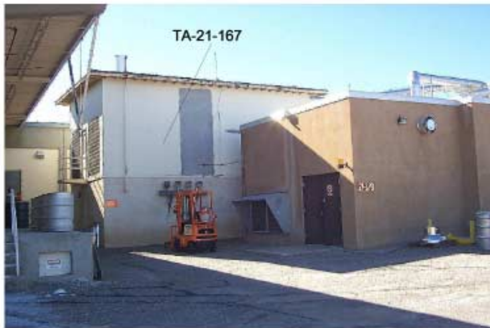
TA-21-167 East and North Elevations
