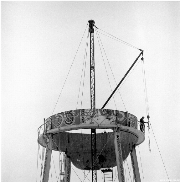
Figure 61. The dismantling of the tank, 1966.
