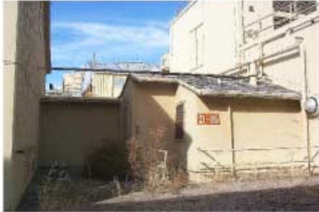
TA-21-116 South and East Elevations of 1950 Portion
