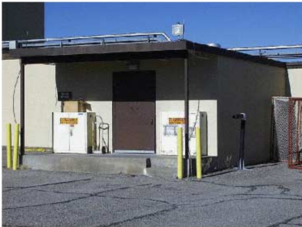
TA-21-328 South and East Elevations
