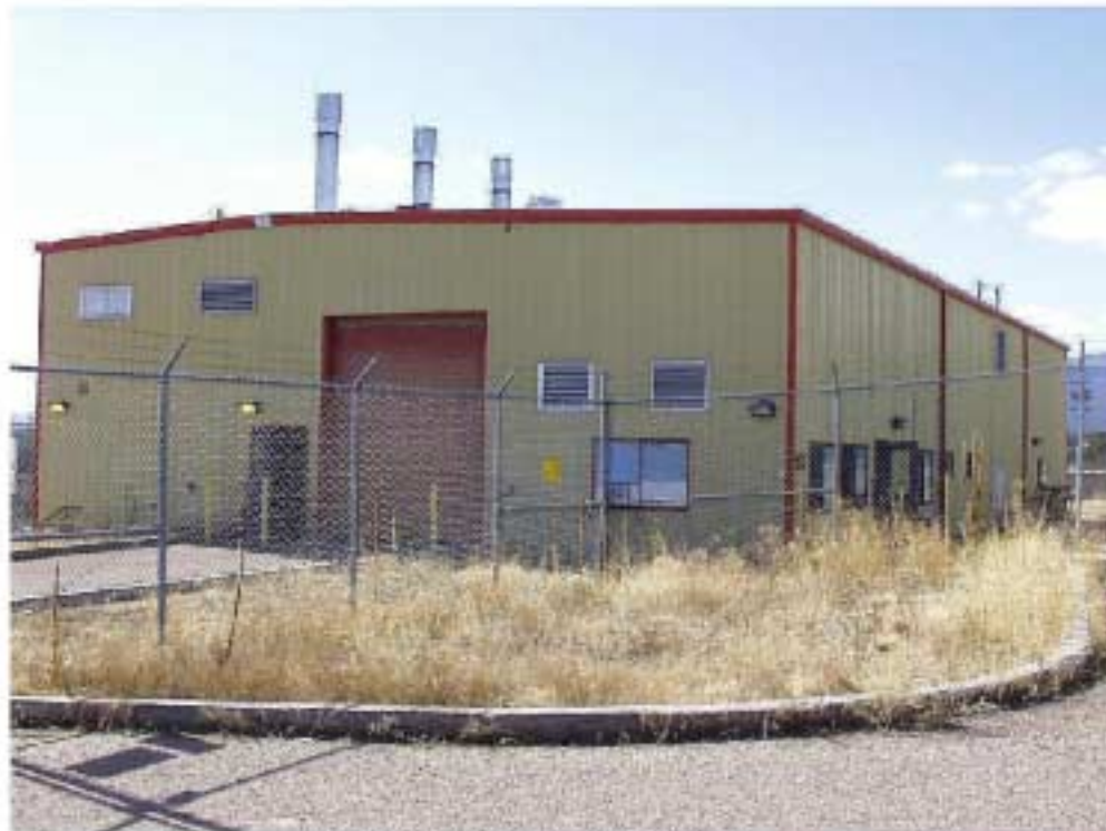
TA-21-357 East and North Elevations
