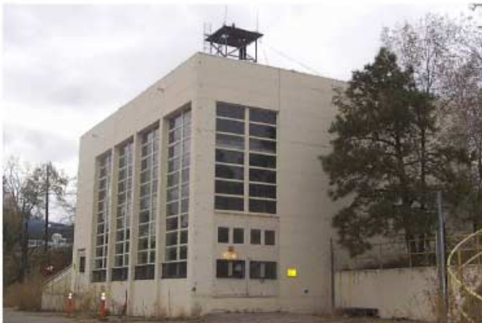
TA-43-41 South and East Elevations
