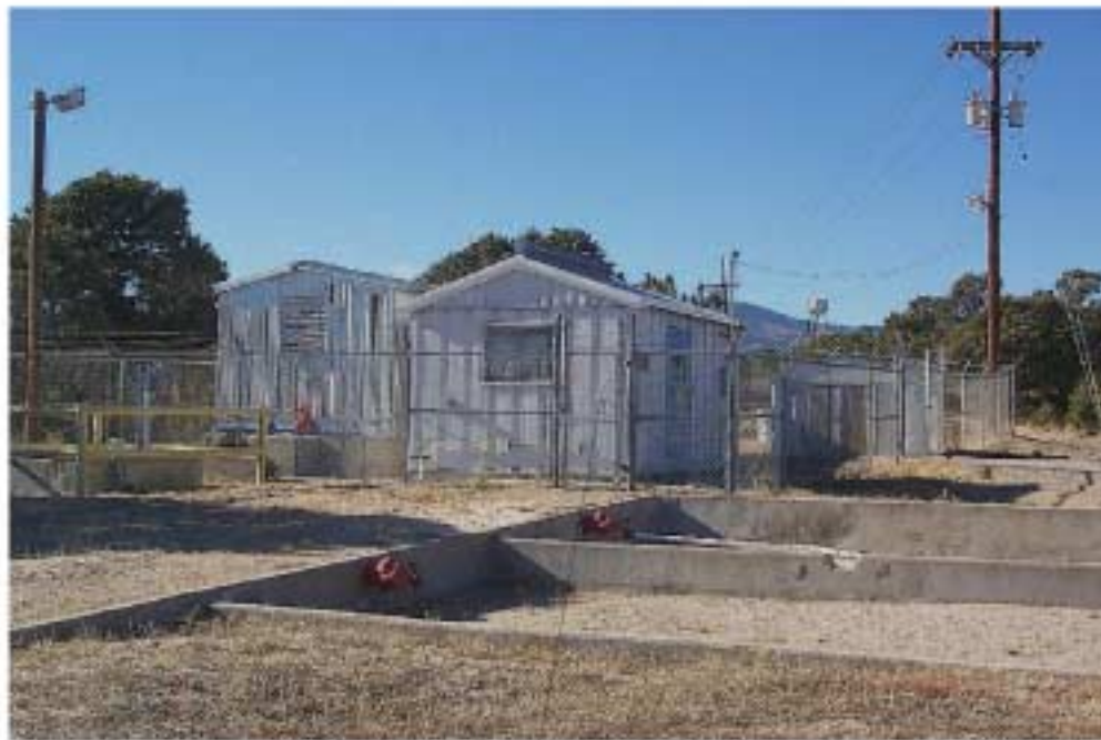
TA-21-229 East and North Elevations
