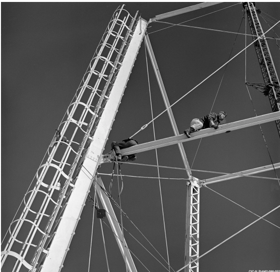
Figure 63. Workers dismantling the tower structure.
