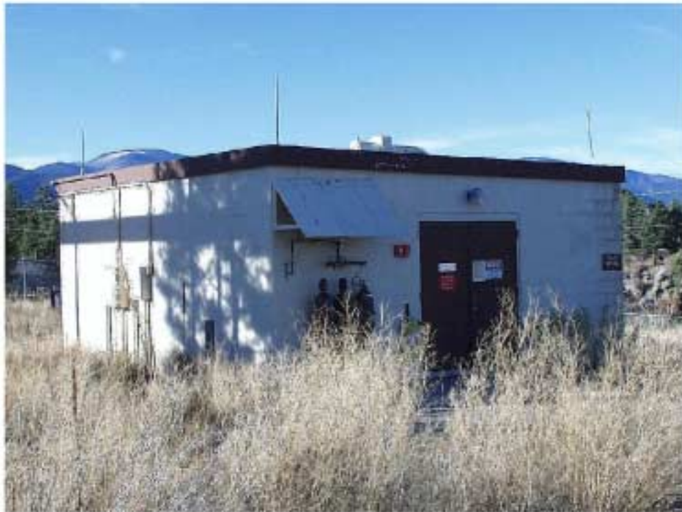
TA-21-212 South and East Elevations
