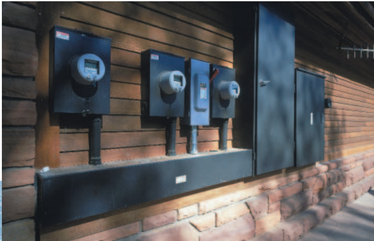
End-use metering provides a good indication of how sub-systems are operating in a building. Sub-meters are recommended for HVAC, lighting, and plug loads. Recording and tracking this information is useful for evaluating the start-up and efficiencies of sub-metered systems.
