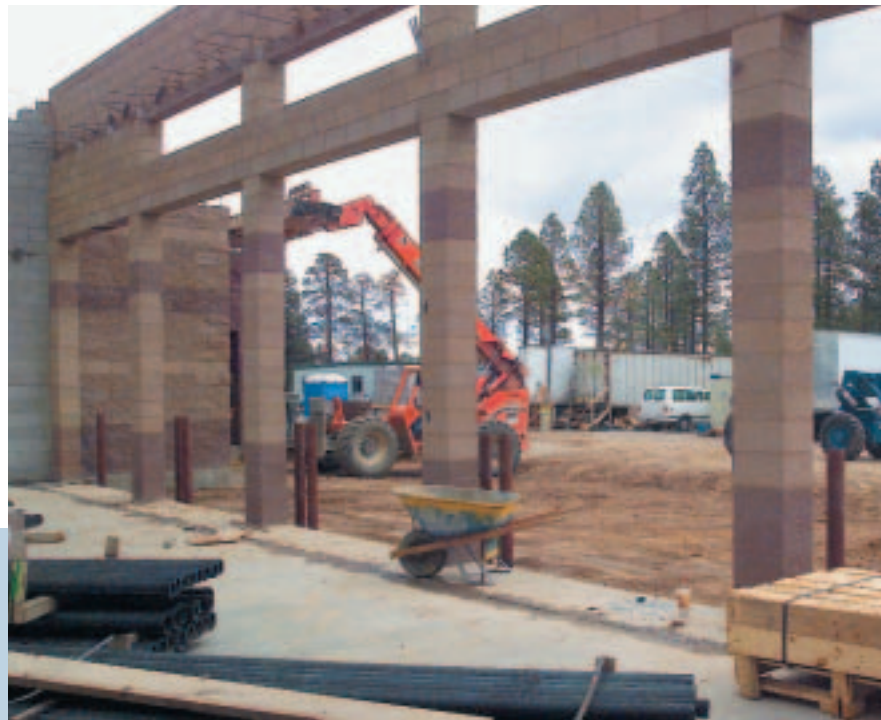
The LANL Emergency Operations Center under construction.
