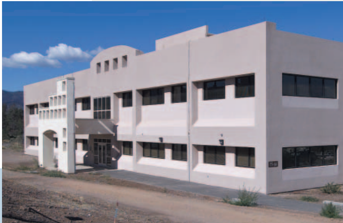
The architectural facade recesses surrounding the south-facing windows also serve as window overhangs to shade the windows and minimize direct solar gains. Placing the windows at the top of these recesses further enhances the effectiveness of these overhangs.
