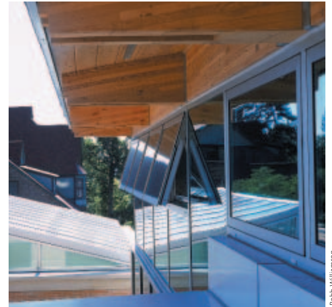
Operable clerestory windows automatically open when natural ventilation is appropriate for cooling the Lewis Center for Environmental Studies at Oberlin College in Oberlin, Ohio.
