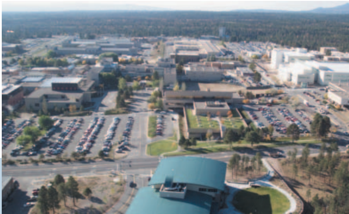
Note in this aerial photo of the Core Area of LANL the amount of land used for automobile parking and circulation.
