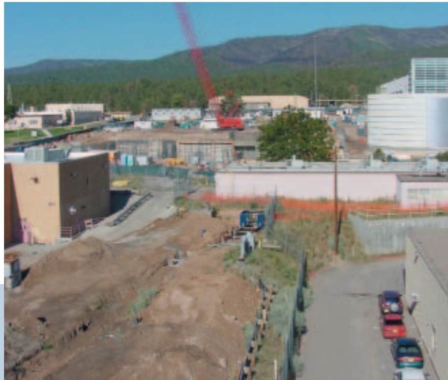
The LANL Non-Proliferation and International Security Center (NISC) was constructed on a previously distributed site.
