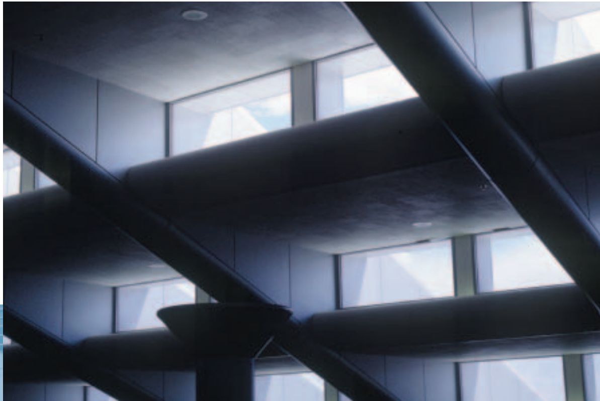
Designers carefully selected glazing with a low solar heat gain coefficient to maximize daylighting and minimize solar gains for the Solar Energy Research Facility at the National Renewable Energy Laboratory in Golden, Colorado.
