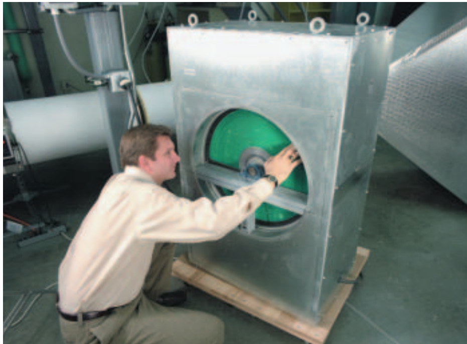
Examining a desiccant wheel upon delivery to the construction site.
