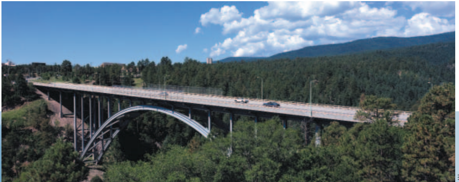
The Los Alamos Canyon Bridge opened the way for LANL growth onto the South Mesa.
