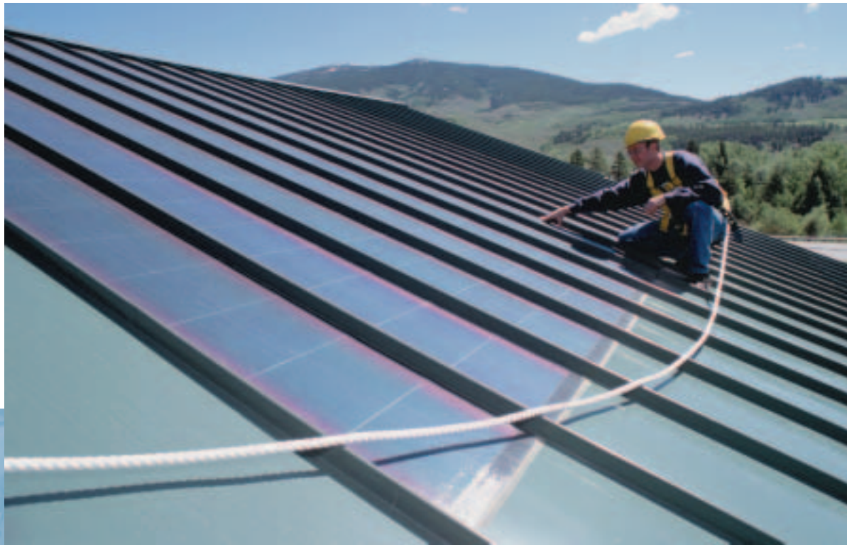
PV modules integrated as a part of the standing seam metal roof system.
