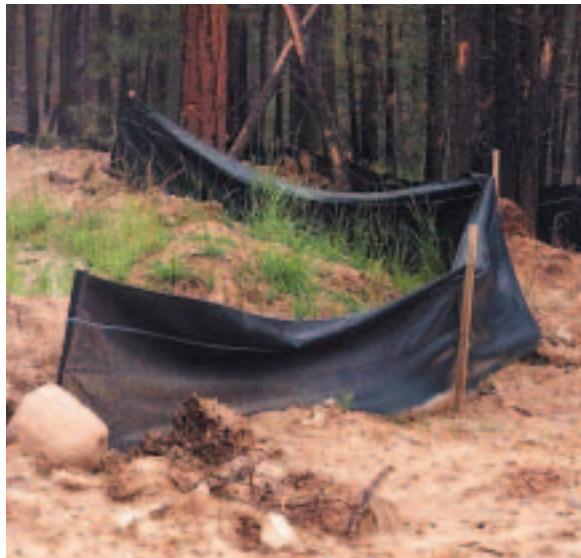
A silt fence is used to control erosion.
