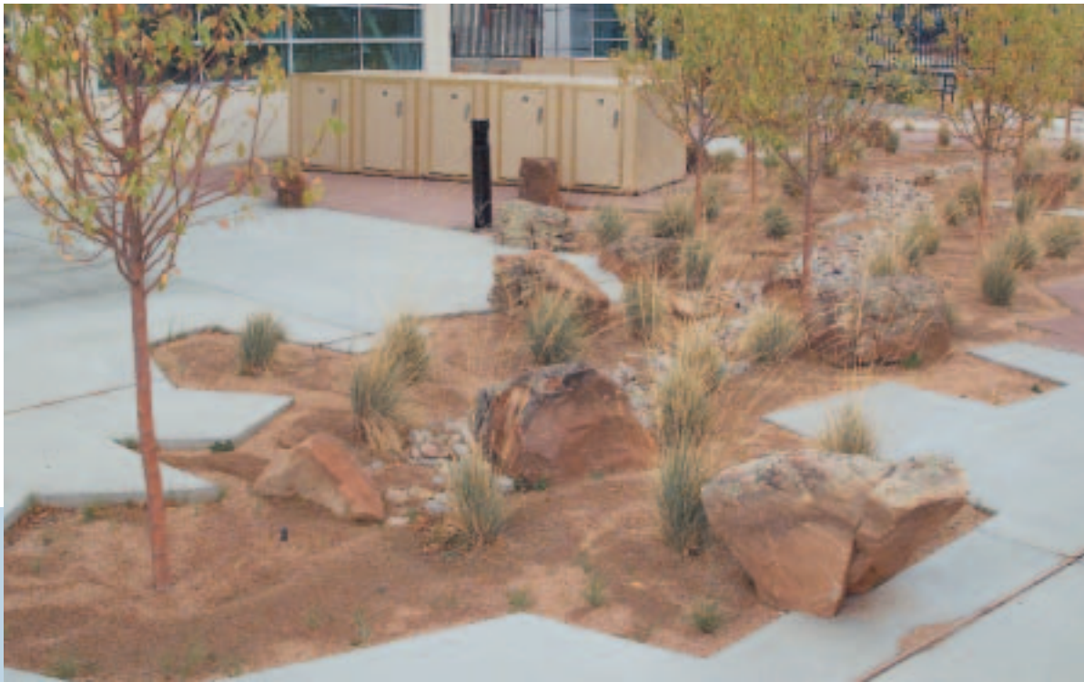
Limiting the use of impermeable paving helps control runoff and protects the watershed.
