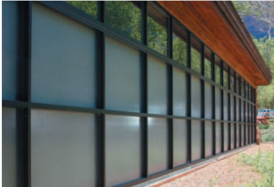
Trombe walls absorb heat during the day and release it into the space at night. An overhang shades this Trombe wall in summer when passive heating is not needed. View glass above this Trombe wall provides daylight to the interior space.
