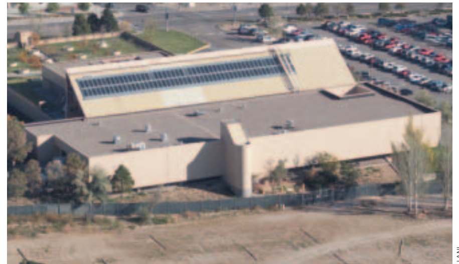
The solar domestic hot water system for the LANL Otowi Building is mounted flush with the roof.
