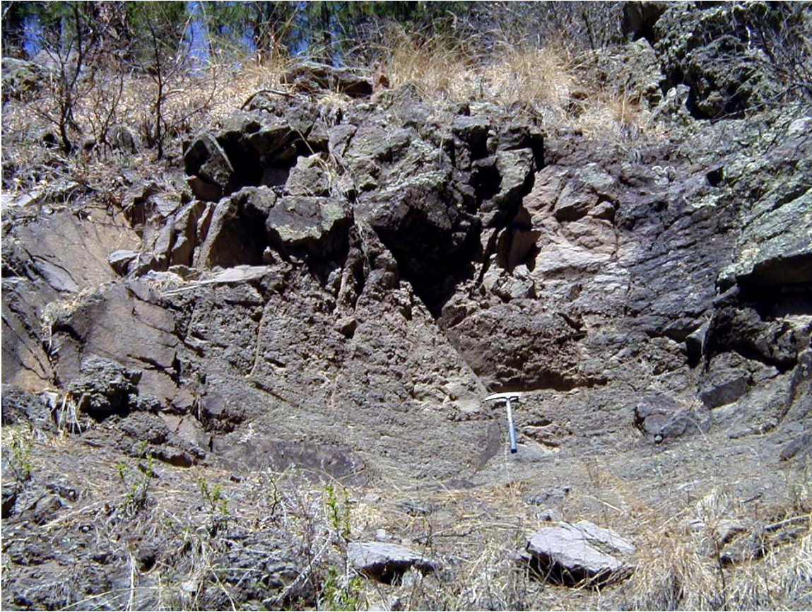
Figure E.6-2. Photograph of weathered, fractured andesite lava exposed in bluff downstream and east of Pine Spring.
