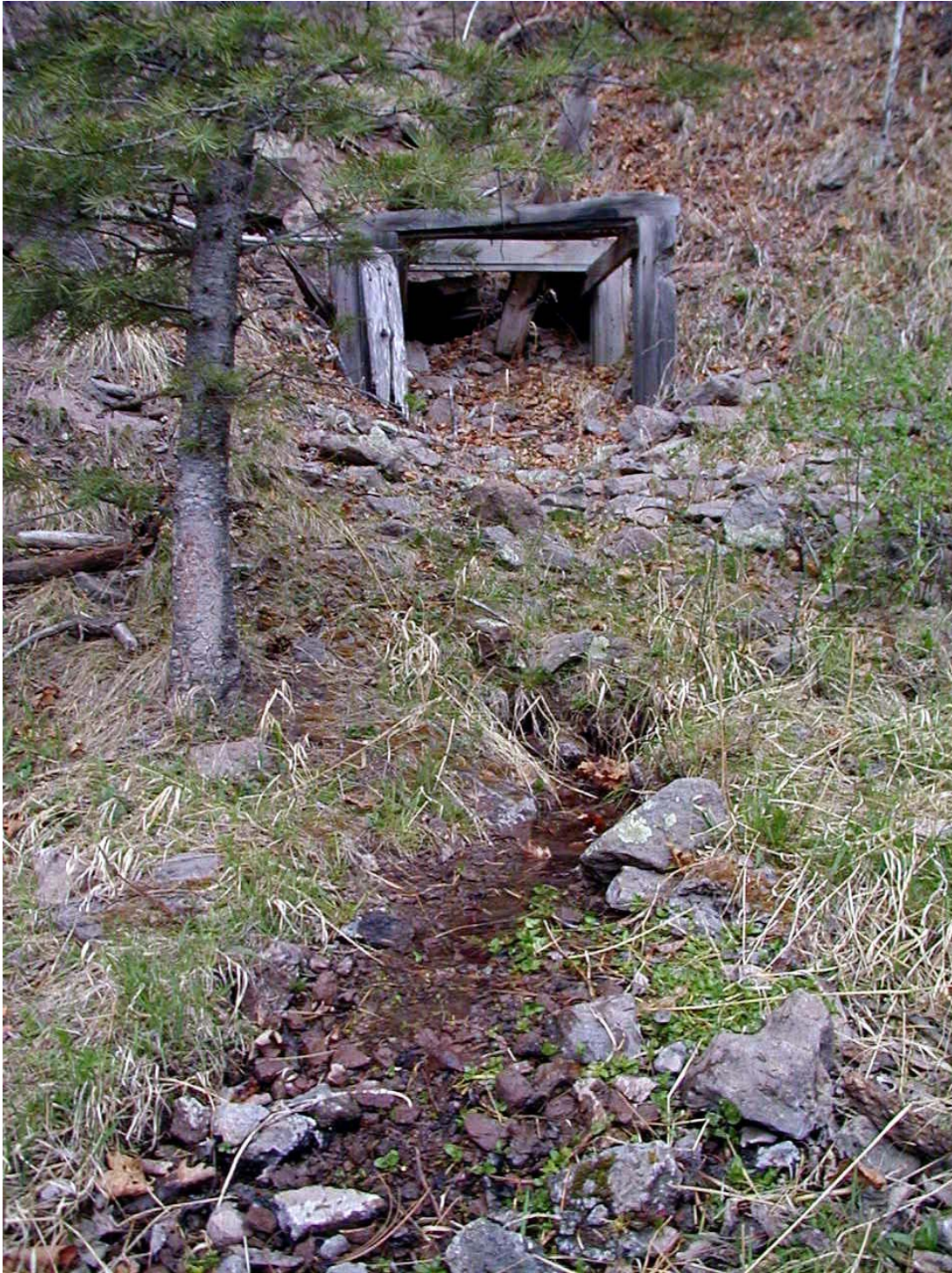
Figure E.10-1. Photograph of Upper Cañon de Valle Spring taken on April 29, 2000; the temperature is 15°C, and the flow rate is 0.8 L/min
