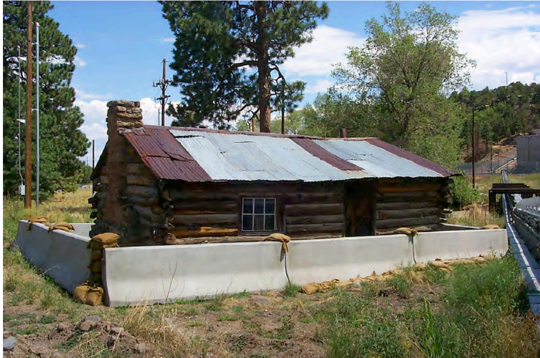
Figure 22.4. The Pond Cabin was enclosed to protect it from possible flash flooding after the Cerro Grande fire.
