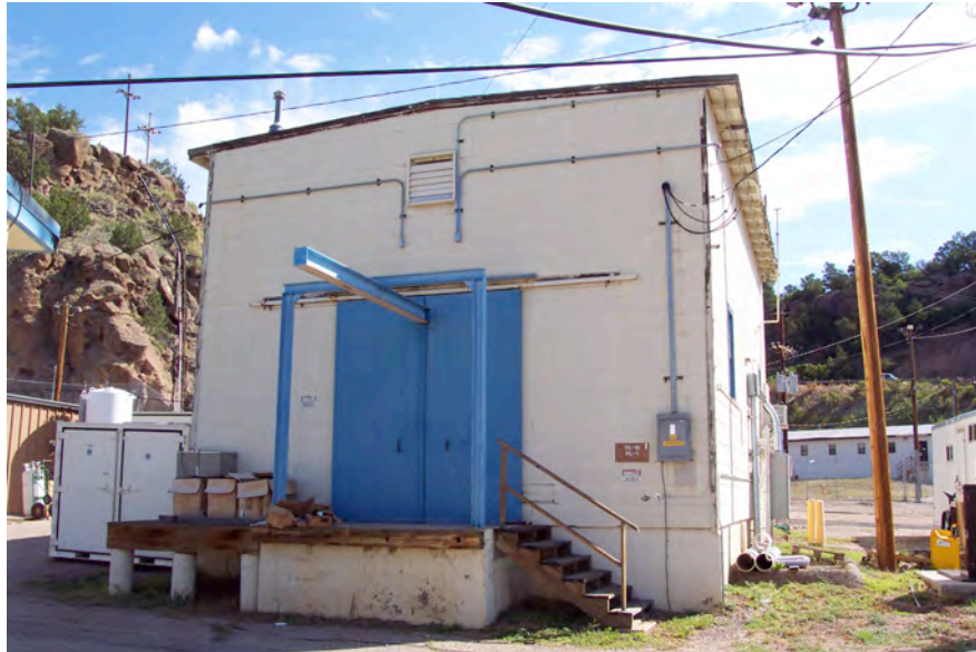
Figure 15.9. Building 18-1, site of a fatal criticality accident.
