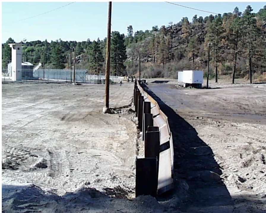
Figure 6-10. Steel diversion wall under construction.
