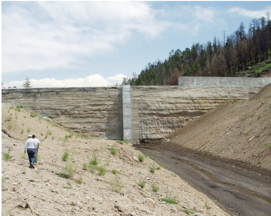
Figure 6-9. Flood retention structure, looking east.
