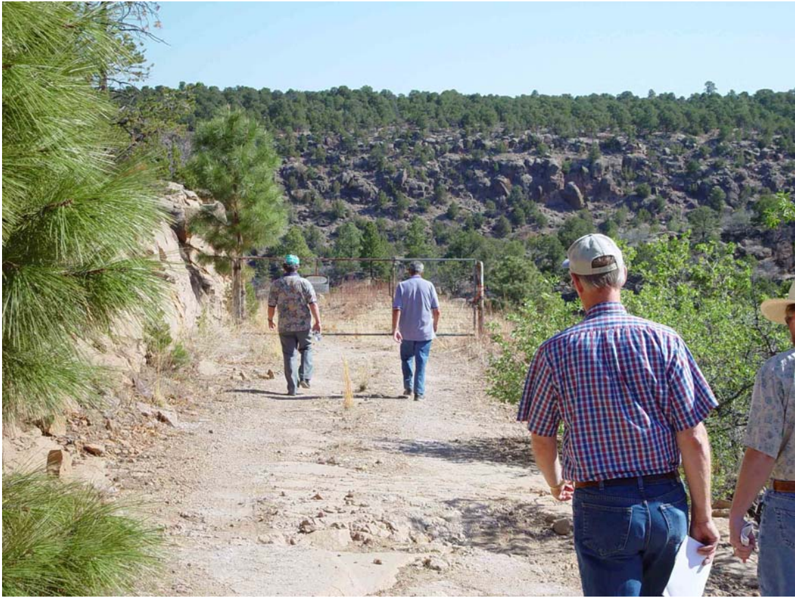
Photo 49A-2: The road entering the ravine from the south is steep and cut into tuff.
