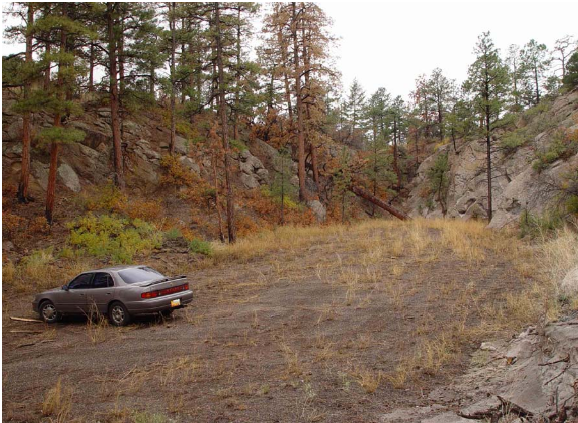
Photo 60-1: The head of the site looking west. The head of the site is a western “finger” that protrudes into the side of Sigma Mesa. This is shown in the middle of the photo, where a fallen tree is located. Control of water entry to the landfill from the mesa top would occur at this point. The initial waste bale cells would be constructed just to the east of this point, with the leachate collection ponds just down-gradient.
