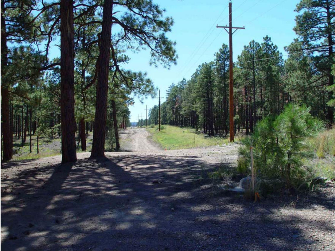
Photo 58-1: The site is split by a utilities corridor running north to south. This is a view to the south.
