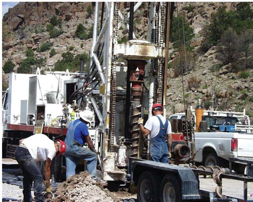
Drilling auger and crew
