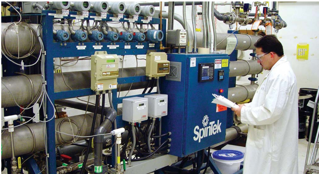
One of the radioactive liquid waste operators prepares to start the reverse osmosis unit
