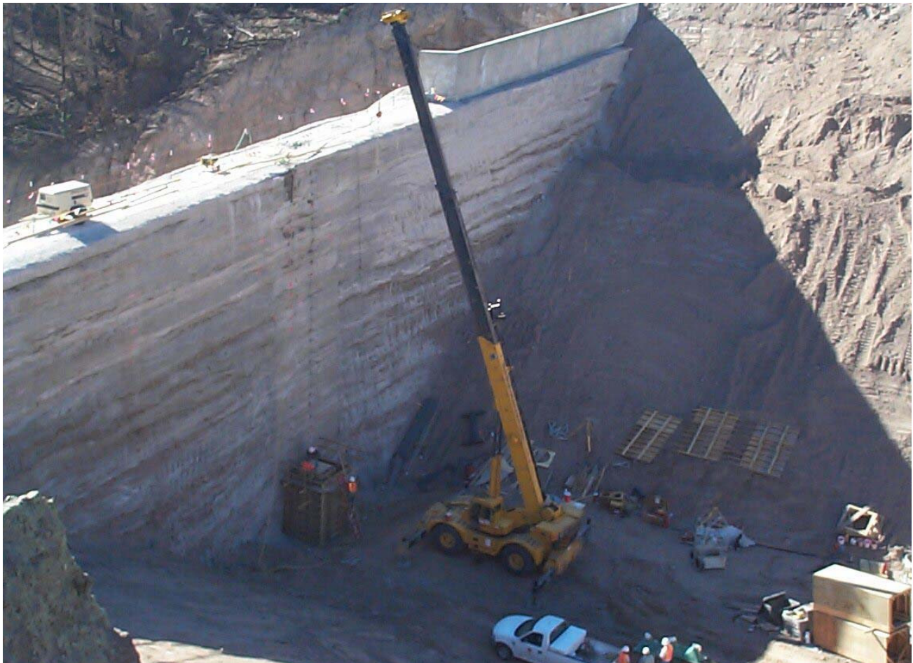
Flood retention structure during construction
