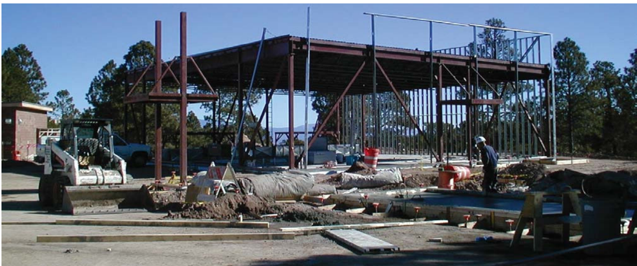
Construction of the BSL-3 facility
