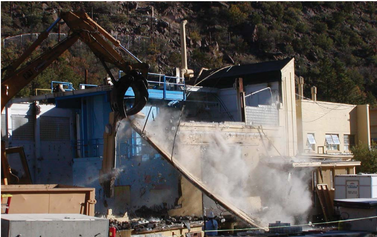
Demolition of the Omega West Facility
