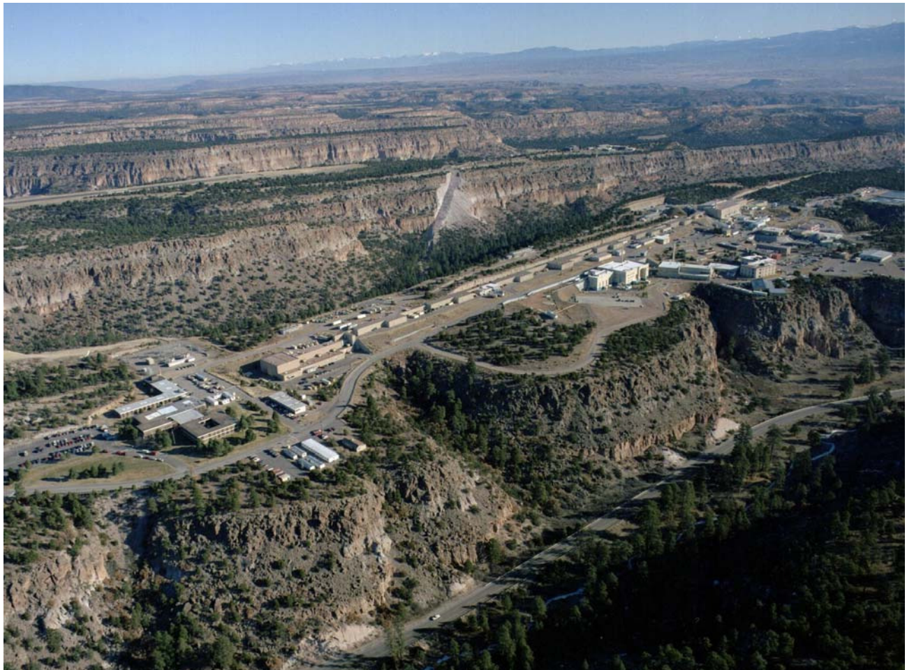
The LANSCE Key Facility
