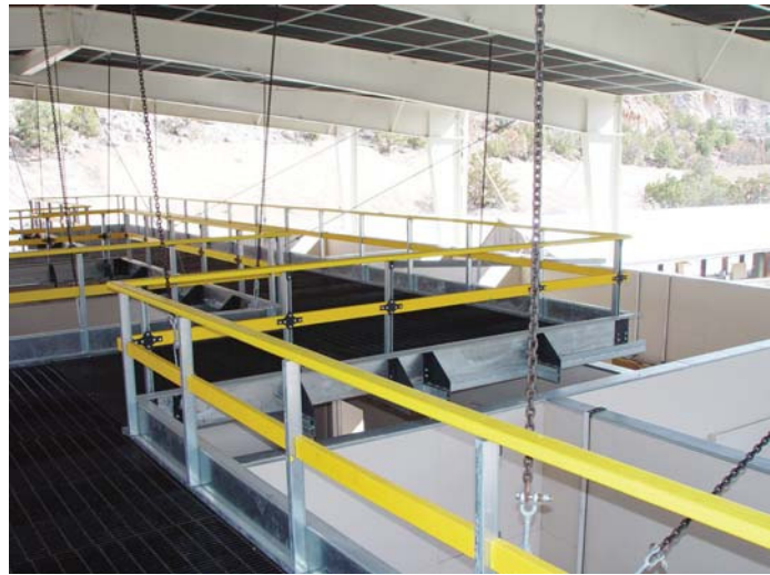
The suspended catwalk observation platform in the Live Fire Shoot House
