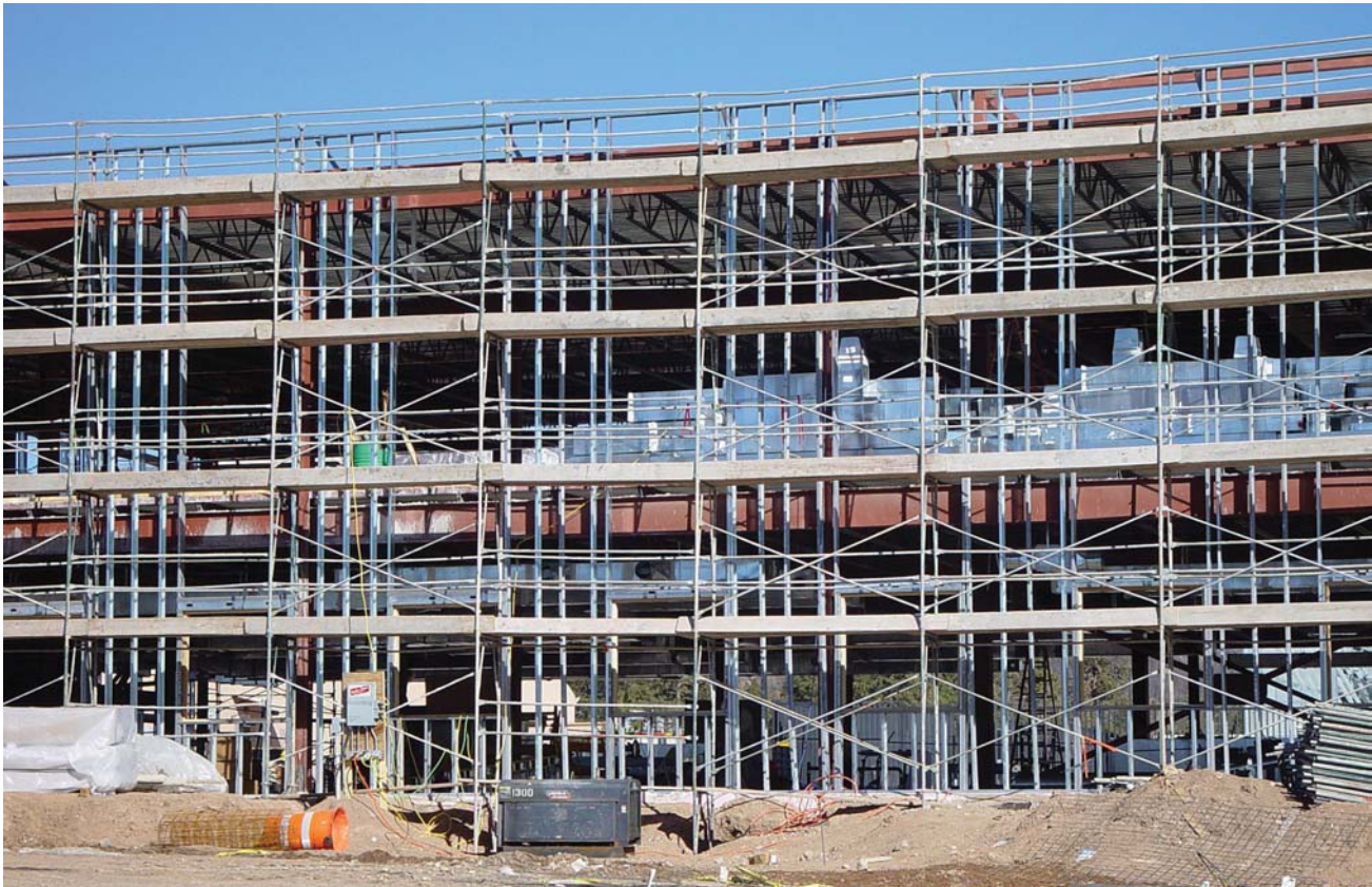
Decision Applications Division Office Building under construction
