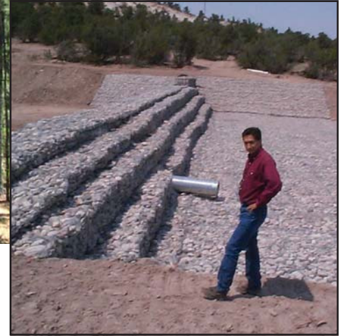
Low-head weir near the White Rock Y
