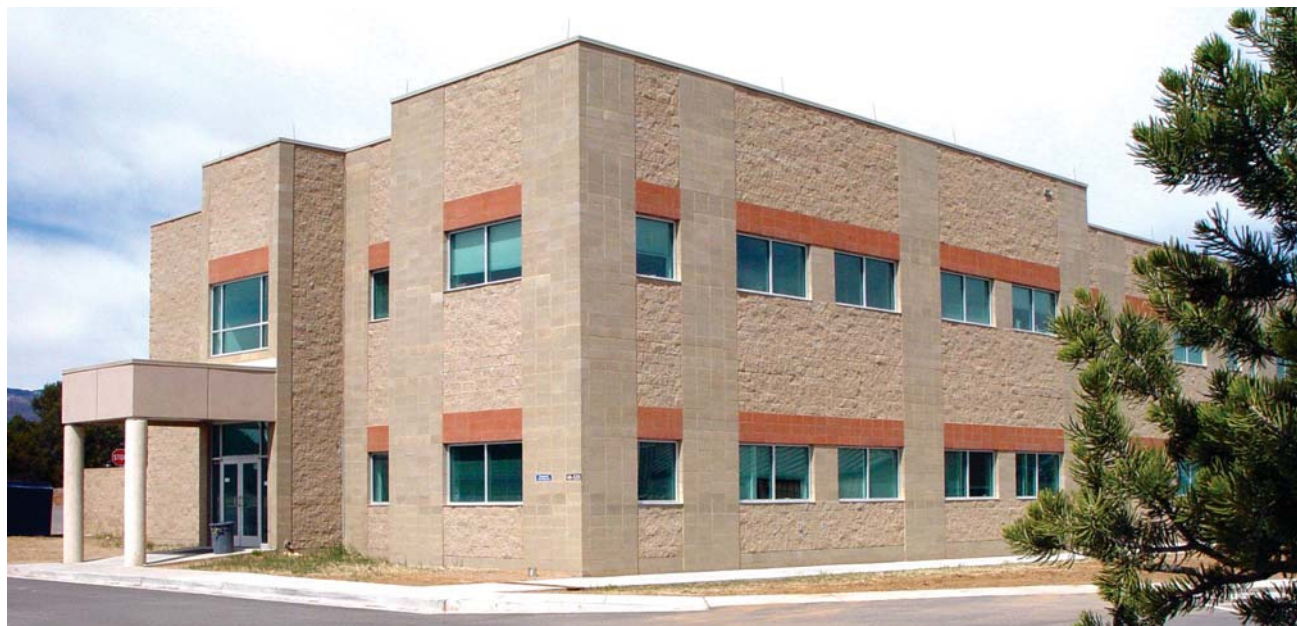
Chemistry Technical Support Building
