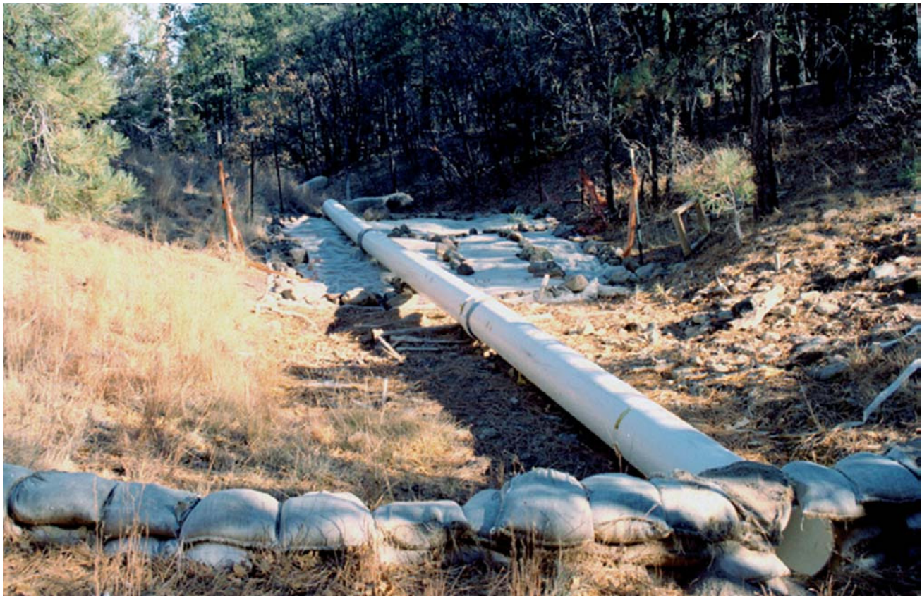
Stabilization measures below the deleted TA-16 Building 260 Outfall
