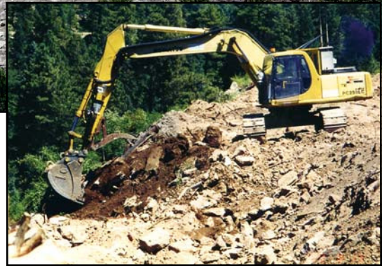
MDA-P after ER Project remediation activities (top), Remote-controlled equipment in use to remove detonable high explosives from MDA-P (right)
