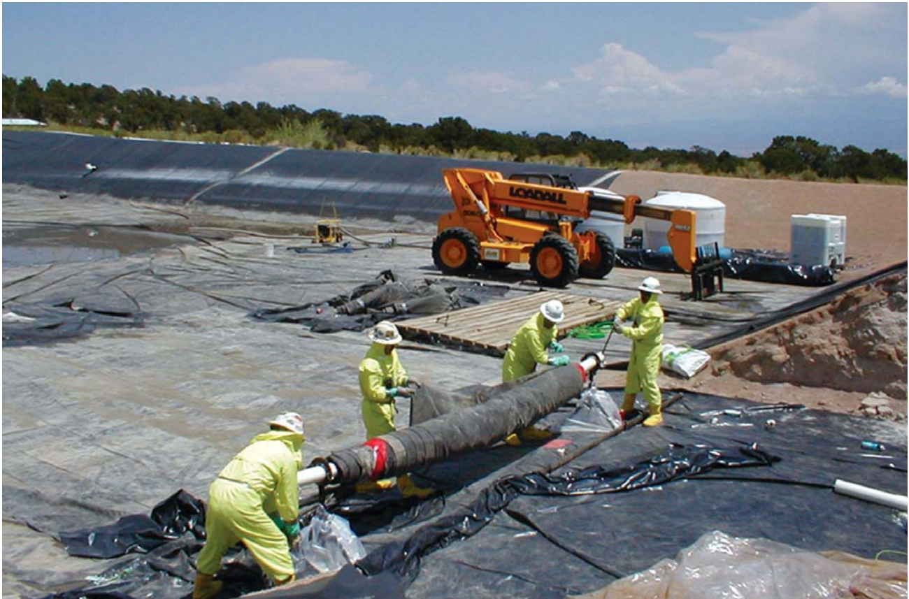
Removal of dried radioactive sludge and the plastic liner from a lagoon at LANSCE
