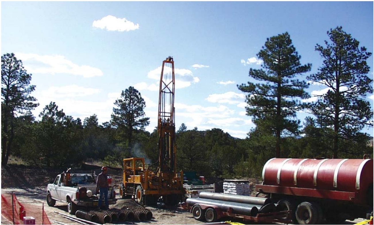
Cleaning the drilling residues from a regional aquifer well
