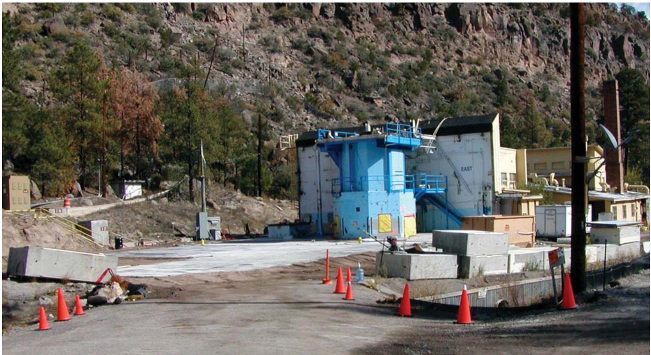
Blue structure—Omega West Reactor housing
