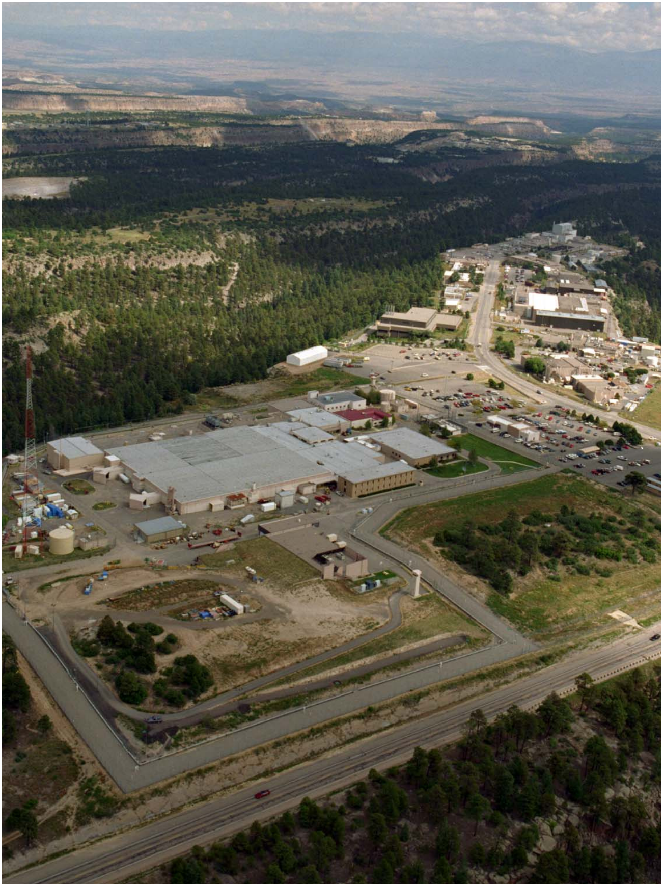
Aerial view—North from Pajarito Road
