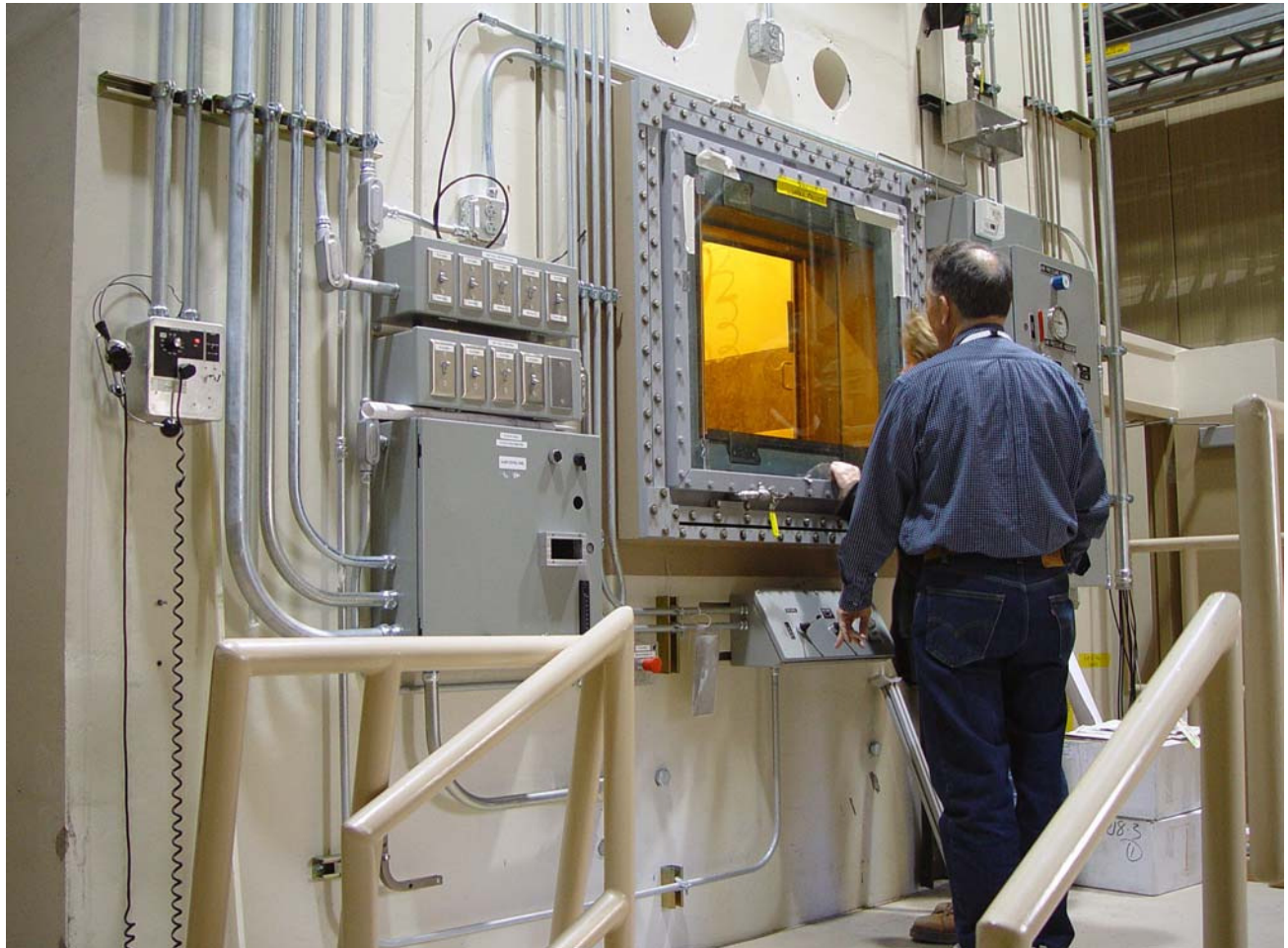
A hot cell in the new Isotope Production Facility at LANSCE
