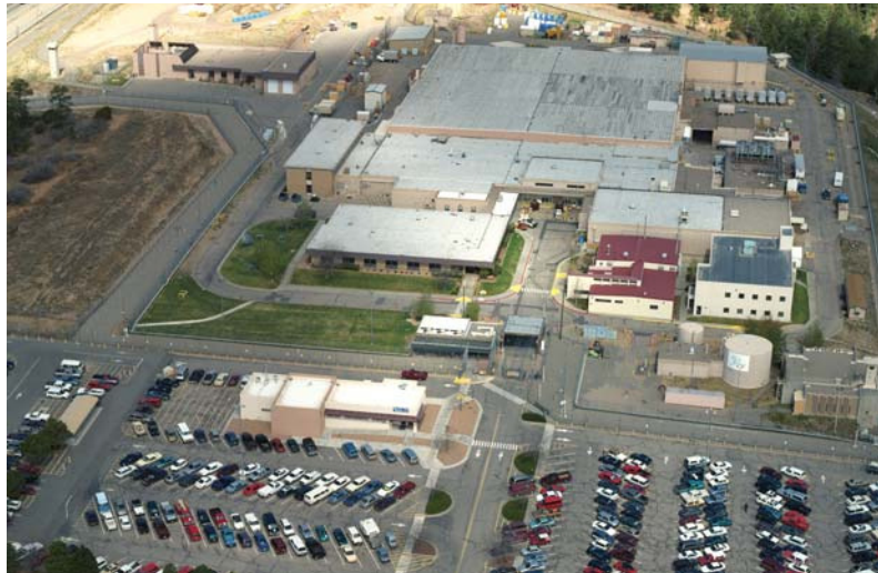
Aerial view of the Plutonium Complex (TA-55)
