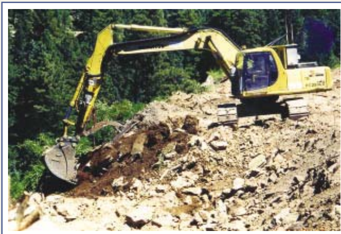
Historical photograph (circa 1965) of MDA P (above). Remote-controlled equipment in use to remove detonable high explosives from MDA P (left). MDA P after ER Project remediation activities (below).
