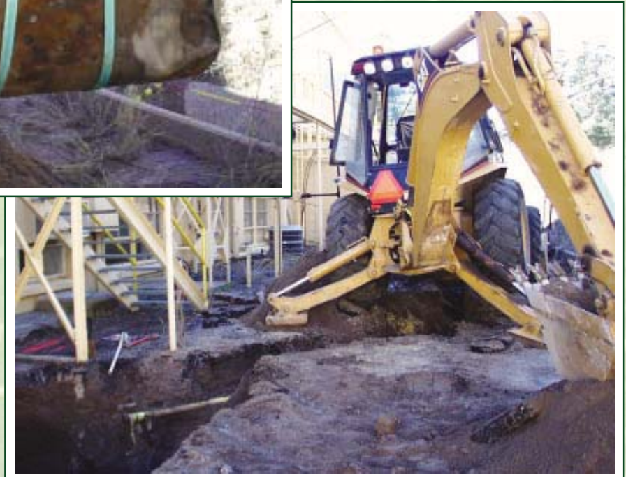
Underground storage tank removal at Technical Area 2 located in Los Alamos Canyon.
