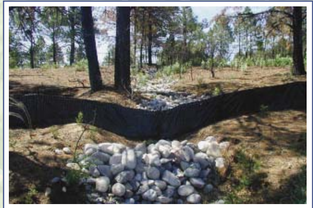
Erosion control measures installed to stabilize soils.
