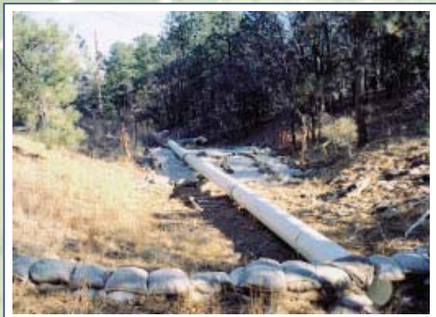
Stabilization measures at 260 Outfall.
