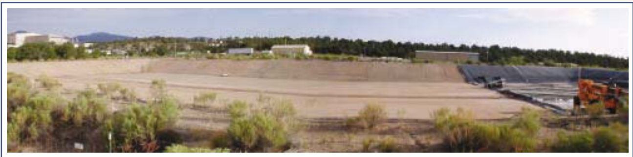
Lagoon remediation efforts almost completed.
