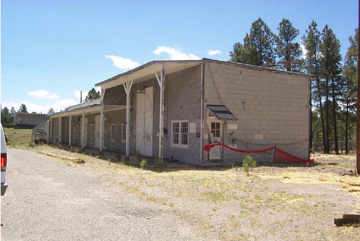
Figure 11.11. TA-16-515 at V-Site before the Cerro Grande Fire.
