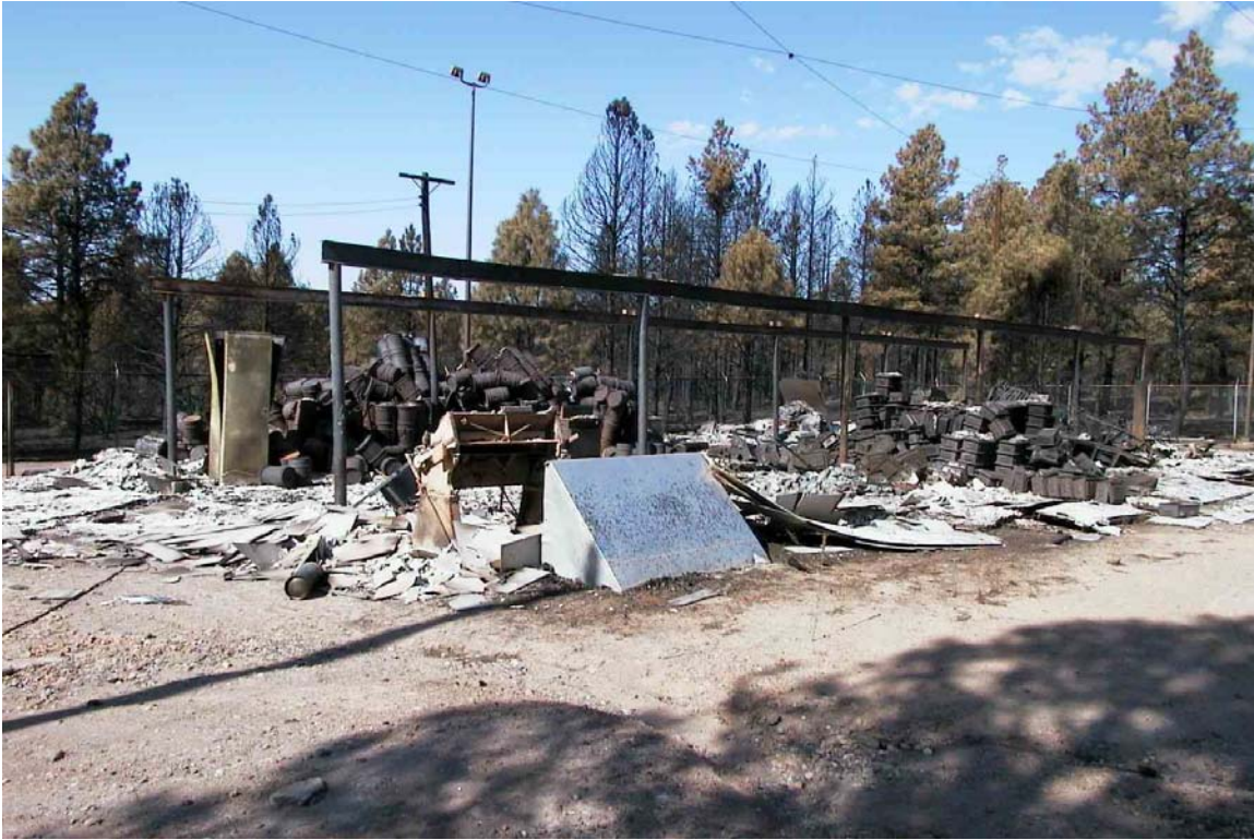
Figure 11.13. TA-40-72 after the Cerro Grande Fire.
