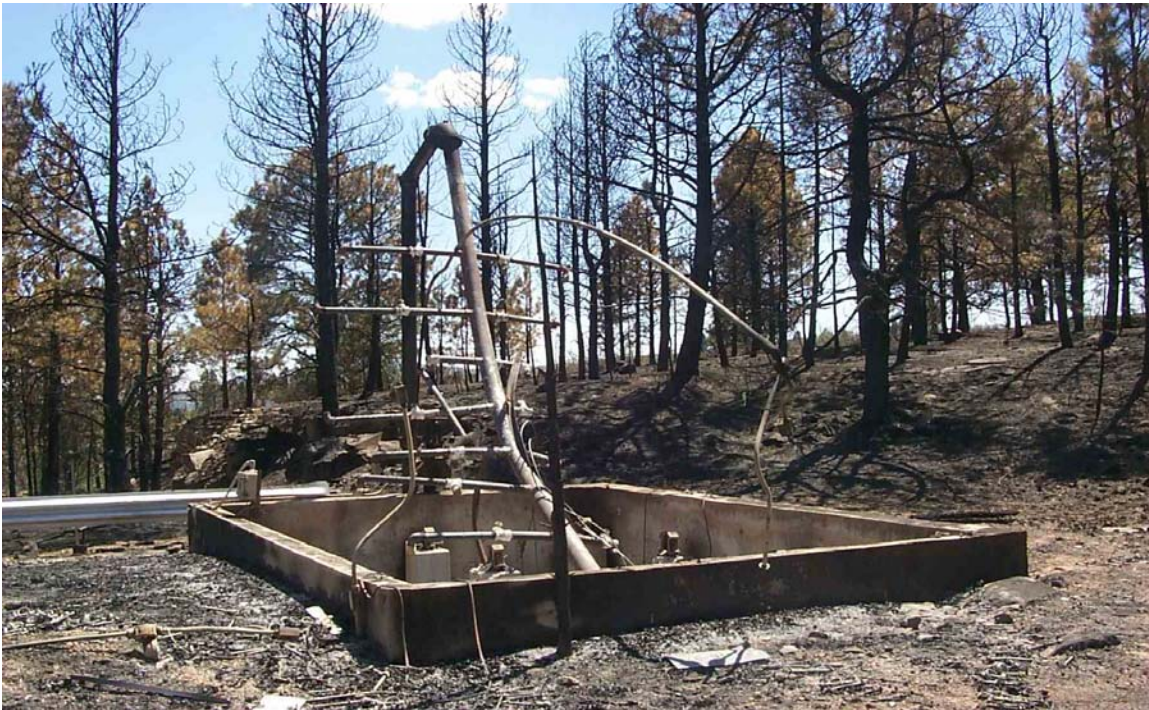
Figure 11.17. TA-16-372 after the Cerro Grande Fire.
