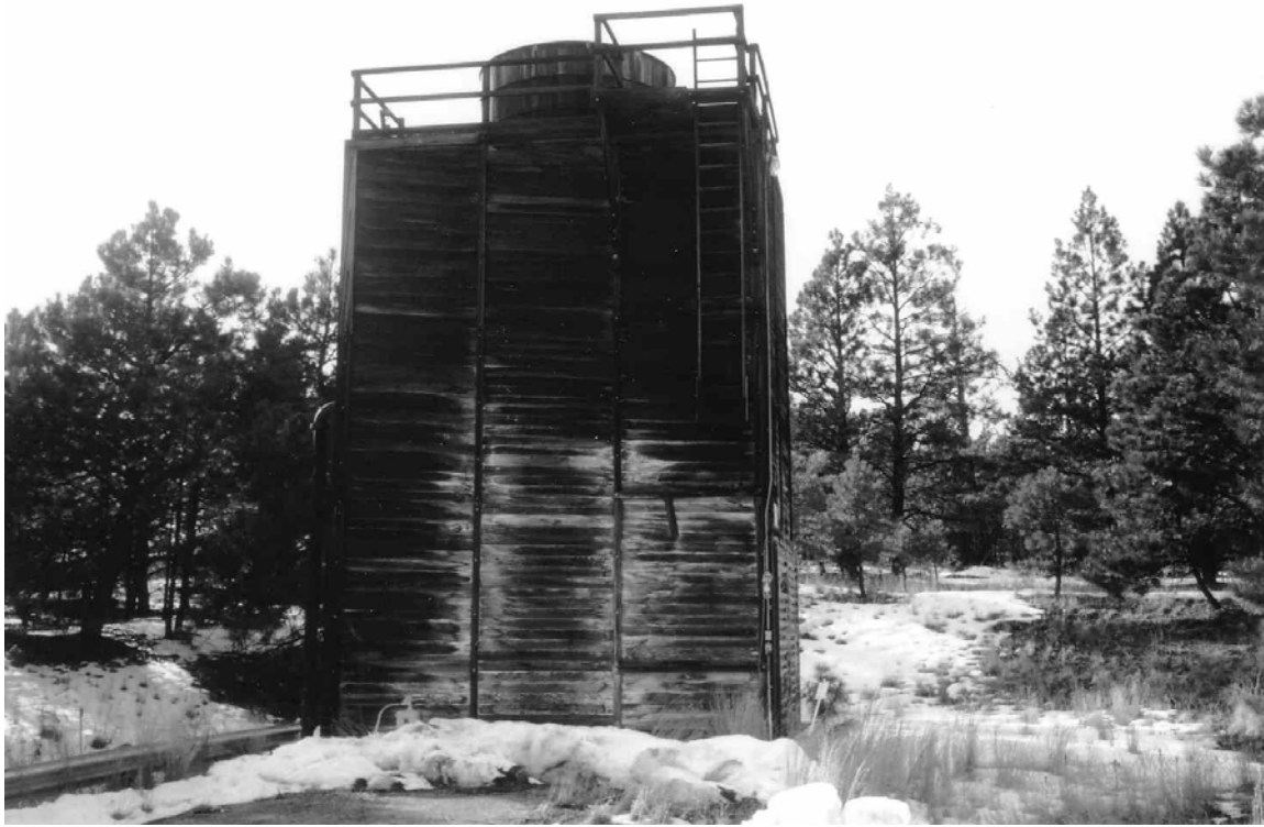
Figure 11.16. TA-16-372 before the Cerro Grande Fire.
