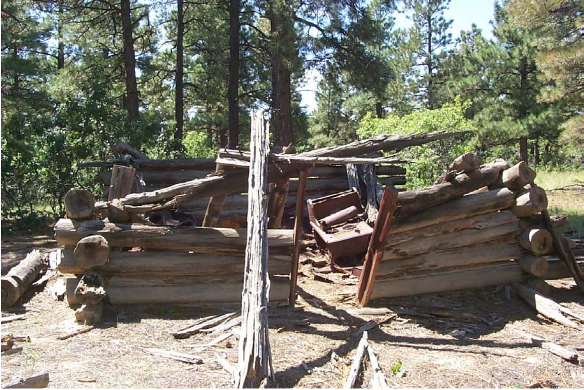
Figure 11.1. LA 21334, the Montoya cabin on Two-Mile Mesa before the Cerro Grande Fire.
