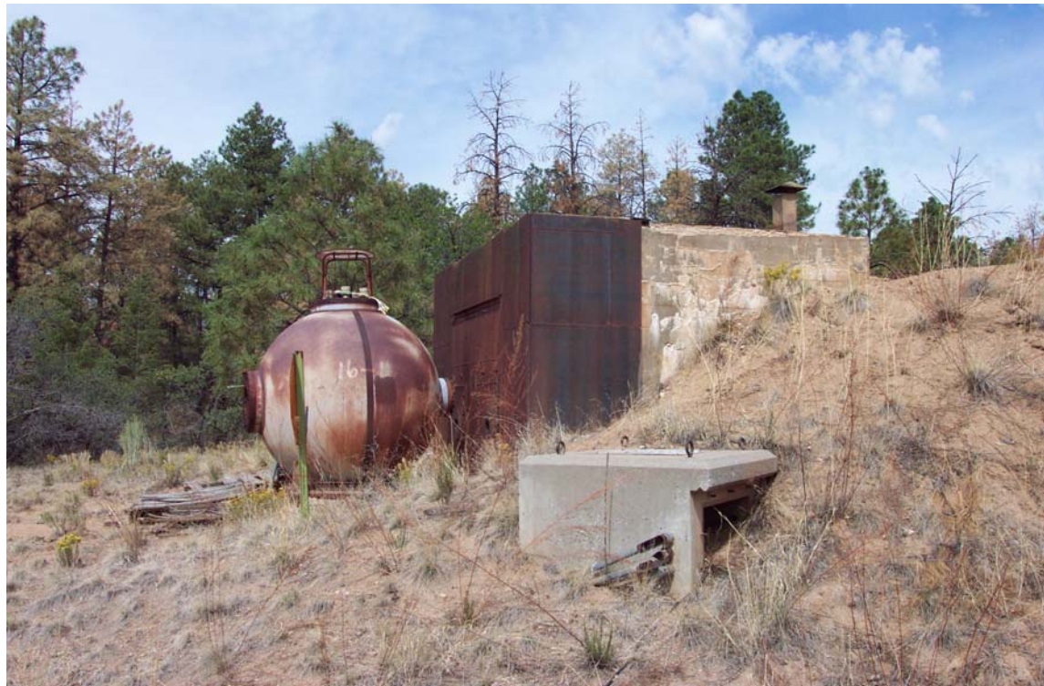
Figure 11.10. TA-14-5, rear view of former control room and berm after the Cerro Grande Fire.
