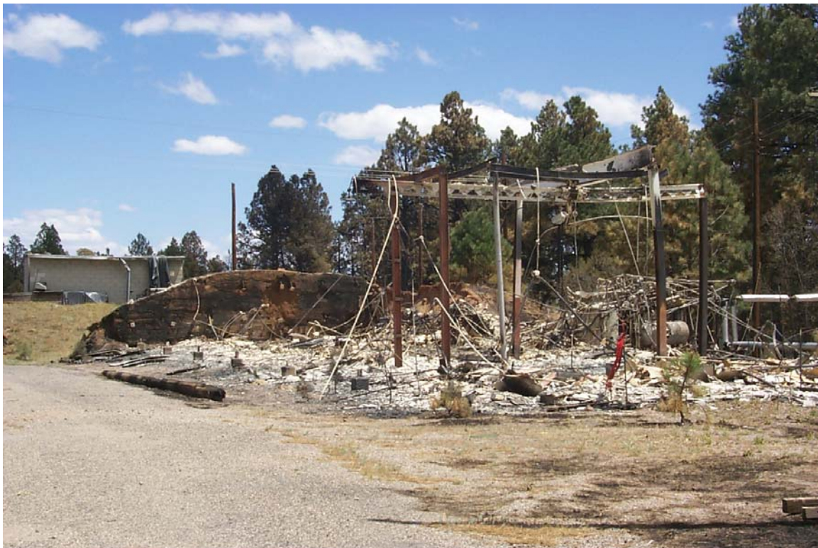
Figure 11.12. TA-16-515 after the Cerro Grande Fire.
