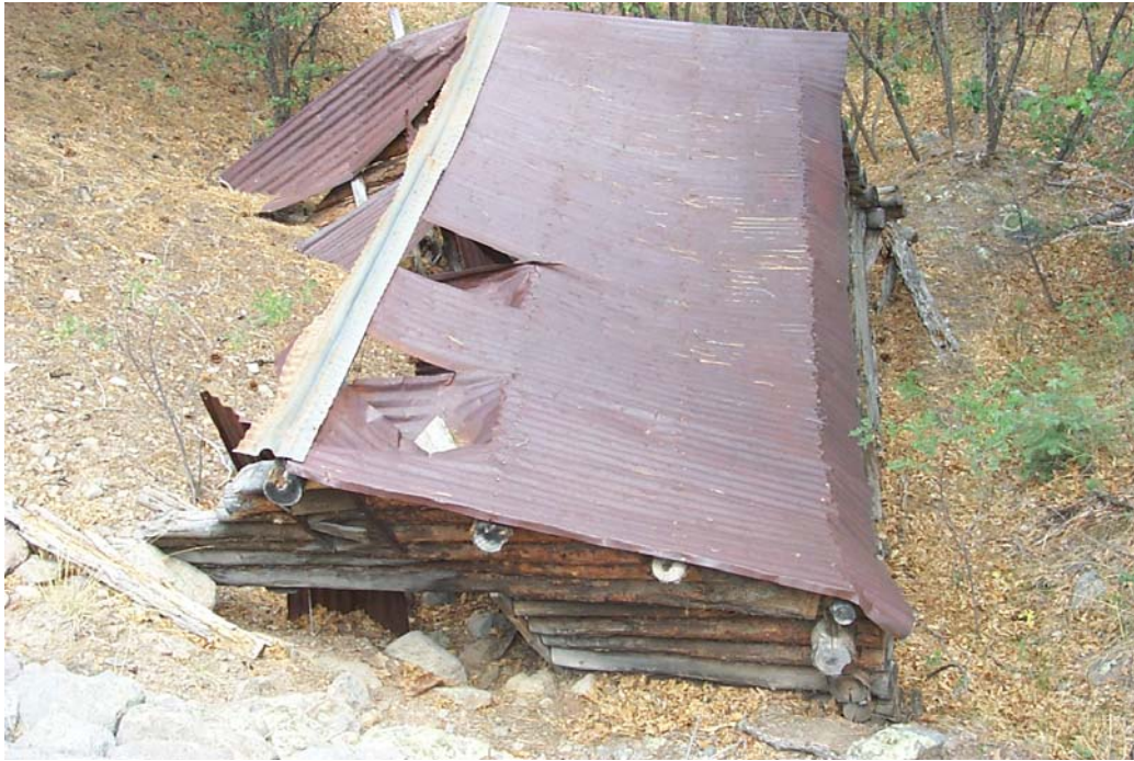
Figure 11.5. The Ice House at Anchor Ranch (pre-flood and pre-fire).
