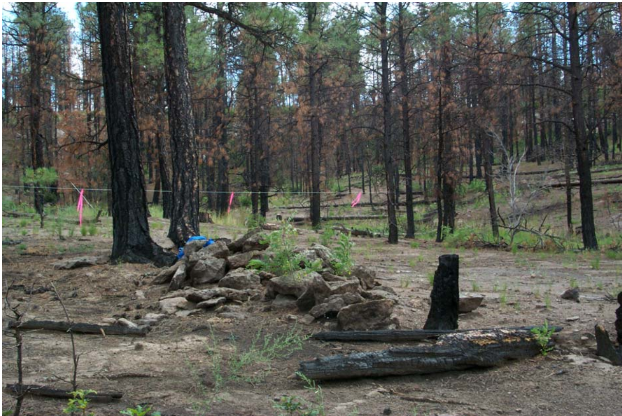
Figure 12.3. LA 21298, a Historic period structure after the Cerro Grande Fire.
