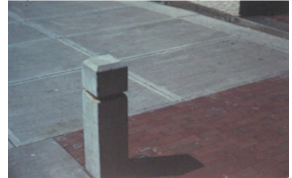
Image IV-35: Textured Concrete Paving Finish Patterns
