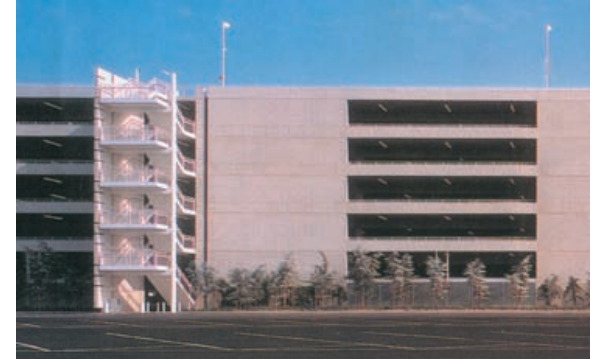
Image IV-4: Parking Structure Example - concrete panel
