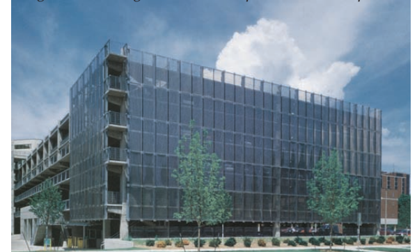
Image IV-5: Parking Structure Example - wire mesh panel
