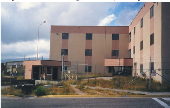
Image IV-12: Before image of security fencing
