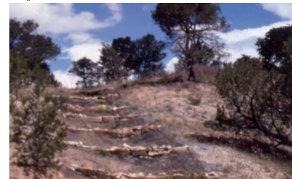
Image IV-3: Erosion Control - Check Dams
