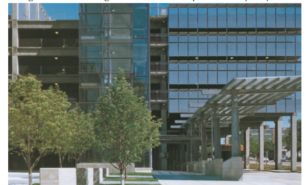
Image IV-6: Parking Structure Example - entryway
