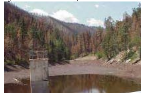
Figure IV-14: Water Reservoir, after Cerro Grande Fire
