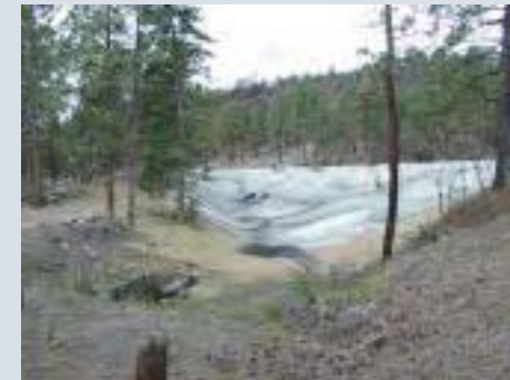
Figure IV-5: Flooding Control Structure
