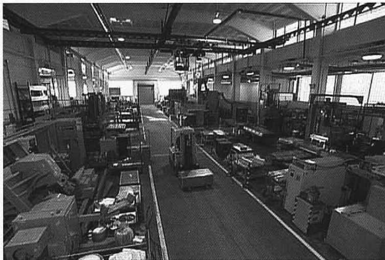
Machine Shops showing numerical-controlled machines
