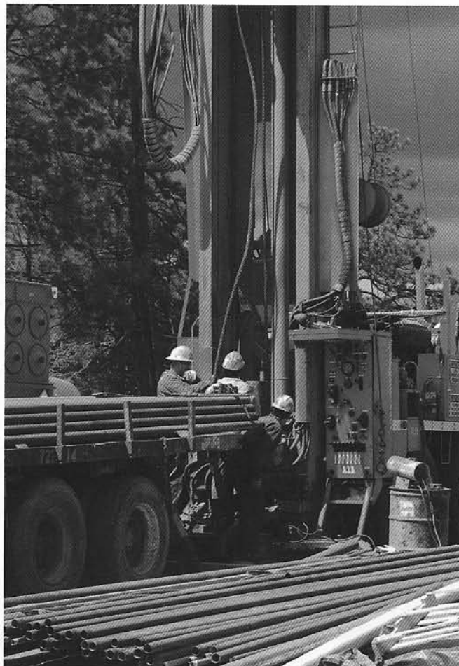
Deep well drilling rig
