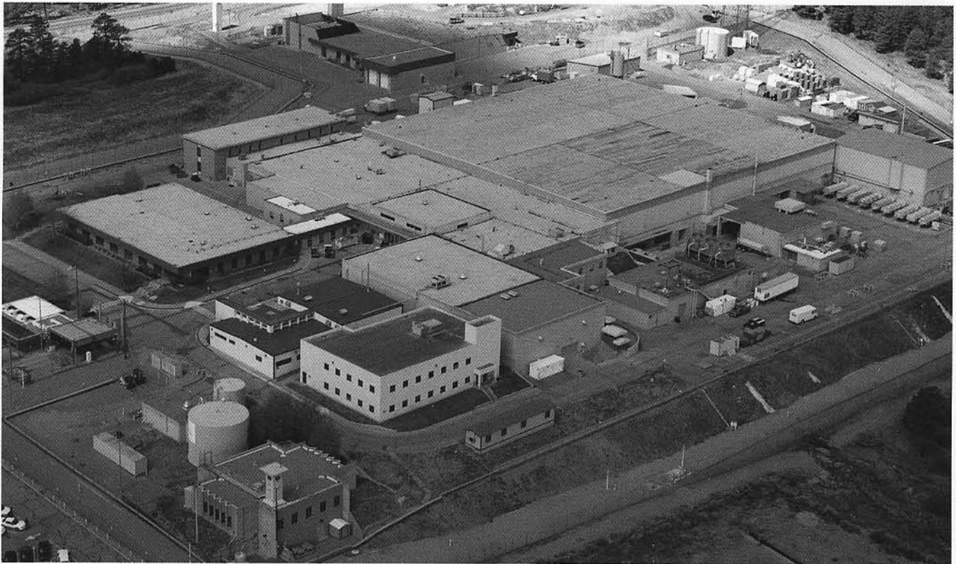
Plutonium Complex at TA-55
