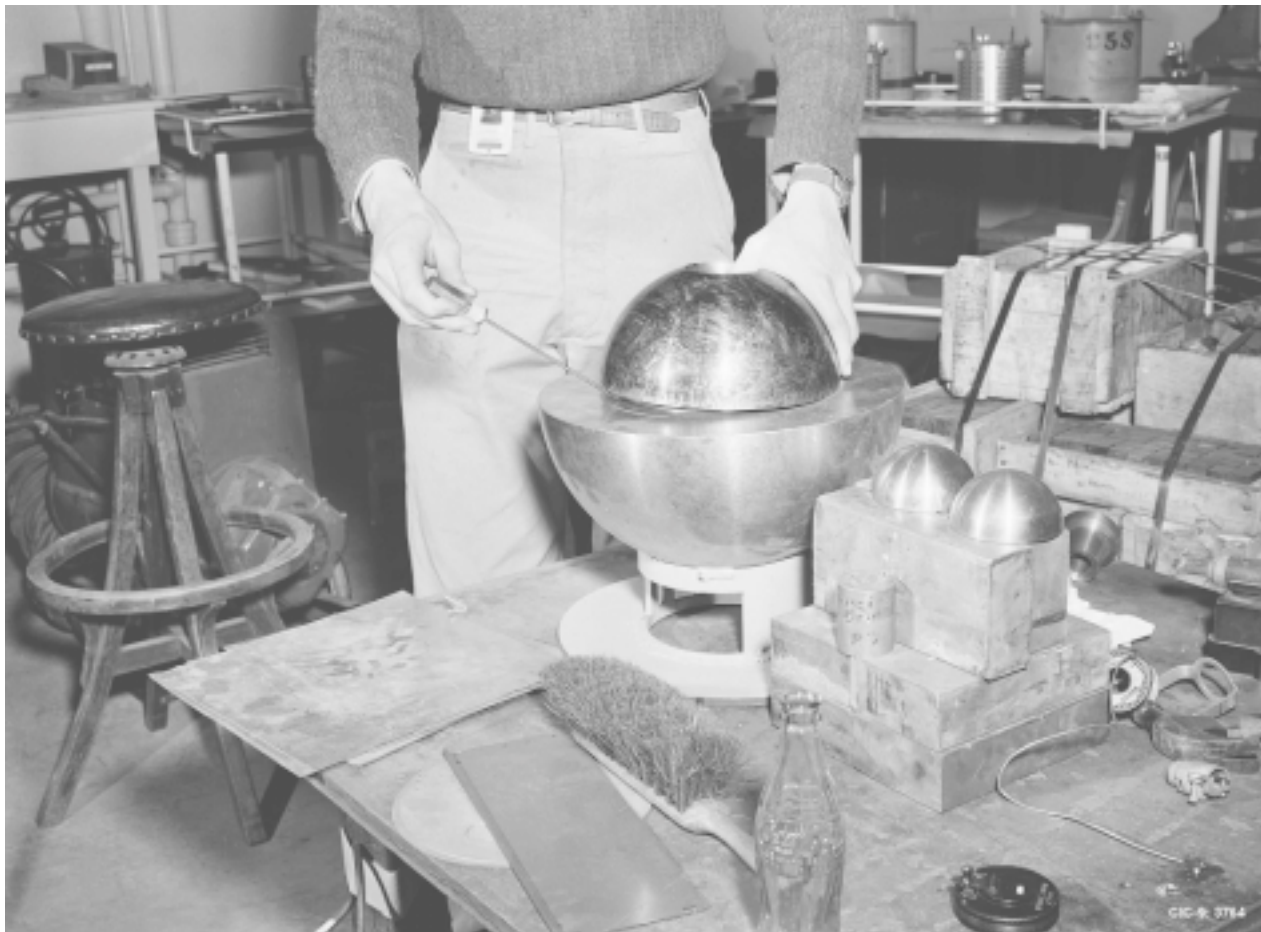
Figure 42. Configuration of beryllium reflector shells prior to the accident 21 May 1946.
