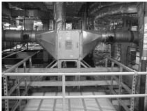
Figure 6.5 – Correct Mounting of In-Duct-HEPA Filter Housing
