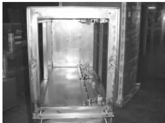
Figure 6.7 – Turned Angle, Gasket Sealing Filter Surface for a Commercial Housing (left-hand side of the photo) [Note: Right-hand side of this photo shows the four-bar-linkage gasket.]
