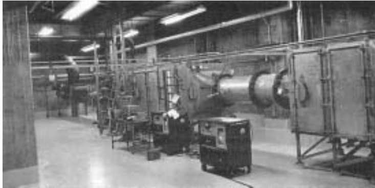
Figure 2.14 – Series-Compartmented Air Cleaning System
