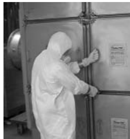
Figure 6.16 – Personnel Dress for Bag-Out Filter Change
