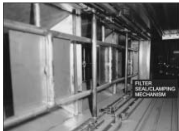
Figure 4.67 – Side-Access Housing with Test Manifold
