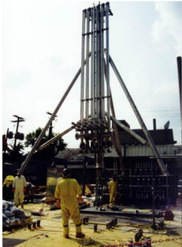
Figure 1. Installation of the jet pump skid.
