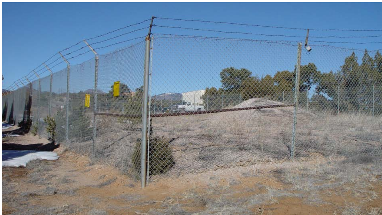
Figure 4. Material Disposal Area H at TA-54. (The mound of soil in the right forefront of the photo is clean fill remaining after the excavation of the last shaft.)
