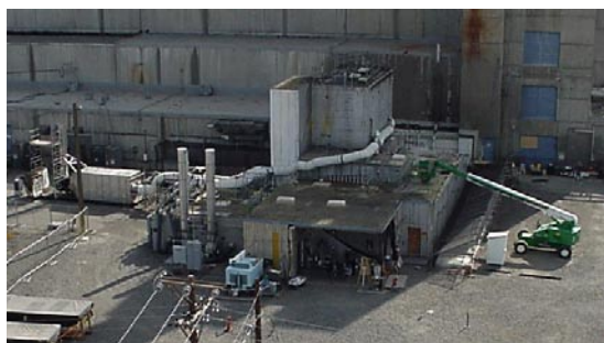
Exhibit 4-1: 233S Prior to Demolition.
