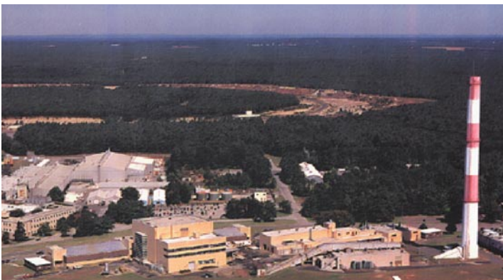
Exhibit 4-17: Brookhaven Graphite Research Reactor at Brookhaven National Laboratory.
