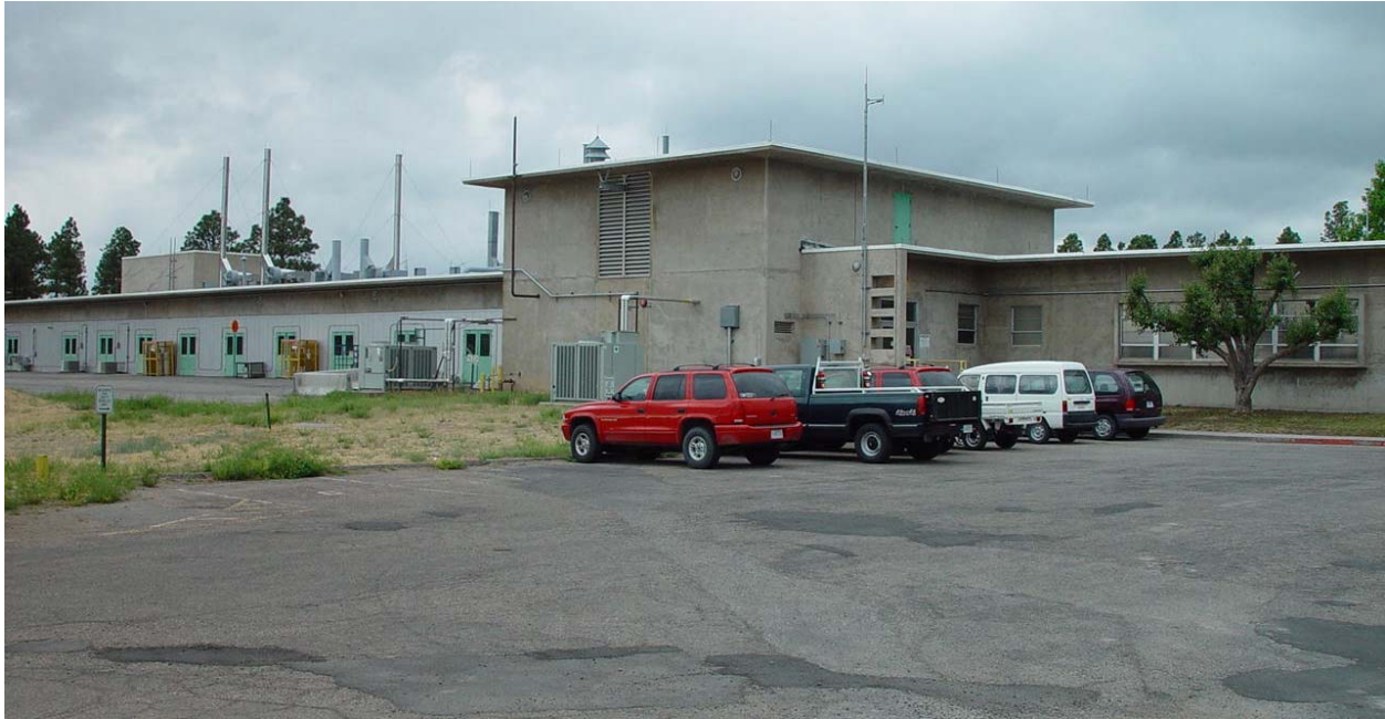
Photo 1. TA-9 Building 21, built in 1952.
