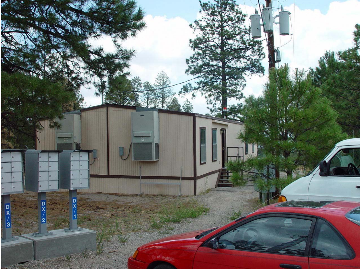
Photo 3. Transportable at TA-69 (Building 2).
