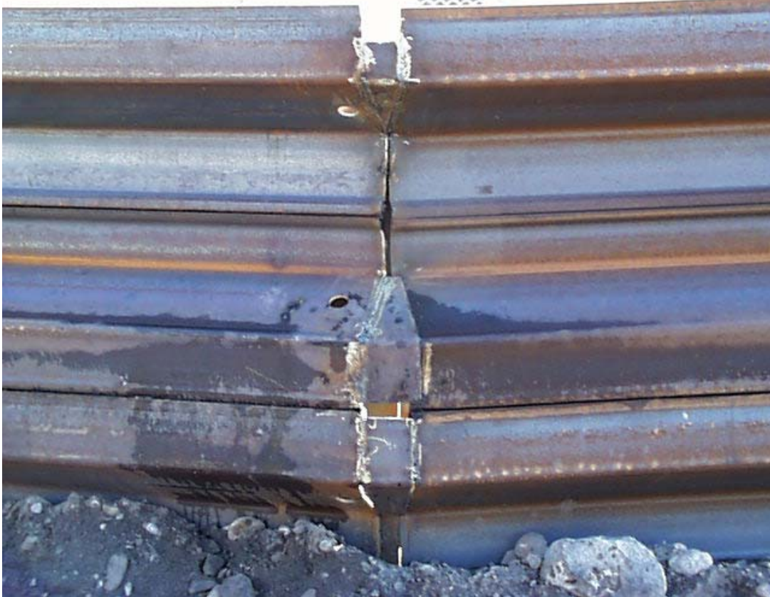
Figure 14. Detail of joined steel panel in steel diversion wall.
