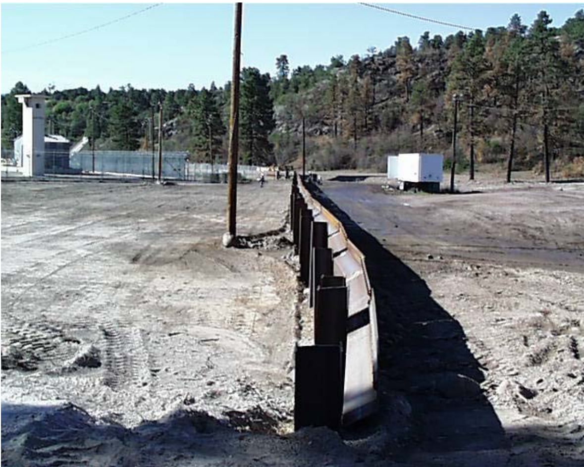
Figure 13. Steel diversion wall at TA-18 under construction.
