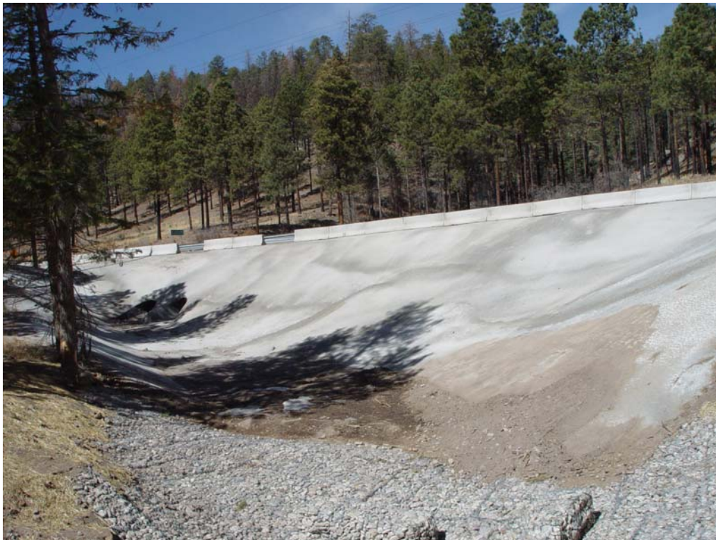
Figure 12. Road reinforcements along SR 501.
