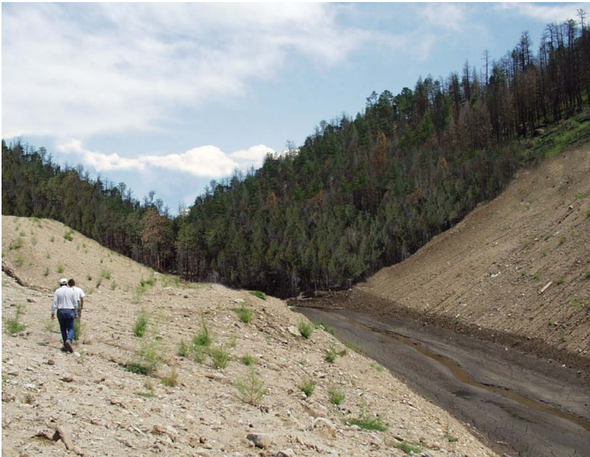
Figure 16. Digitally altered picture of complete removal of the FRS.
