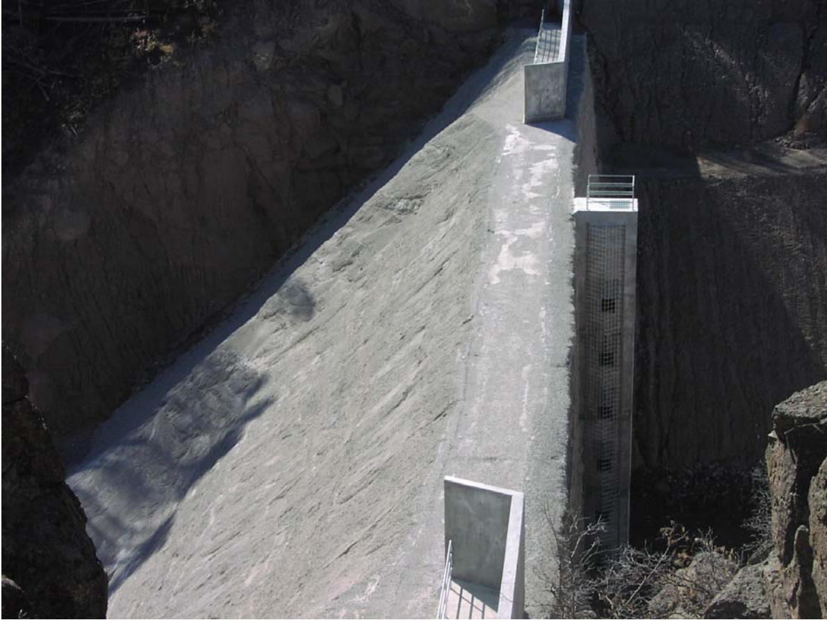
Figure 7. FRS from top of canyon to show 200-ft-wide (60 m) spillway.
