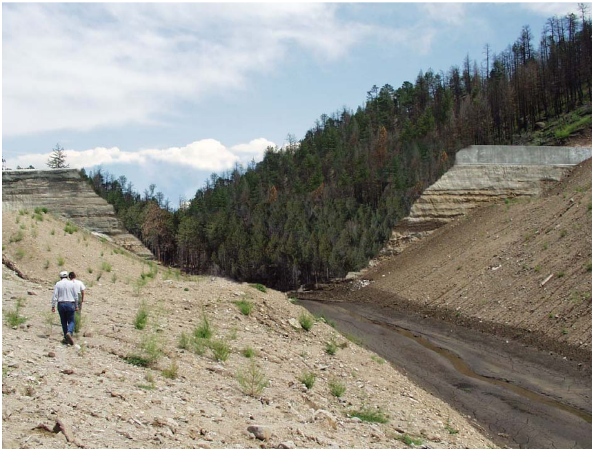
Figure 15. Digitally altered picture of the FRS to show partial removal.
