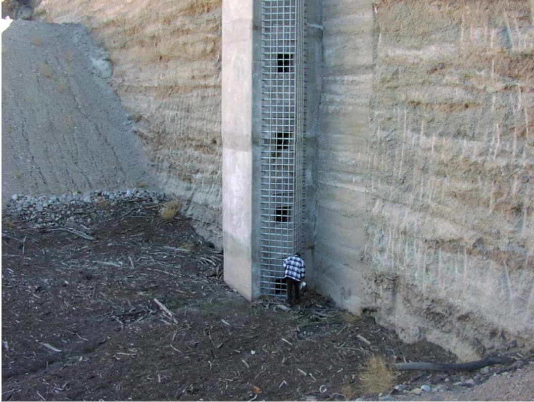
Figure 9. Inlet tower taken from north bank of reservoir to show spacing of openings.
