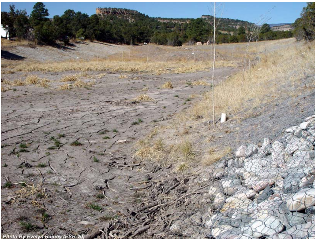
Figure 11. Los Alamos Canyon weir showing detention basin on the left and gabions on the right.
