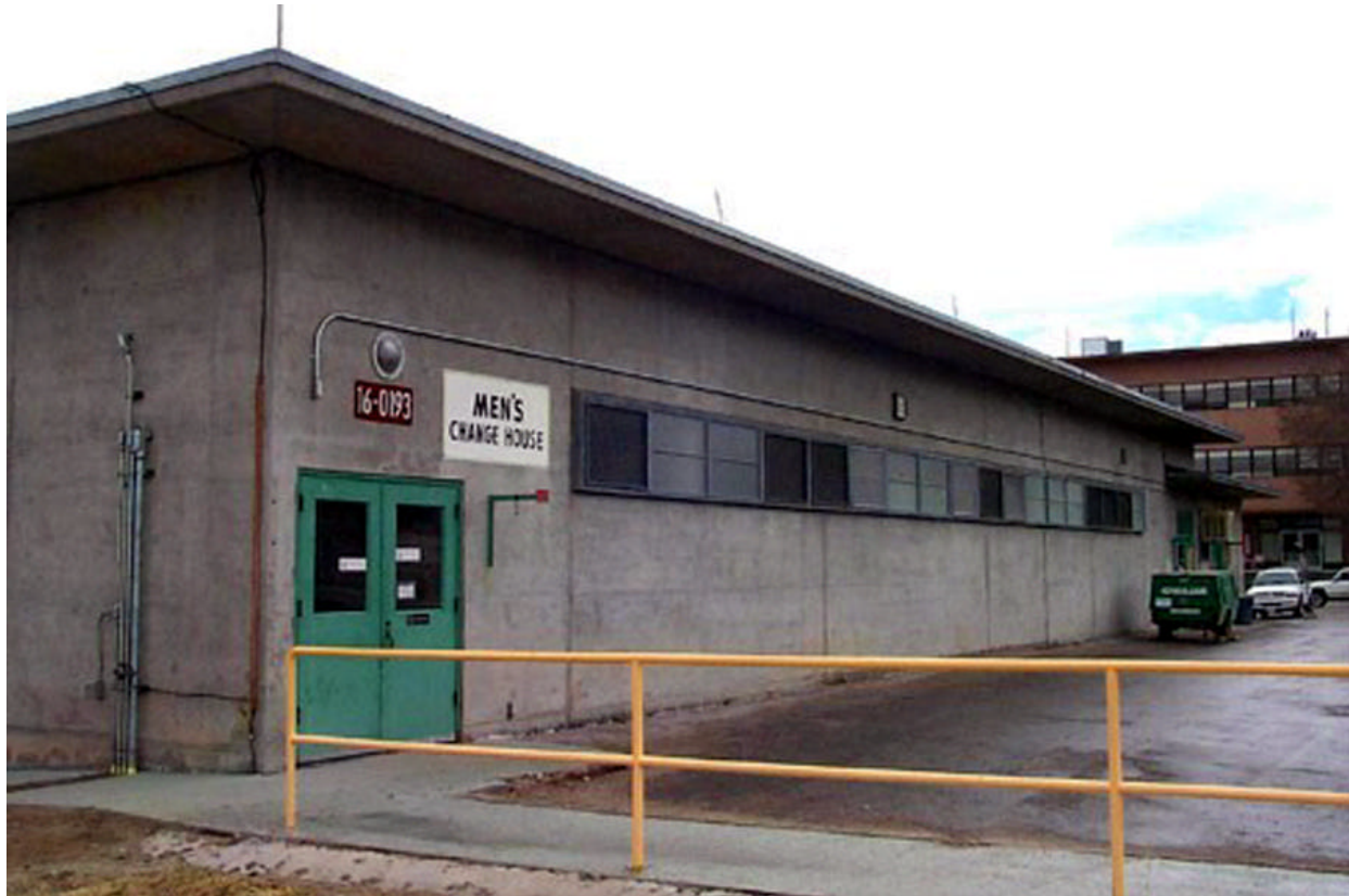
Photo 1. TA-16 Building 193, built in 1952.
