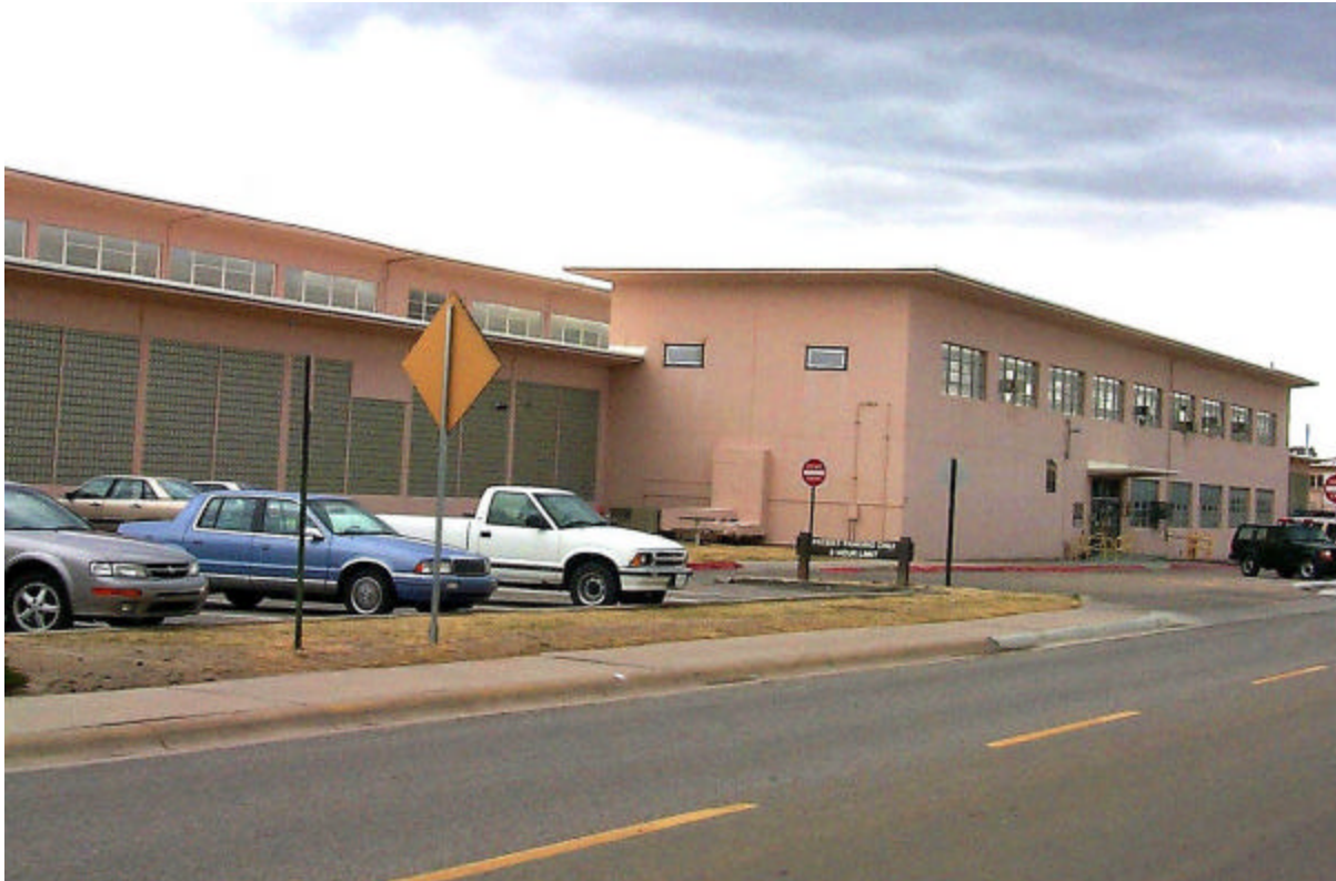
Photo 4. TA-3 Building 39, built in 1953.
