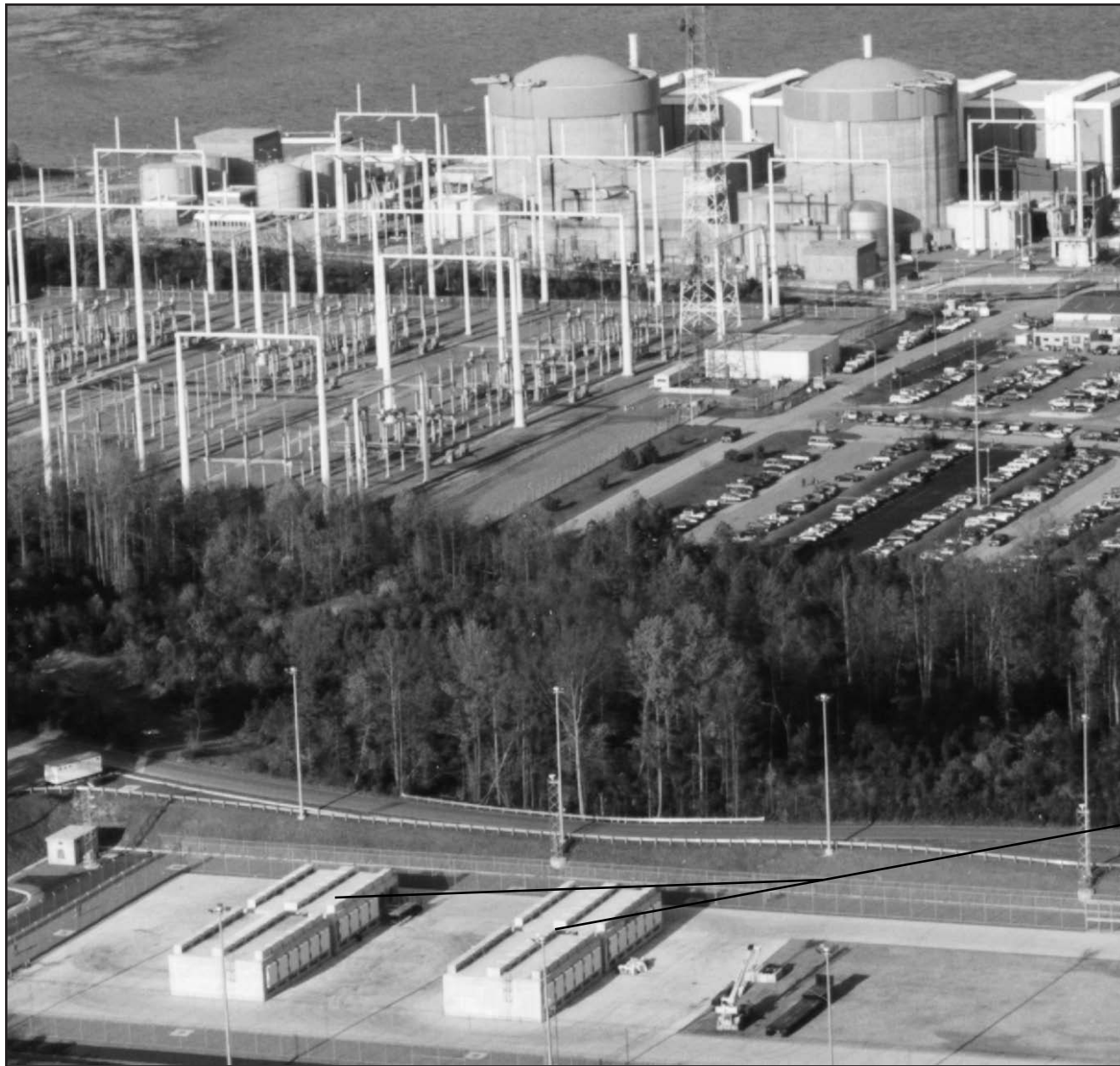
Figure 2-32. Typical independent spent fuel storage installation.
