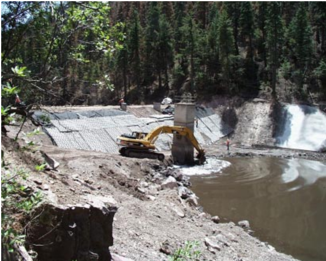
PHOTO 2.15—Reinforcing Los Alamos Reservoir
