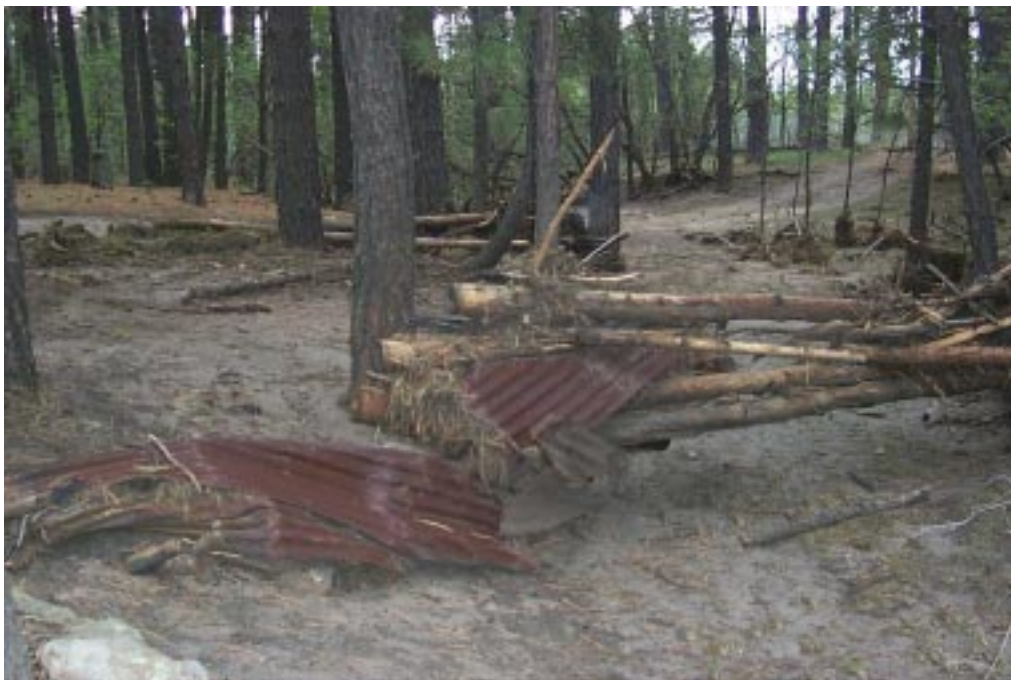
PHOTO 3.6—Anchor Ranch Icehouse after Flooding
