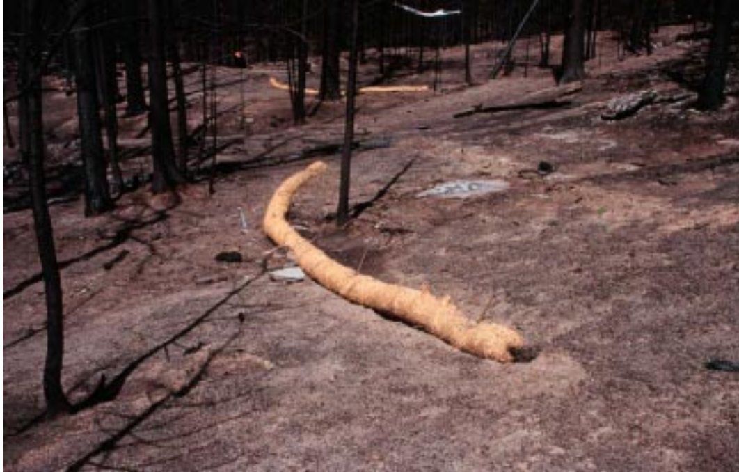
PHOTO 2.12—Straw Wattles in Severely Burned Area
