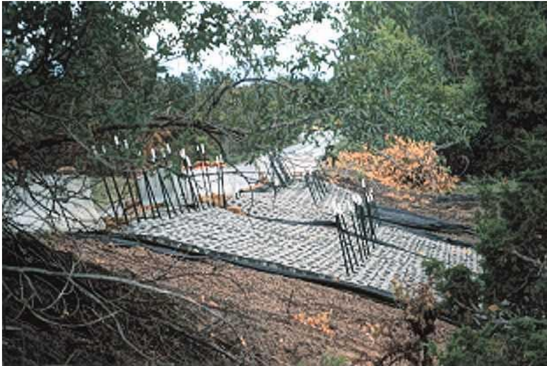
PHOTO 2.18—ACMs Used to Reinforce Road
