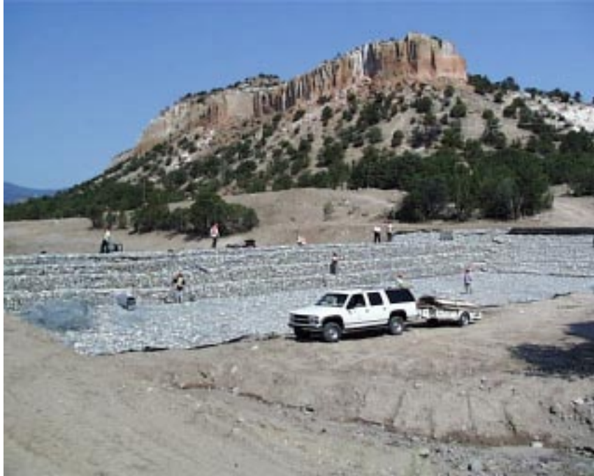
PHOTO 2.17 — Los Alamos Canyon Weir Near SR 4 Under Construction
