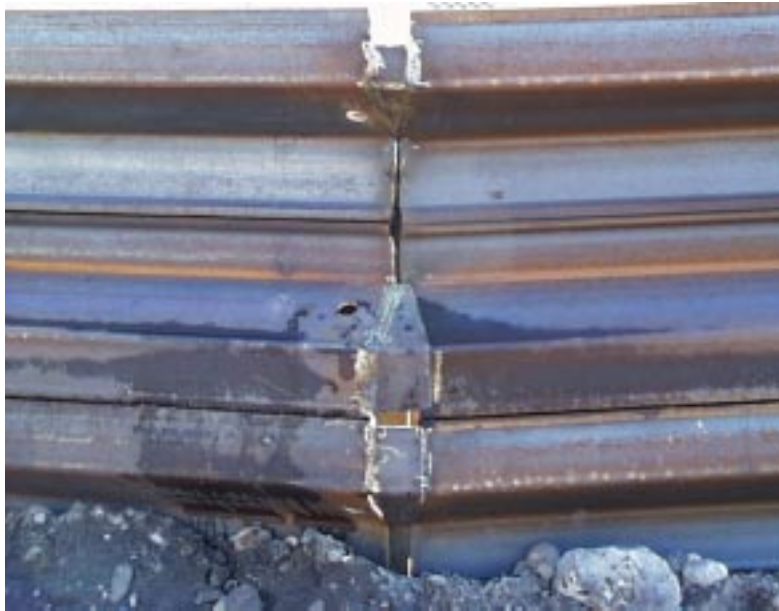
PHOTO 2.21 — Detail of Joined Steel Panel
