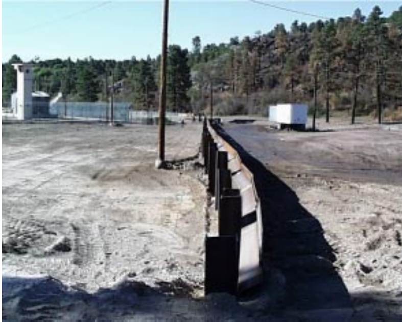
PHOTO 2.20 — Steel Diversion Wall at TA-18 Under Construction
