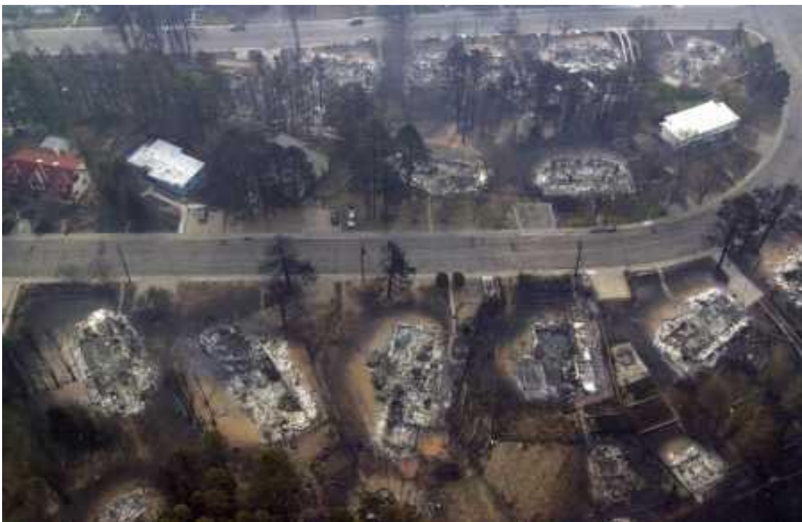
PHOTO 1.2— Cerro Grande Fire Damage to Los Alamos Townsite May 12, 2000
