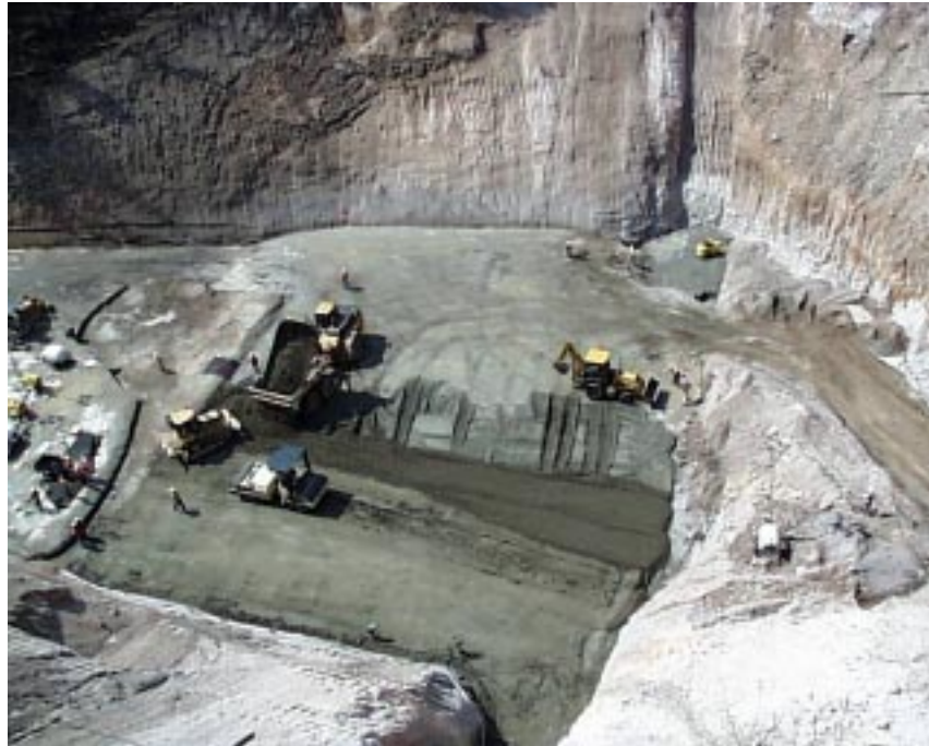
PHOTO 2.19—Base of Flood Retention Structure in Pajarito Canyon Under Construction
