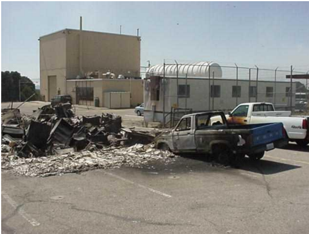
PHOTO 2.5—Burned Transportable at LANL
