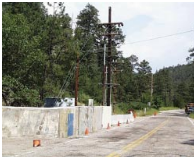
PHOTO 2.13—Storm Water Protection around Utility Pole
