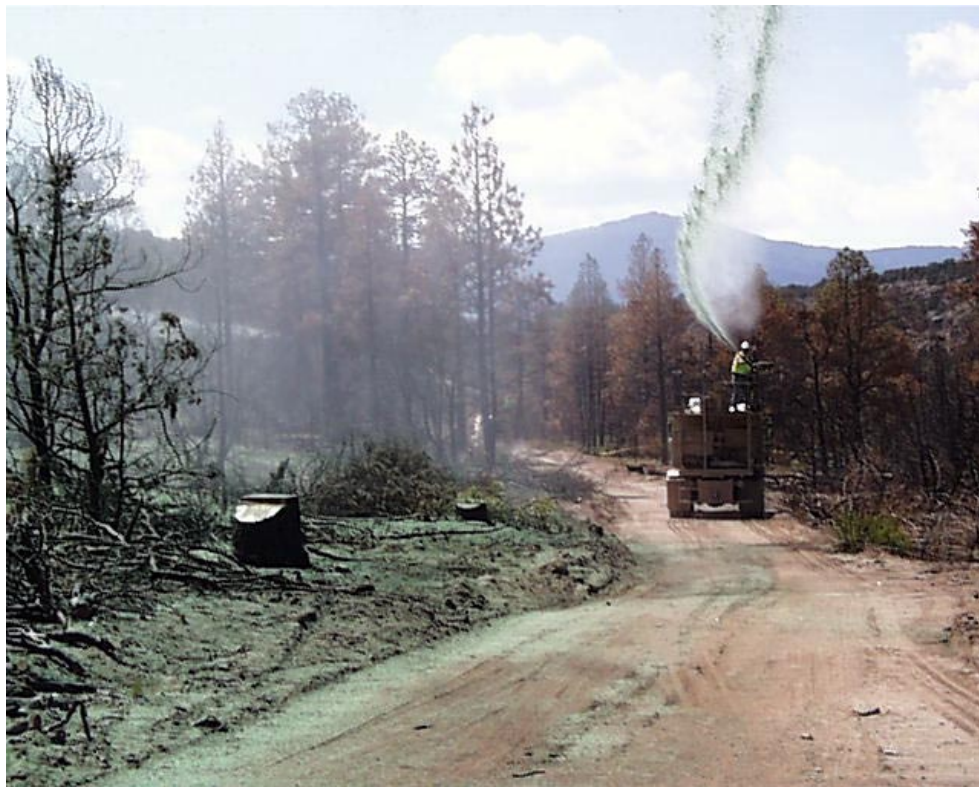
PHOTO 2.9— Spraying Hydromulch
