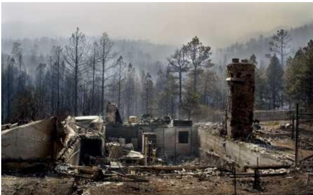
PHOTO 3.1— Burned Residential Unit in Los Alamos Townsite
