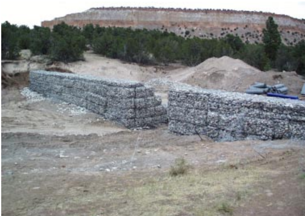
PHOTO 2.14 — Multiple Rock Gabions being Assembled at Los Alamos Canyon Weir
