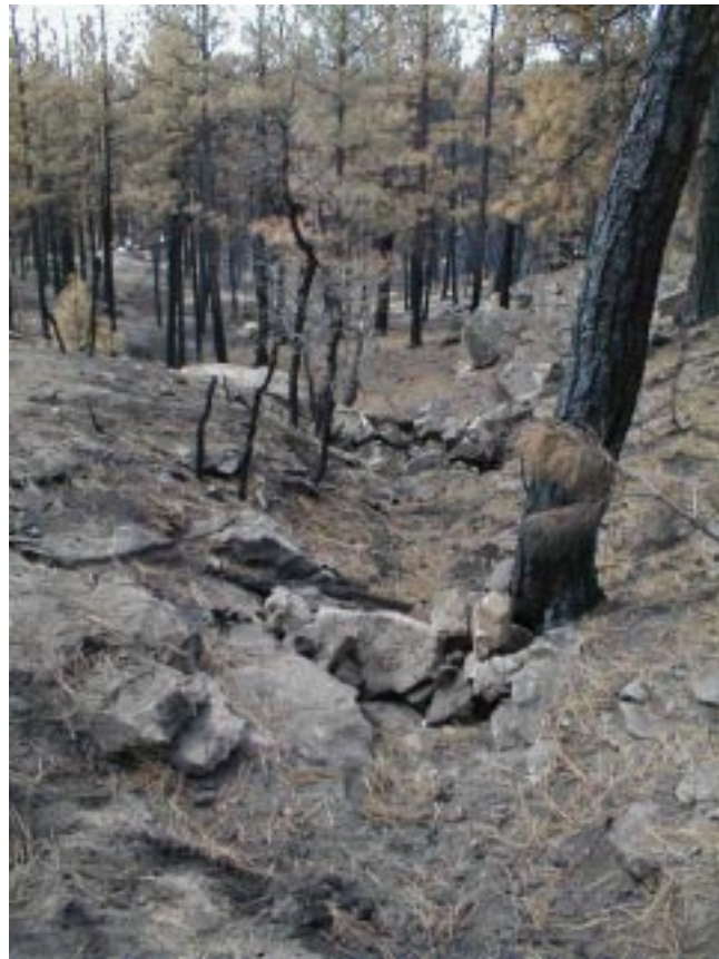
PHOTO 2.11— Rock Check Dam on Burned Slope
