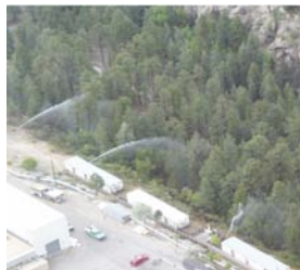
During Cerro Grande fire, trailers at TA-35 were difficult to protect.
