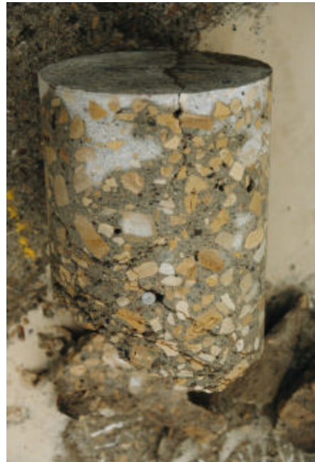
Figures 4.4.3 Close-up photos of joint deterioration from test section 19-3006.
