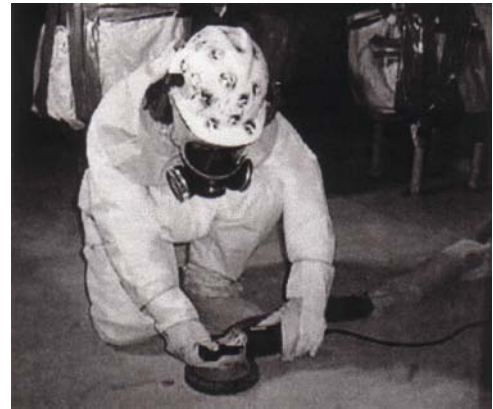
Concrete Grinder in Use
