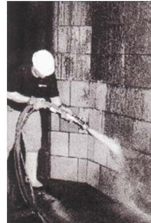
Soft Media Blasting Exhibit 3-28.
