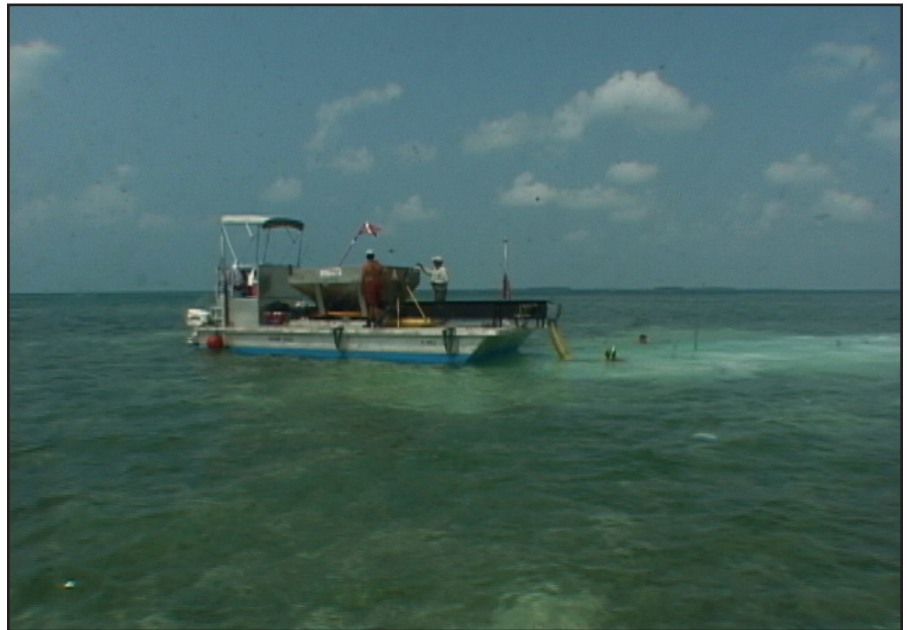
Figure 18.4. Restoration of seagrass beds damaged by a vessel grounding required the addition of gravel substrate at Calda Bank off Key West, Florida. Photo: A. Farner.
