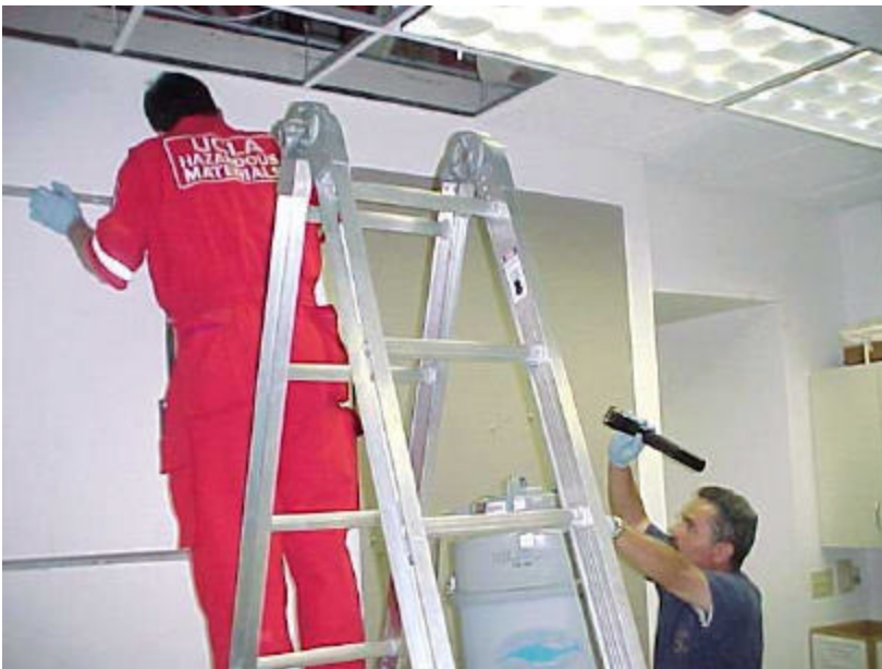
Figure 20 Investigating the extent of damage to ceiling tiles from a mercury spill. (Photograph courtesy of UCLA, Office of Environment, Health & Safety)
