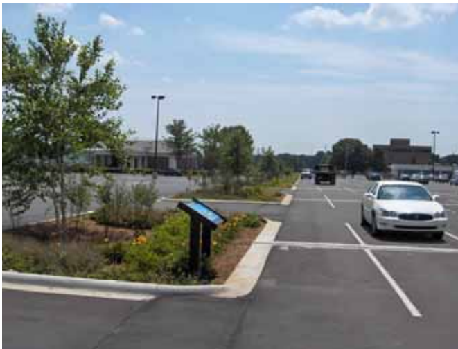
FIGURE 5-27 North Carolina Retrofit Bioretention SCMs. SOURCE: Traver.
