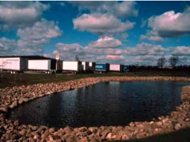
FIGURE 5-3 On-site detention. SOURCE: Tom Schueler.
