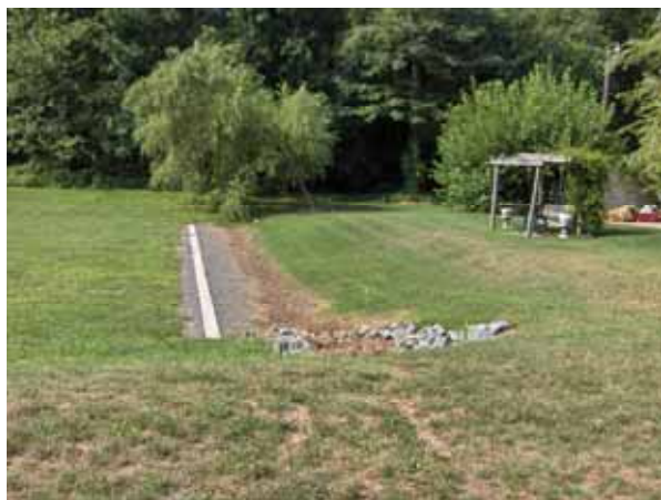
FIGURE 5-11 Level spreader. SOURCE: Robert Traver.
