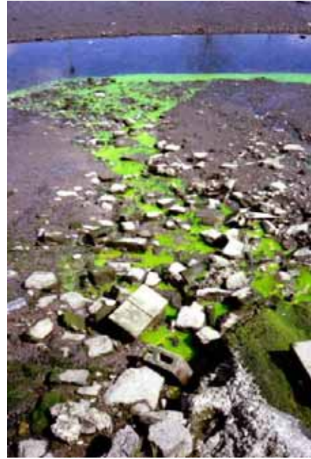
Dye tests to confirm improper sanitary sewage connection to storm drainage system SOURCE: Robert Pitt.
