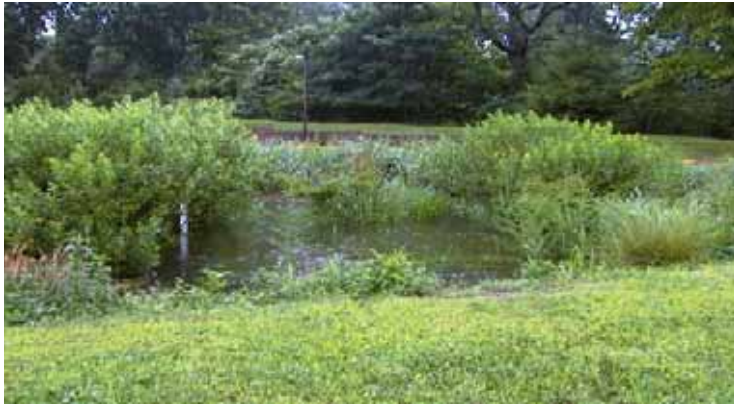
FIGURE 5-19 Retrofit bioinfiltration at Villanova University immediately following a storm event. SOURCE: Robert Traver.
