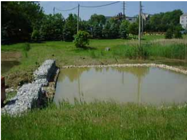
FIGURE 5-44 Villanova University sediment forebay. SOURCE: Reprinted, with permission, from VUSP. Copyright by VUSP002E
