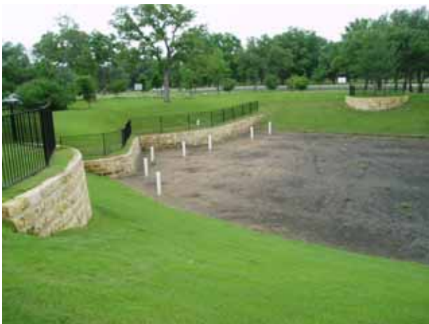
FIGURE 5-45 Austin sand filter. SOURCE: Robert Traver.
