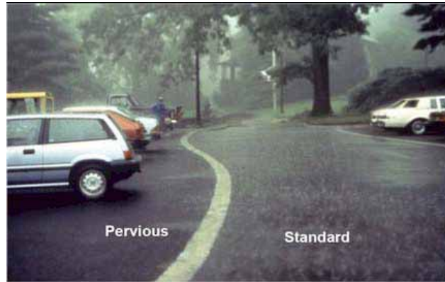
FIGURE 5-29 Porous asphalt. SOURCE: SOURCE: PaDEP.
