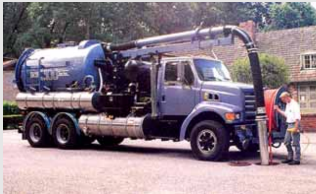
FIGURE 2-3 Catch basin cleaning. Courtesy of Robert Pitt.
