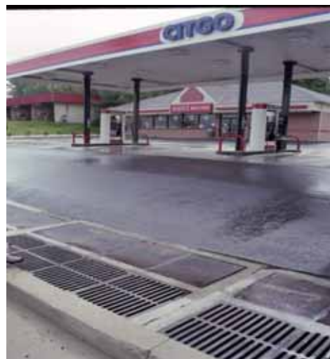
FIGURE 5-46 Delaware sand filter. SOURCE: Tom Schueler.
