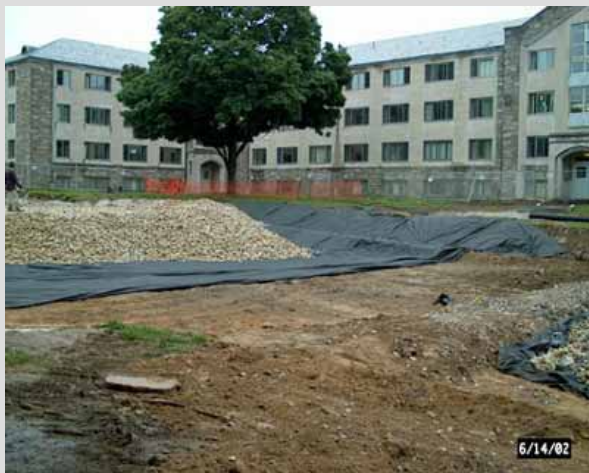
FIGURE 5-34 Infiltration bed under construction. Pervious concrete has functionality and workability similar to that of regular concrete. However, the pervious concrete mix lacks the sand and other fine particles found in regular concrete. This creates a significant amount of void space which allows water to flow relatively unobstructed through the concrete. This site was the first attempt at creating a pervious concrete SCM in the area, and there were construction and material problems. Since that time the industry has matured, and a second site on campus constructed in 2007 has not had any significant difficulties. SOURCE: Reprinted, with permission, from VUSP. Copyright by VUSP.
