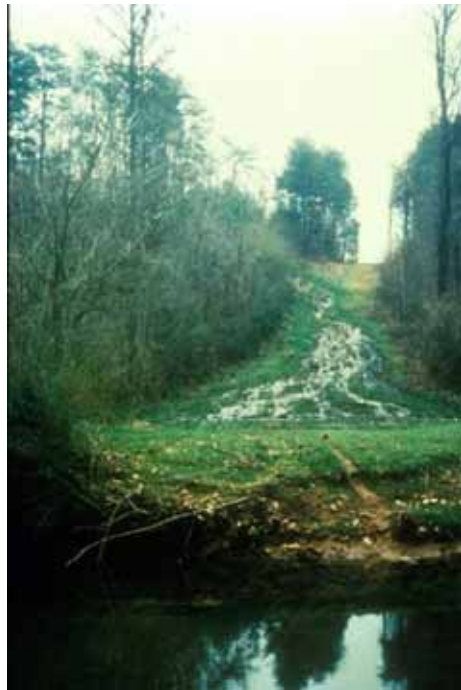
Sewage from clogged system overflowing into storm drainage system. SOURCE: Robert Pitt.
