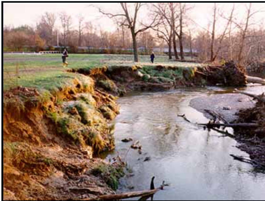
FIGURE 1-5B A destabilized stream in Vermont. SOURCE: Courtesy of Pete LaFlamme, Vermont Department of Environmental Conservation.
