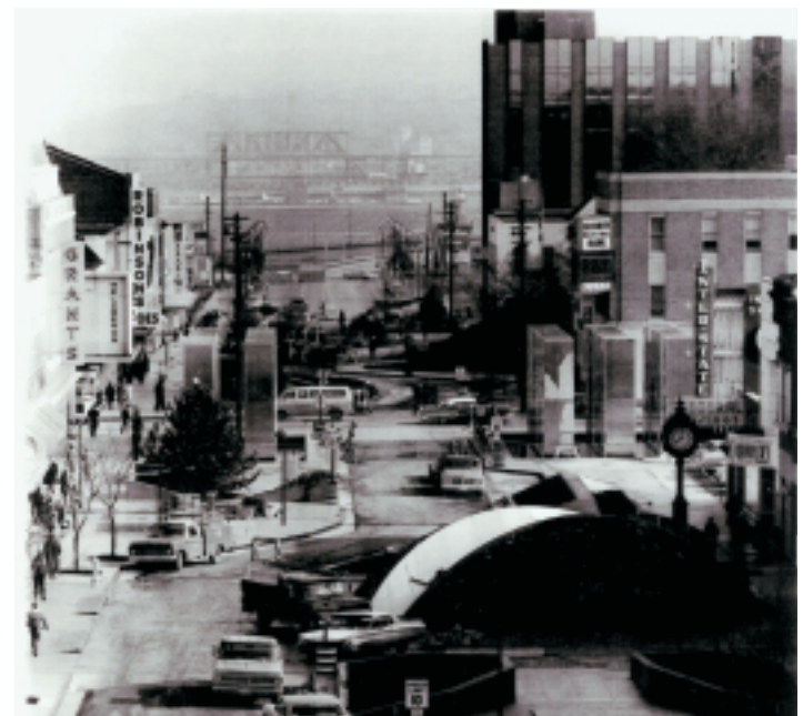
MINNESOTA AVENUE LOOKING EAST c1970 Provided by Wyandotte County Museum
