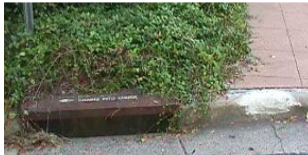
Figure 18: Public education is a vital component to a successful water quality management program. Stormdrain stenciling teaches citizens not to dump pollutants such as motor oil, fertilizers, and trash into stormdrains and ultimately into the nearest waterbody. Other education tools aimed at protecting valuable water resources include brochures, waterway clean-up events, and adopt-a-stream volunteer groups.
