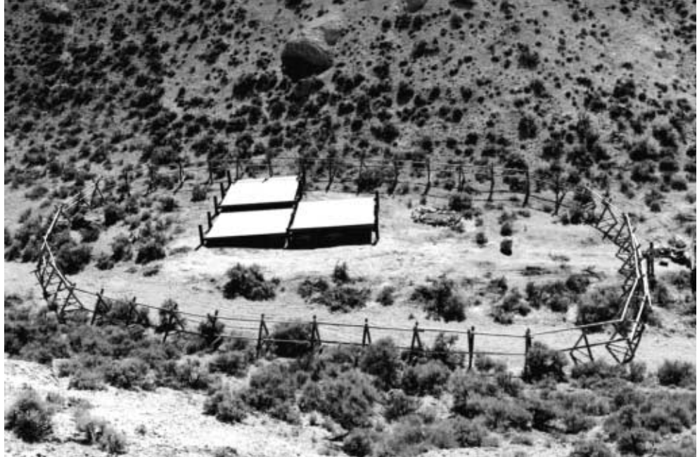
Photo 12. Completed big game guzzler in northern Nevada, consisting of water collecting aprons, buried tanks, drinker surrounded by rocks, and buck-and-rail fence.
