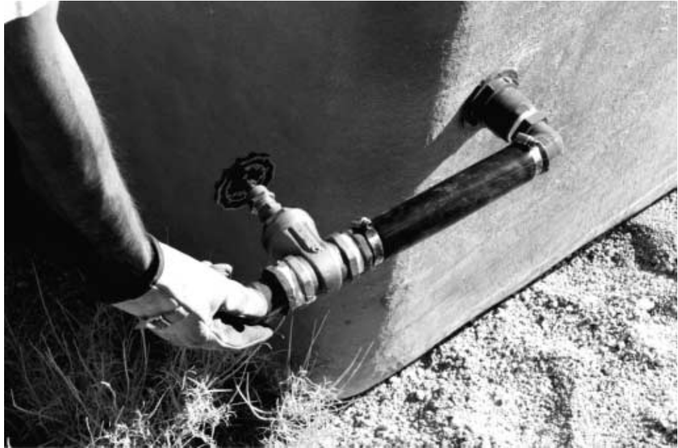
Photo 5. Completed/installed plumbing unit for big game guzzler.
