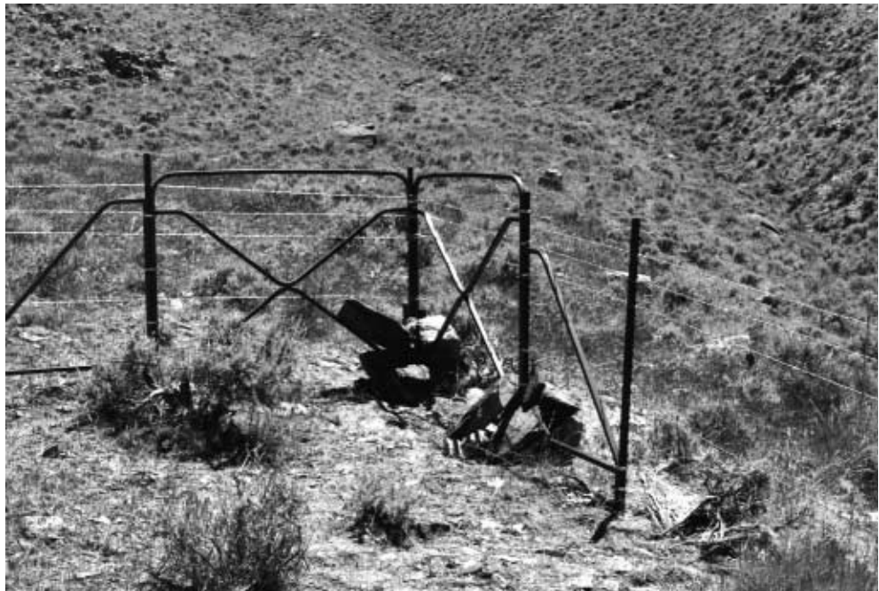
Photo 13. Barbed and smooth wire (bottom strand only) using steel "T" posts and "EZ" panel corners. Rocks (piled or wired on) strengthen the corner.
