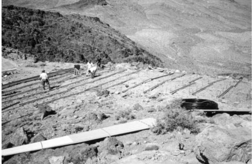
Photo 1. Rows of purlins in place.
