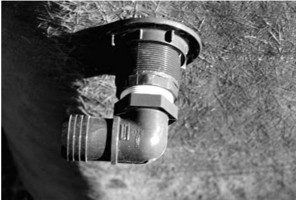
Photo 3. Bottom of fiberglass tank showing bulkhead fastener and 90° MIP-barbed fittings in place.
