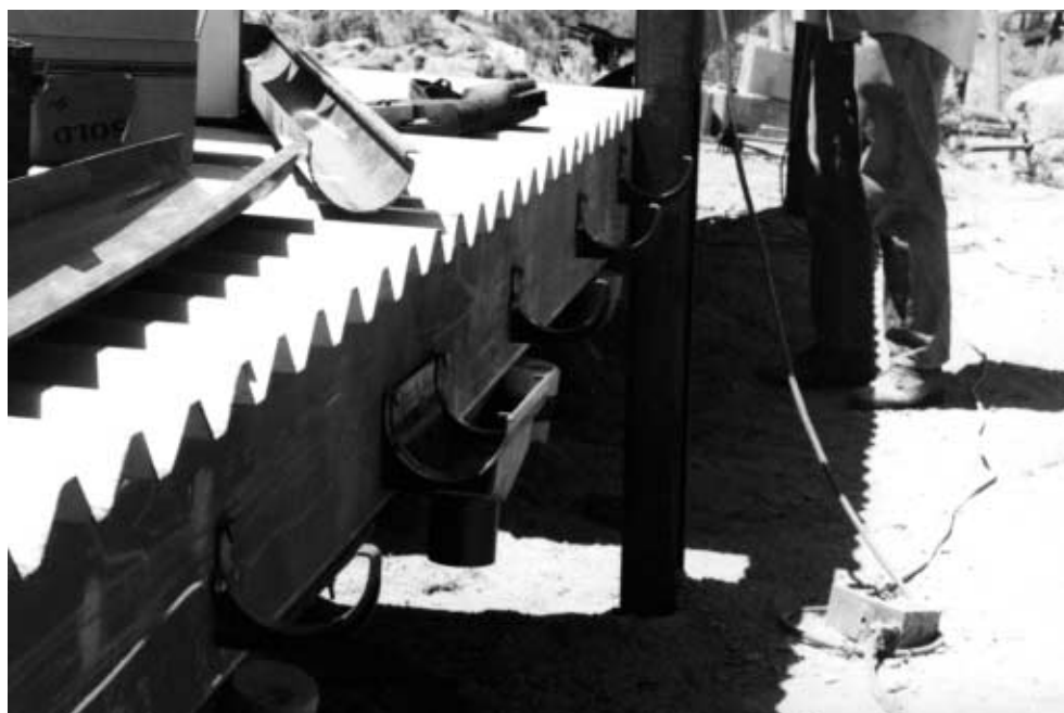
Photo 11. Guzzler gutter details: center drop and PVC gutter brackets are installed; pieces of the snap-in gutter lie on apron.
