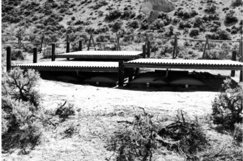
Photo 1. Northern guzzler details. Front aprons share three central uprights; rear apron shares uprights with one front apron. Gutter is in place and connected to tanks. Tops of tanks and sewer and drainpipe (S&D) protecting gate valves are visible.
