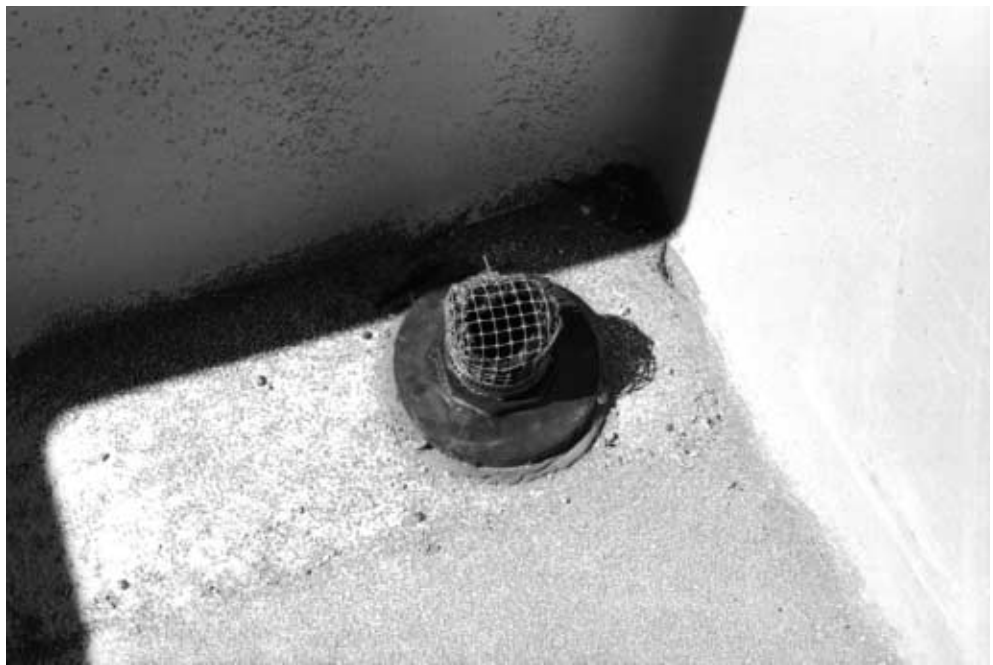
Photo 7. Guzzler riser installed in drinker in self-leveling systems.
