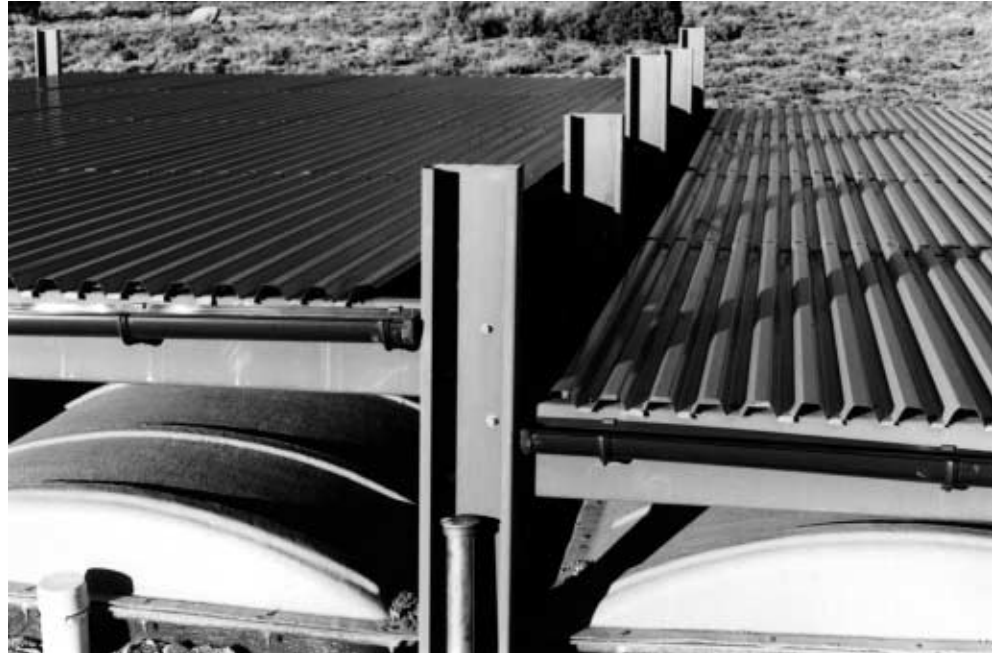
Photo 9. Center uprights with horizontal beams attached, one above the other, resulting in left apron sitting higher.
