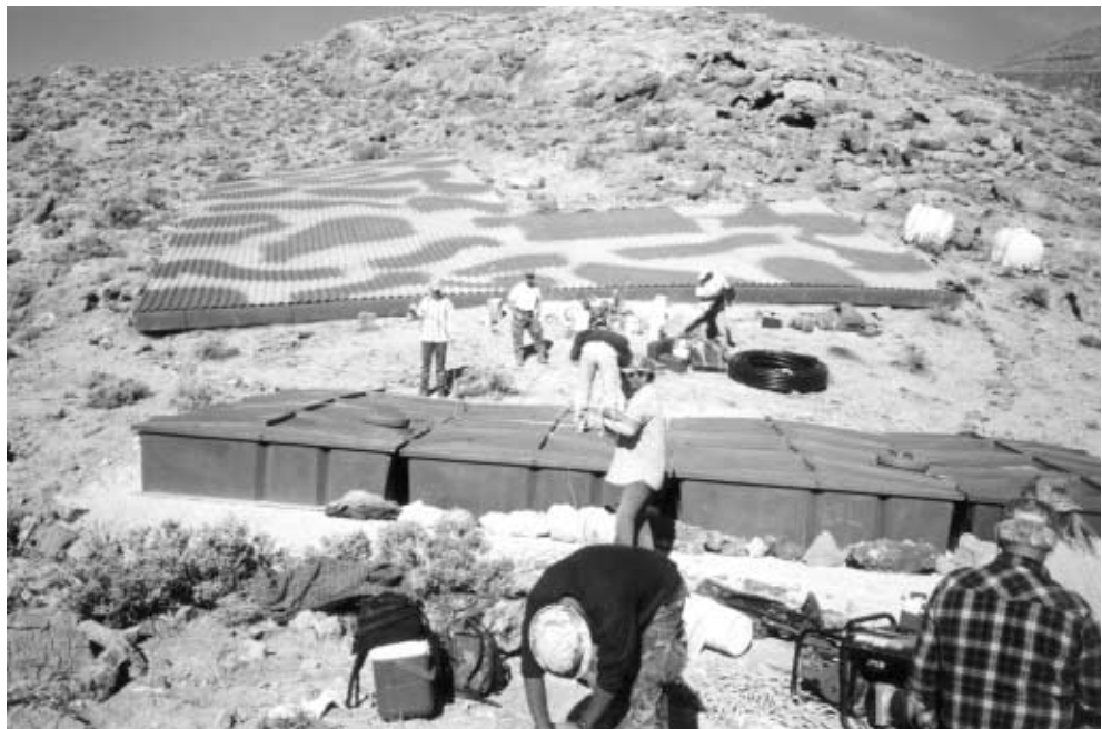
Photo 2. Completed apron in background.
