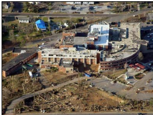
Sumter Regional Hospital devastated by March 1st tornado.
