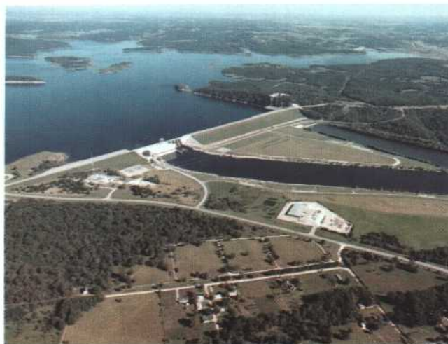
Flood storage in the Missouri River Basin reservoirs, such as the Harry S Truman Lake, reduced the average daily flow near St. Louis for July 1993 by over 211,000 ft 3 /s. (U.S. Army Corps of Engineers.)
