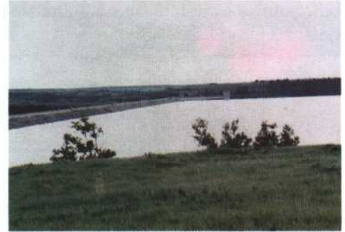
Tuttle Creek Lake rose over 60 feet above multipurpose level into its surcharge pool.
