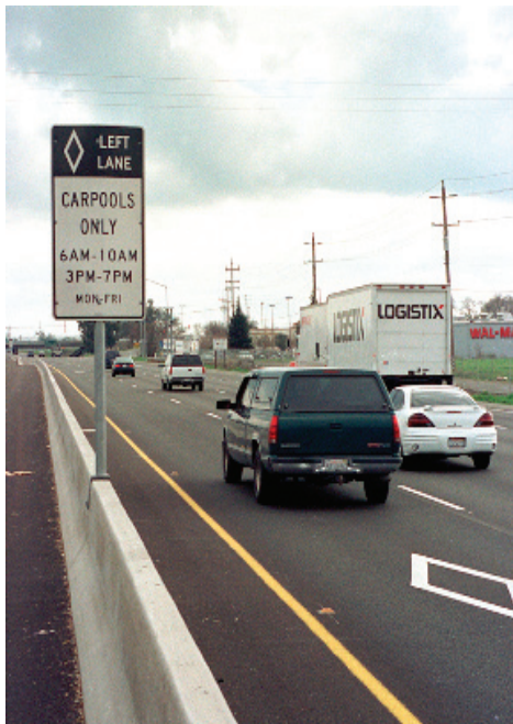
Caltrans has constructed 1,268 miles of high occupancy vehicle (HOV) or carpool lanes statewide.
