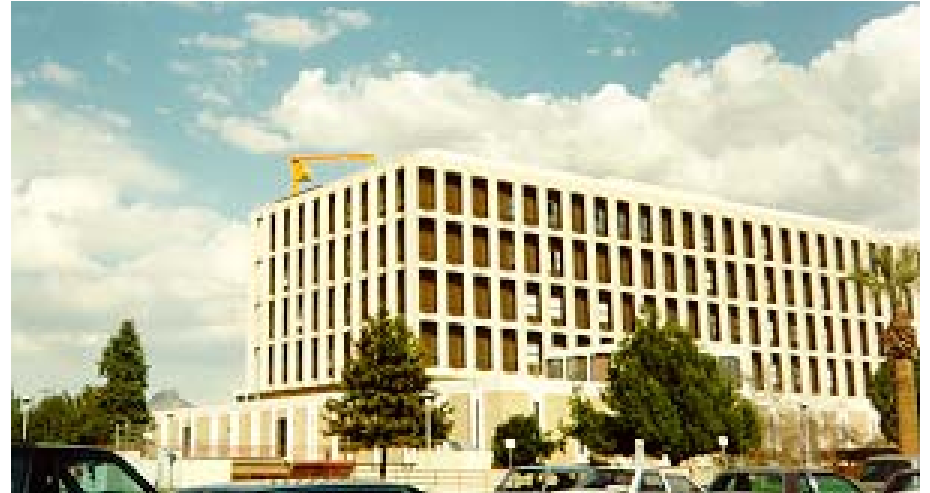
The IHS Phoenix Indian Medical Center, in Phoenix, Arizona was constructed in 1970.
