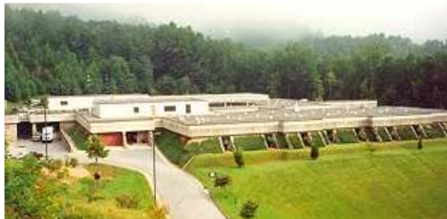
The IHS Hospital in Cherokee, North Carolina (below), was designed with solar panels in the roof to increase energy efficiency.
