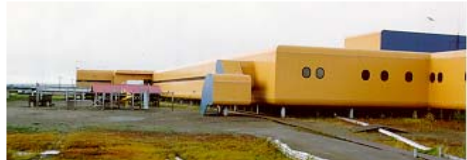
The Yukon Kuskokwim Delta Regional Hospital in Bethel, Alaska, (above) received an architectural award for its design.
