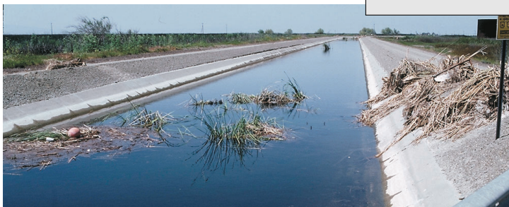
In 1996, a 45-kilometer section of the San Luis Drain was re-opened to transport agricultural drainage to the San Joaquin River and ultimately to the San Francisco Bay/Delta Estuary. The drain is posted with a state health advisory because of selenium.
