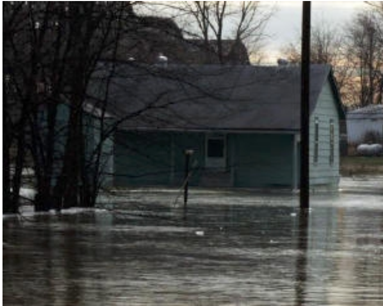
Photo of a flooded area on Pearl Street in Metropolis, IL. Metropolis is one of the largest cities on the lower Ohio River not protected by a levee or floodwall. Photo courtesy of Beau Dodson.
