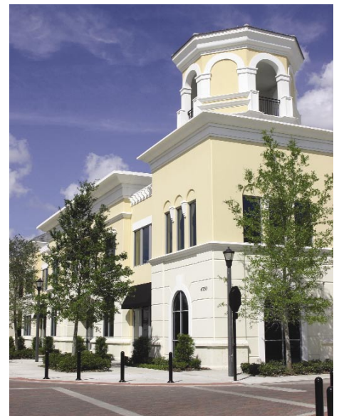
Attractive office space is a critical part of the Baldwin Park project.
