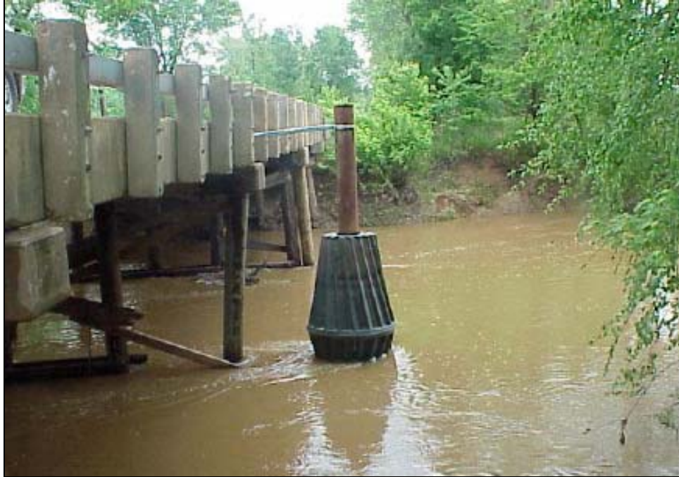
Figure 5.46. Close up of a debris sweeper installed on the South Fork Obion River in Tennessee.
