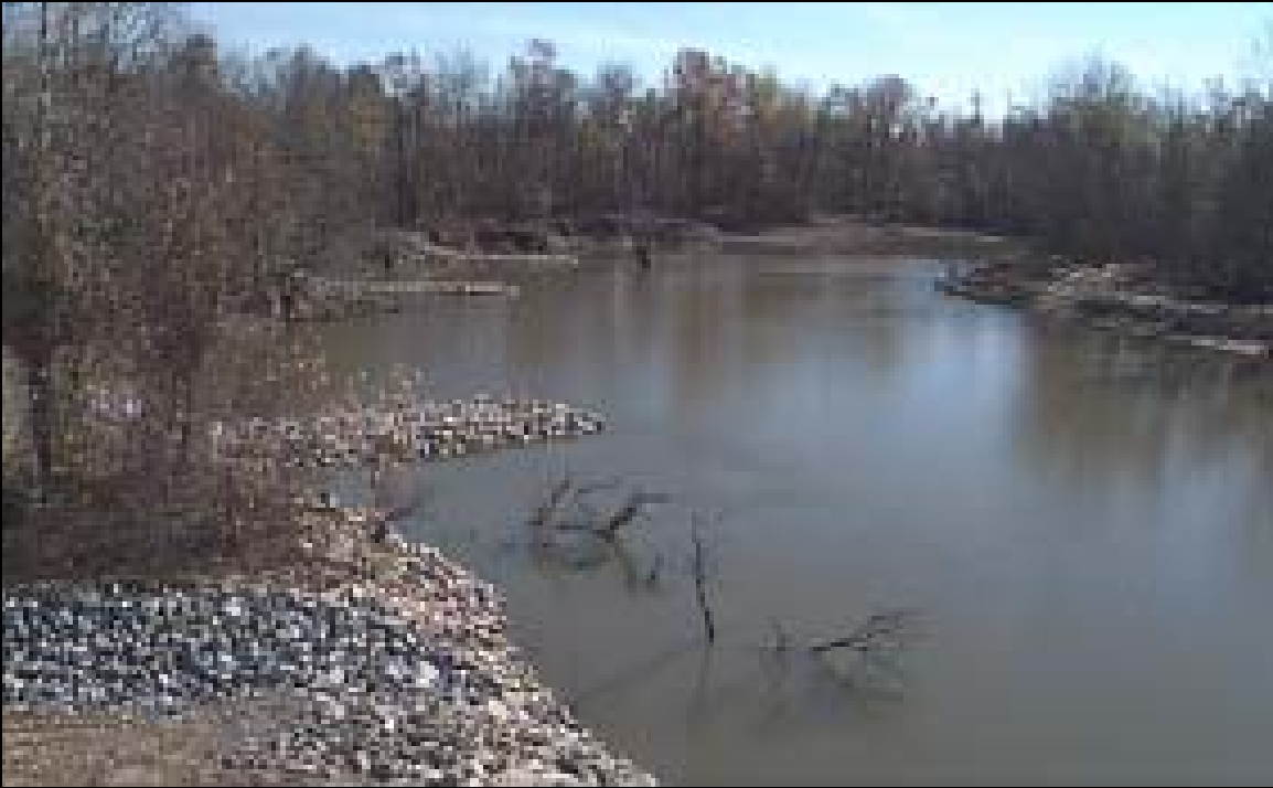
Figure 5.41. Bendway wiers on outer bank of Hatchie River looking upstream (TDOT).
