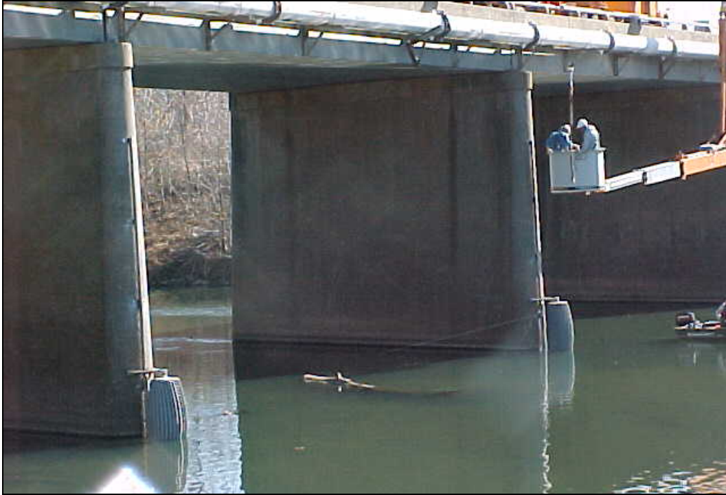
Figure 5.44. Debris sweeper being installed on a bridge over Staunton River in Altavista, Virginia.
