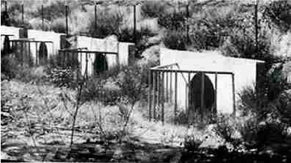
Figure 5.4. Steel debris deflectors installed at entrances to a battery of culverts.
