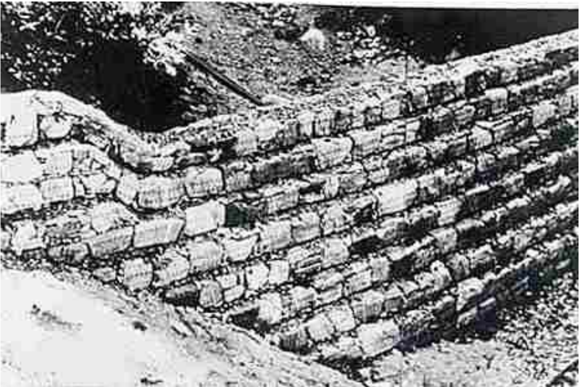
Figure 5.37. Gabion debris dam.
