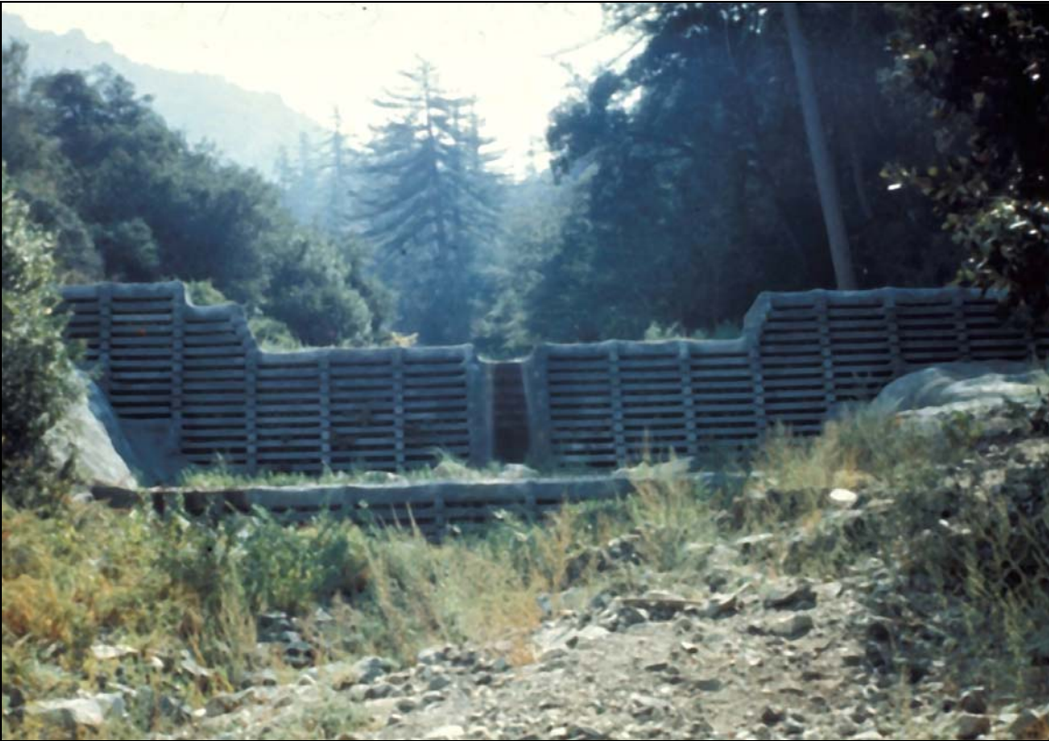
Figure 5.39. Debris dam of precast concrete sections fabricated to enable placement in interlocking fashion.
