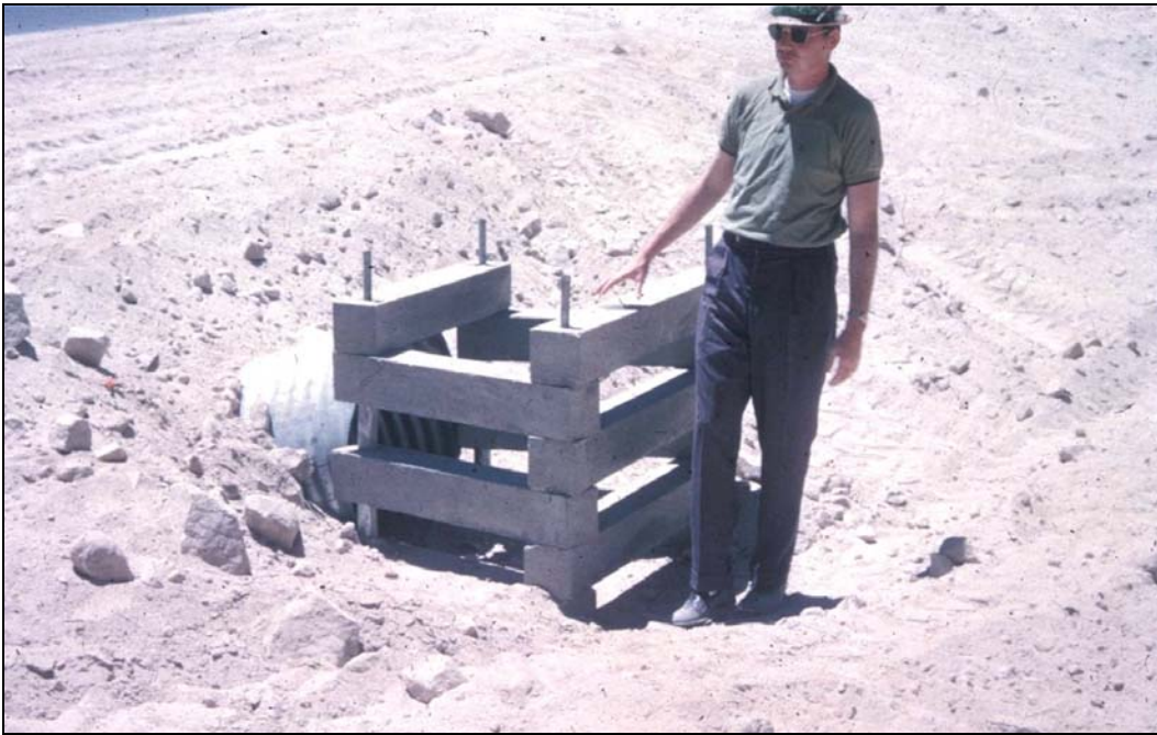
Figure 5.27. Arid region debris crib of precast concrete sections and metal dowels.
