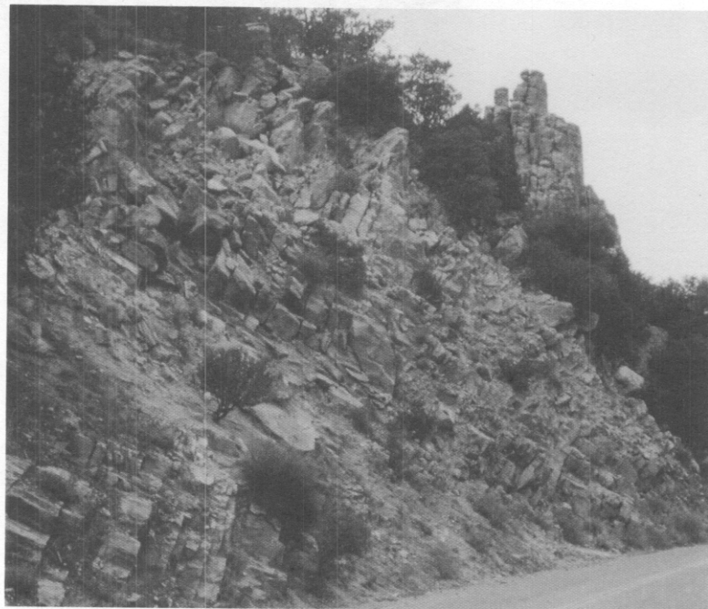
Figure 5.3 Determine the vertical height of the slope not the slope length. This 73-foot high slope is scored 25 points.
