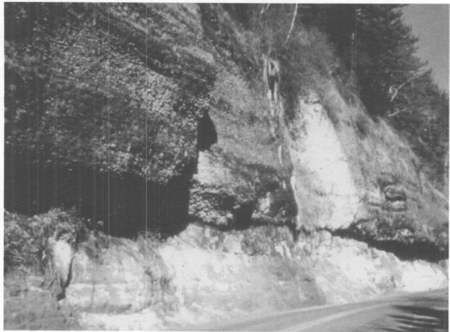
Figure 3.4 Overhanging slope caused by differential erosion.
