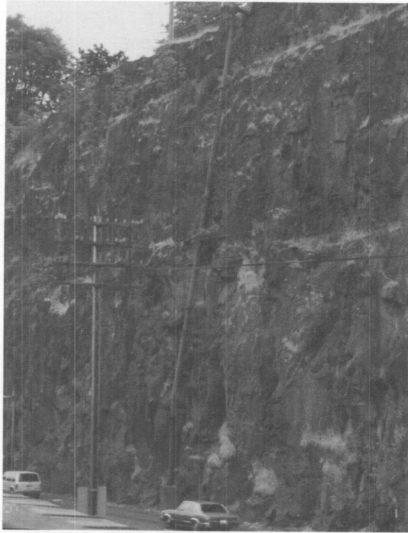
Figure 5.2 When the slope is nearly vertical and there is access to the top, the height can be measured with a tape.
