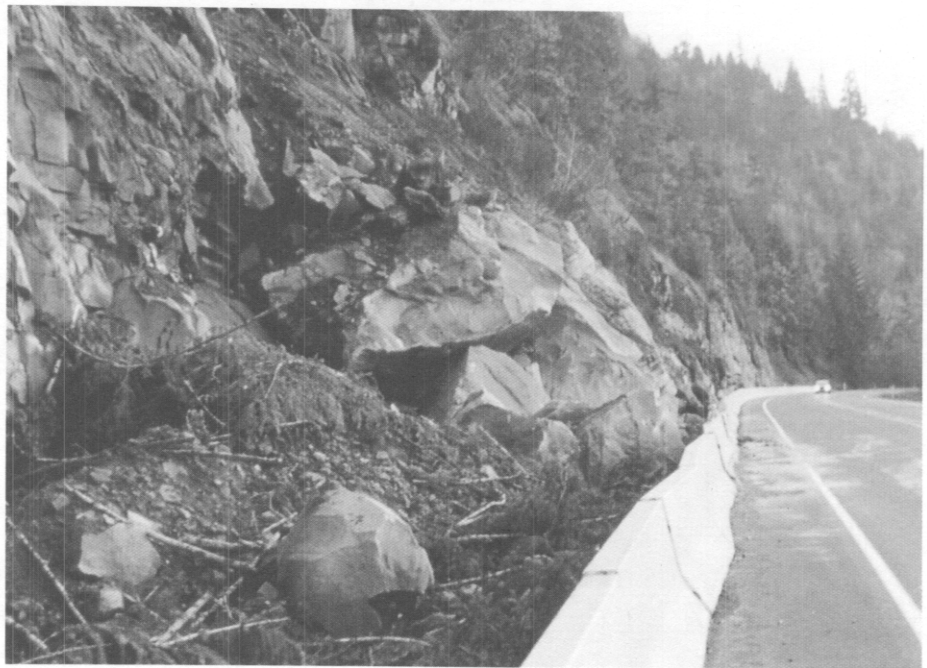
Figure 8.2: When the large block fell, some of the debris reached the roadway. Future rockfalls, which will be smaller, should be retained in the ditch.
