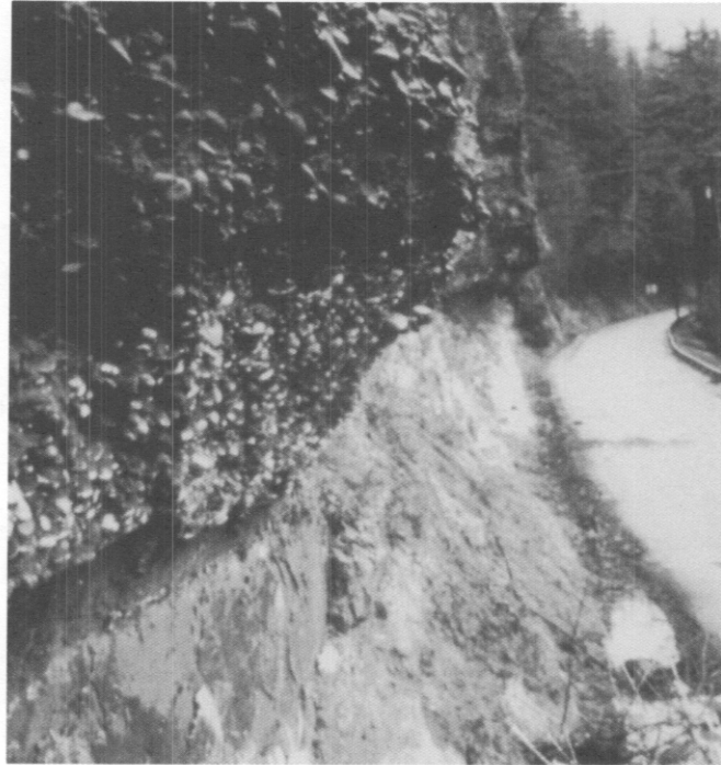
Figure 5.11 The measured sight distance is 330 feet.
