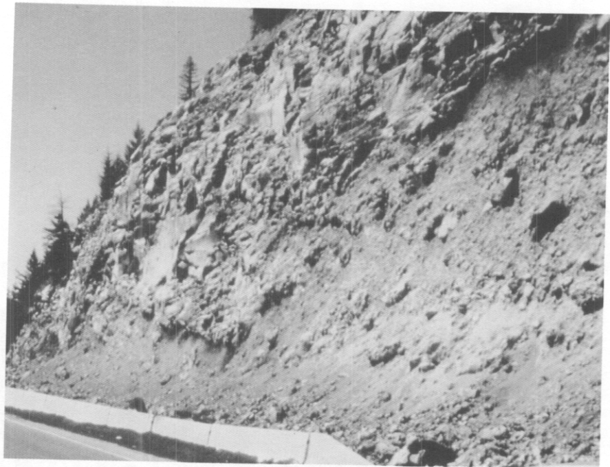
Figure 5.27 The cinders at the base of the slope are strongly affected by freeze/thaw cycles and rain. The difference is extreme.
