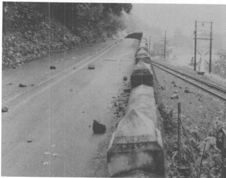
Figure 5.10 Vertical curves can also restrict sight distance.
