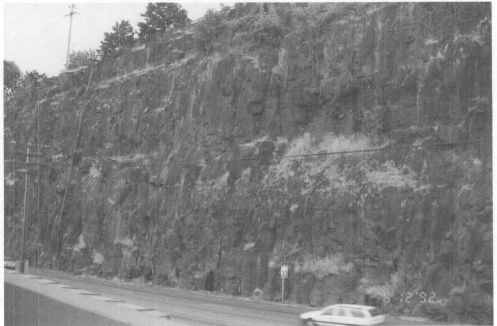
Figure 10.1 Overview of site 2. Slope height?
