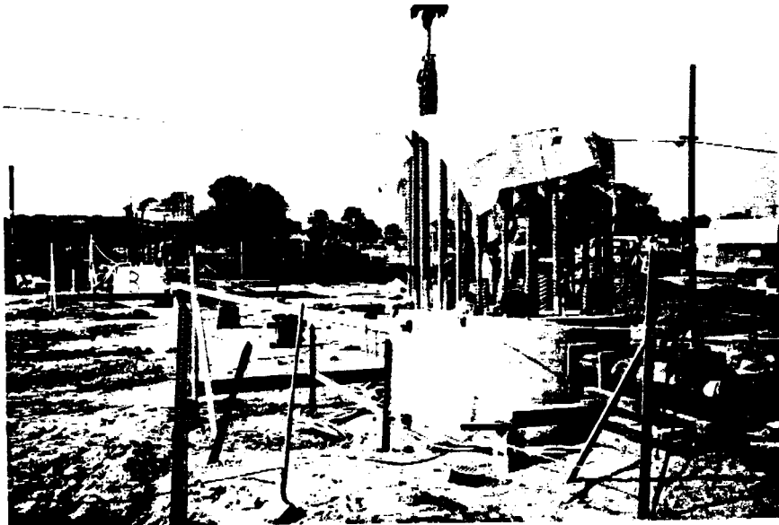
Figure 6.1. Testing of a drilled shaft under lateral loading, Los Angeles.
