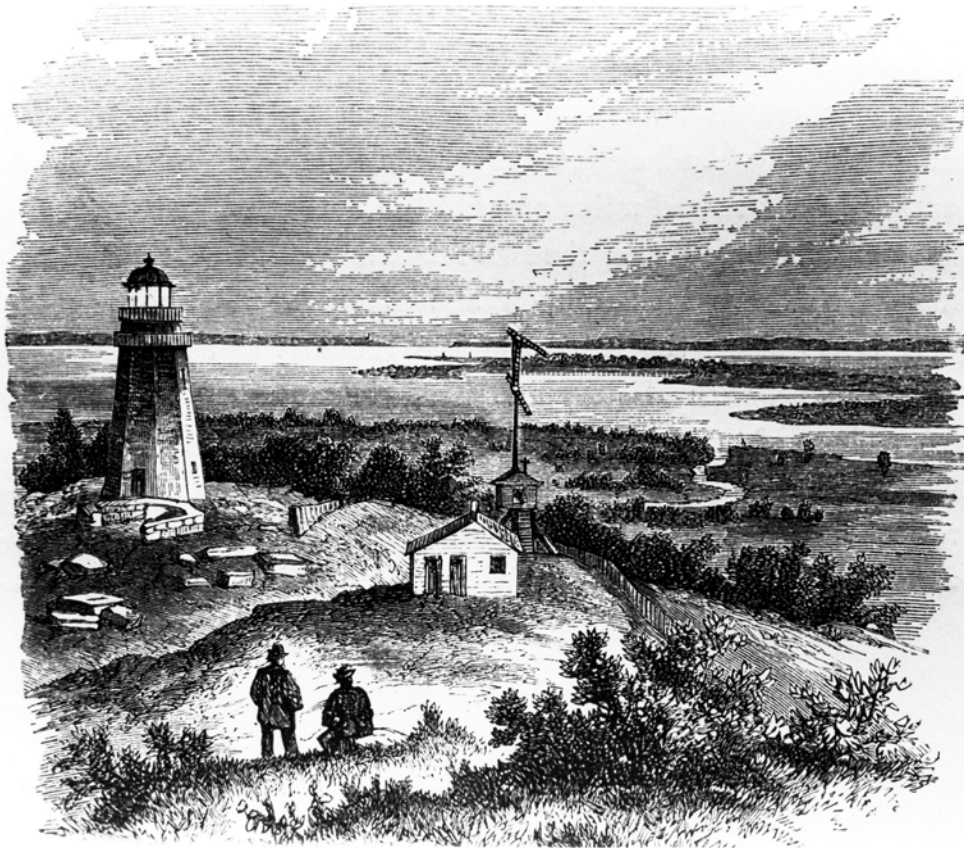
Figure 16: Historic sketch of Navesink Light Station depicting 1862 north tower and foundation of 1828 north tower; also in sketch is semaphore tower.
