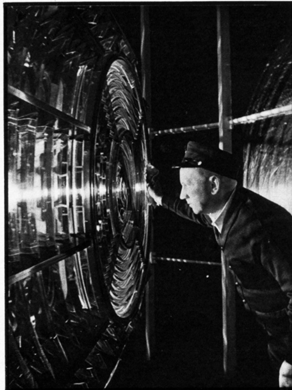
9,000,000 CANDLEPOWER: THE LENS AT NAVESINK Keeper Murphy L. Rockette of the Navesink Light station at the land end of Sandy Hook, New Jersey, inspects his bulbs, looks for dust flecks on his prisms. His lens, a bivalve worth $20,000, is turned six times each minute in a pot of mercury by electric current supplied by the Jersey Central Power & Light Co.
