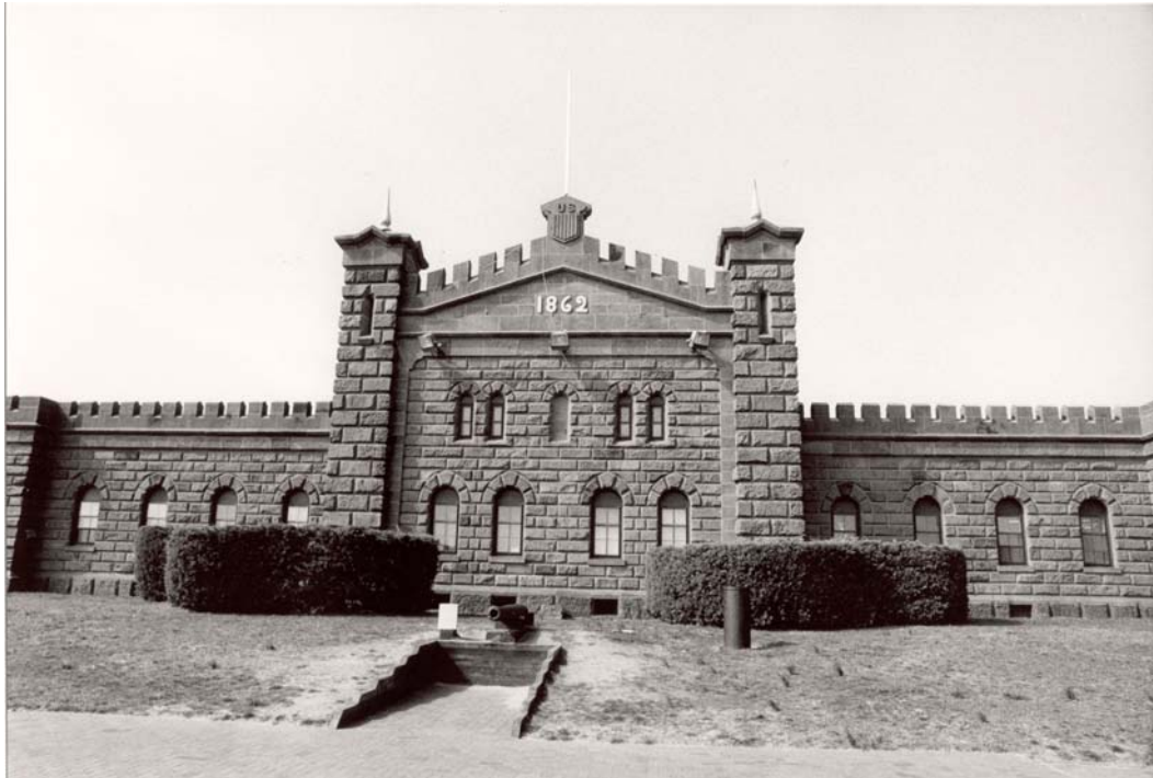
Figure 3: Navesink Light Station Keepers' Quarters (east elevation)
