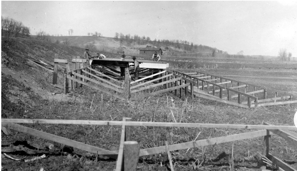
Fig. 33. Constructing the troughs at Fairport Biological Station. Courtesy Fairport Fish Hatchery, Iowa Department of Natural Resources.
