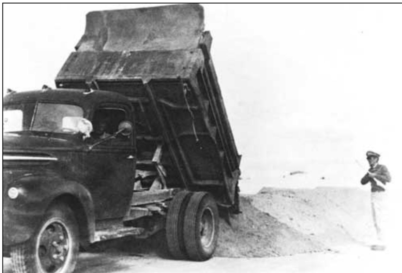
Figure 12. Pouring gypsum for road shoulder construction (1930s). (Courtesy White Sands National Monument)
