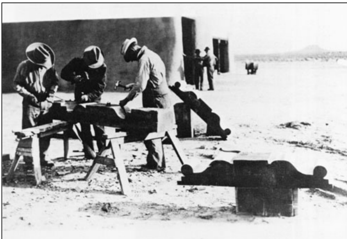
Figure 16. Hispanic workers making corbels for Visitors Center (1930s). (Courtesy White Sands National Monument)
