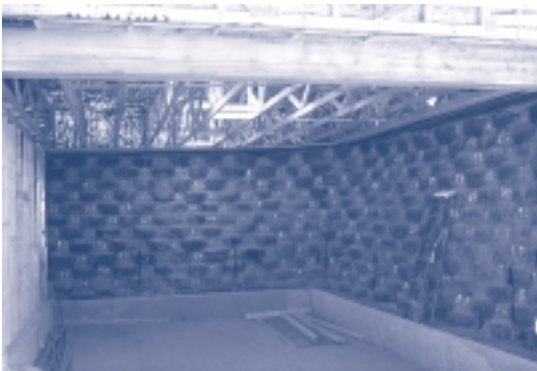
Tires and dirt are used to construct the conference room walls.
