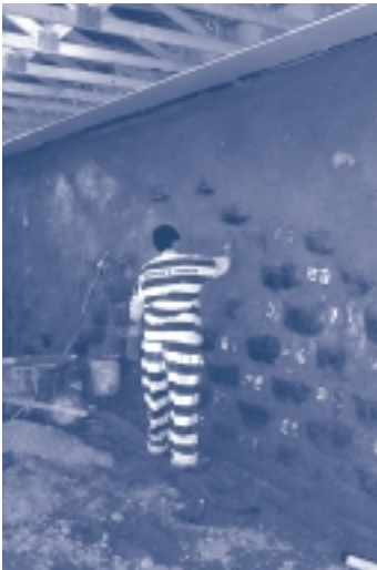
Worker preparing for placement of the final layer of dirt.
