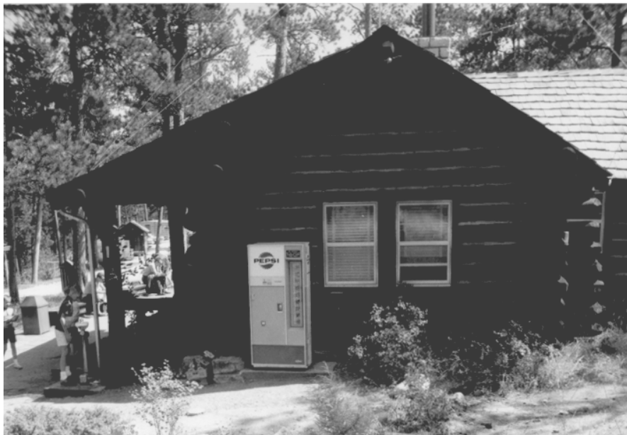
Figure 17. "Ranger Station and Pop Machine, Fassbender, 1965." By this time the cabin had been modernized with aluminum storm windows, a pop machine, and a drinking fountain. Jewel Cave NM photo archives, Neg. No. 2286.
