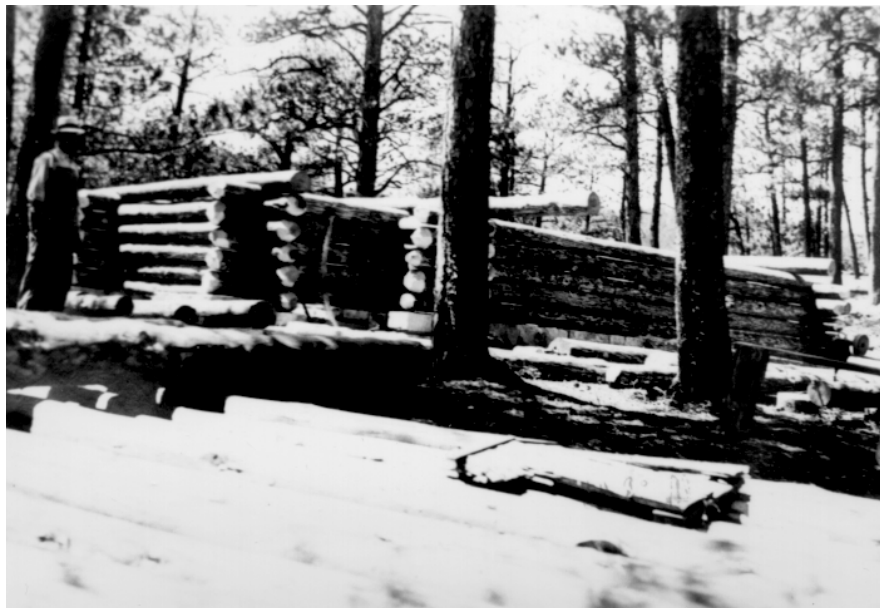
Figure 1. "July 2, 1935, Stevens Studio, Hot Springs, S.D." View to the northwest showing first few log courses. Jewel Cave NP photo archives, Neg. No. 789.
