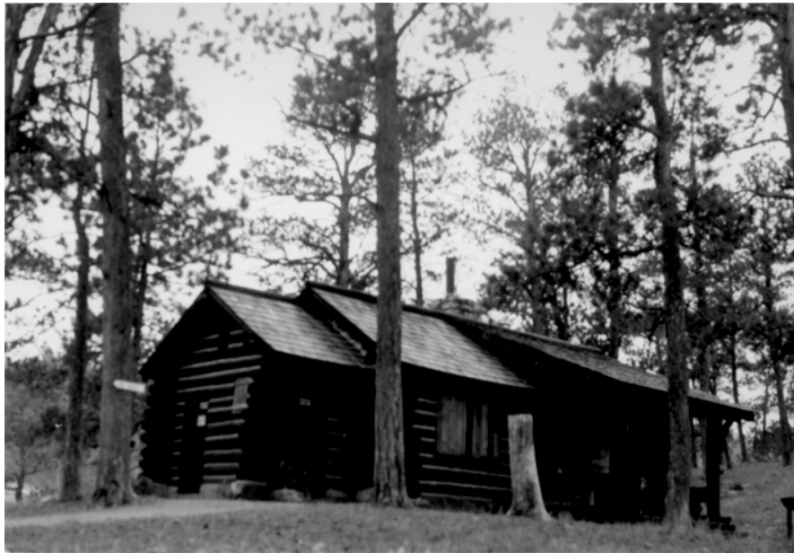
Figure 16. "Ranger Station," circa 1952. In this image the board shutters in place on the windows, and a clay flue pipe extends from the chimney. Jewel Cave NM photo archives, Neg. No. 2616.
