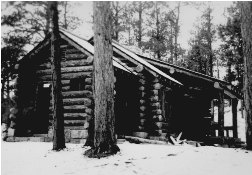
Figure 5. The Ranger Cabin during construction, 1935, view to the northwest. By the time of this winter photo some of the windows had been installed. Jewel Cave NM photo archives, Neg. No. 2626.
