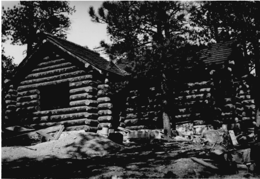
Figure 4. “Ranger Station, Serran, 1935.” In this view to the northeast the roof and chimney are complete, but the windows have not been installed. Jewel Cave NM photo archives, Neg. No. 2618.
