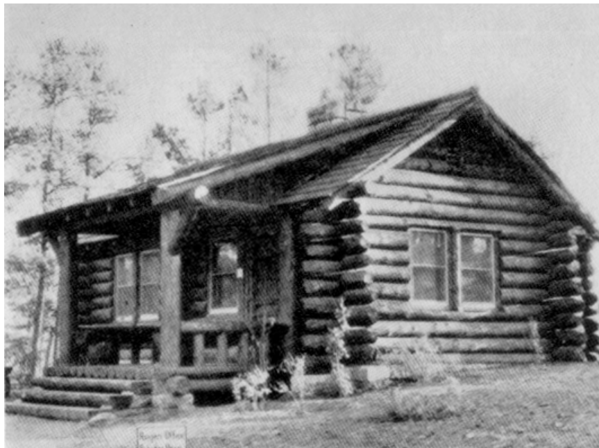
Figure 9. "Ranger's Station, Jewel Cave National Monument." Note the sign in the foreground indicating that the cabin was in use at the time. Log joints had yet to be daubed. From Albert Good, Park and Recreation Structures , Boulder, Colorado: Greybooks, 1990, (1938), 84.
