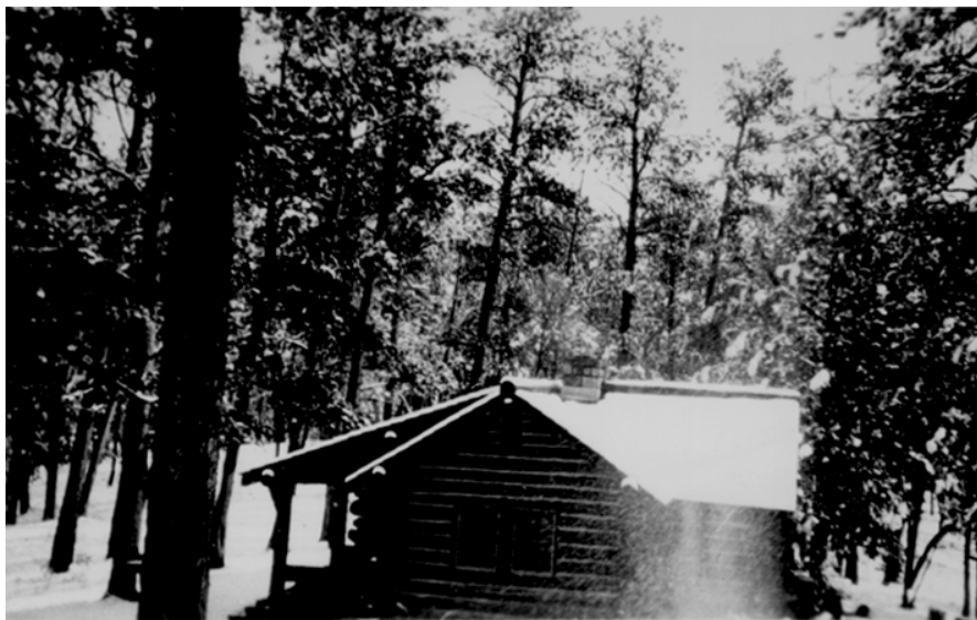
Figure 11. "Taken from the well (water fountain), circa 1942." This is the first image showing log joint daubing. Smoke from the chimney indicates the building was occupied during the winter. Jewel Cave NM photo archives.
