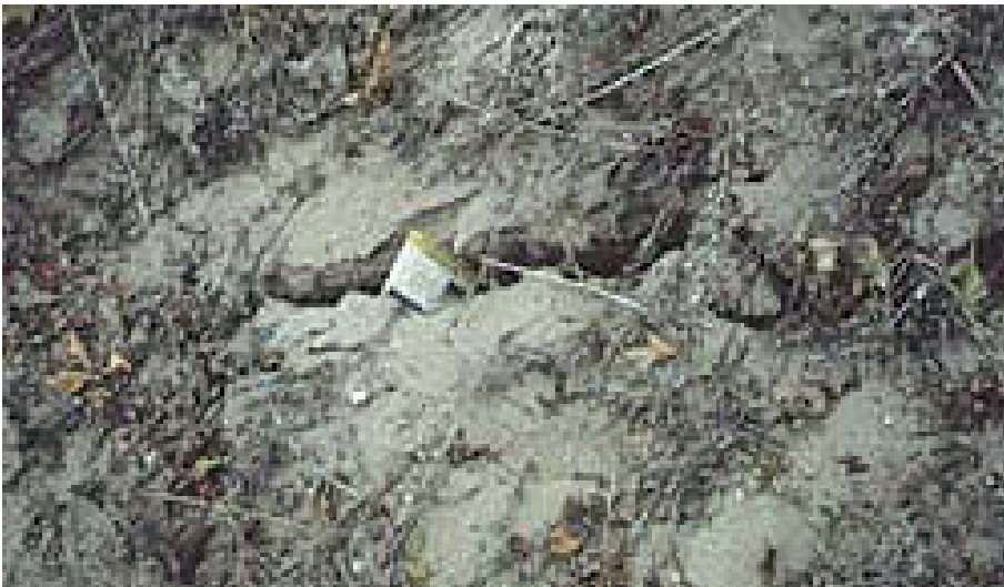
Figure 36. Ground cracks. (Photograph courtesy of Utah Geological Survey.)
