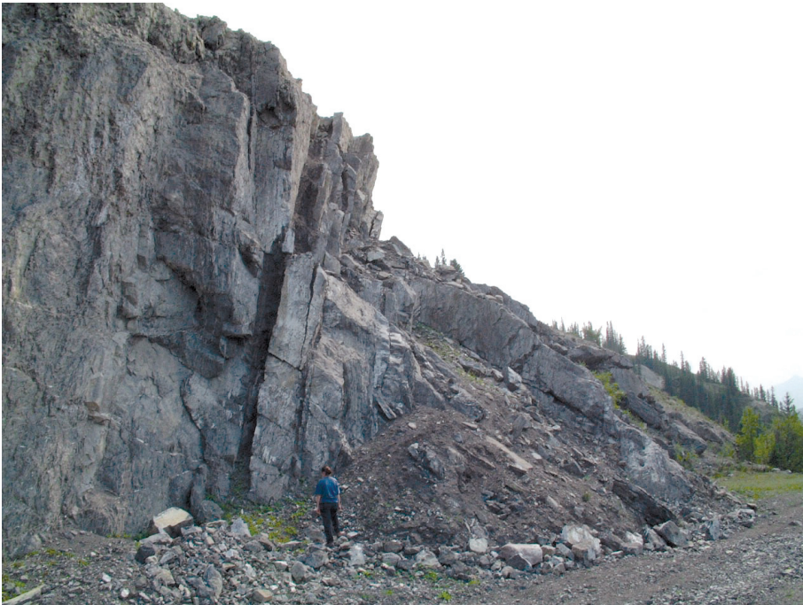
Figure 6. Photograph of block toppling at Fort St. John, British Columbia, Canada. (Photograph by G. Bianchi Fasani.)
