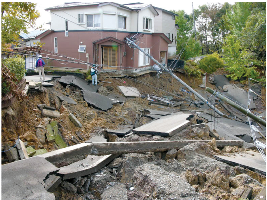
Figure 27. Earthquake-induced landslide damage to a house built on artificial fill, after the 2004 Niigata Prefecture earthquake in Japan. (Photograph by Professor Kamai, Kyoto University, Japan.)
